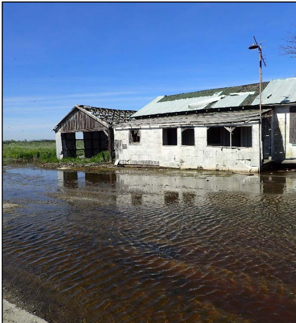
Photograph 19. View of abandoned building and site flooding; view west (Figure 2d).
