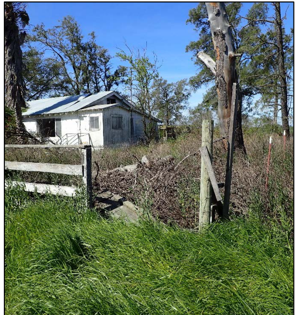
Photograph 48. Abandoned residence (Figure 2e).
