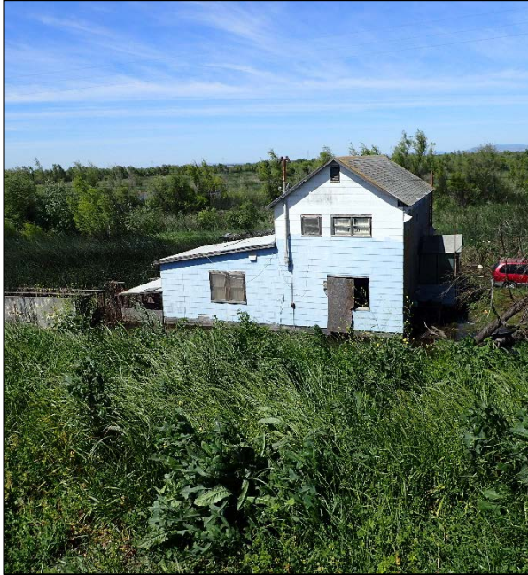
Photograph 65. Abandoned residence with vehicle. Final residence along main access road; south end of development (Figure 2e).
