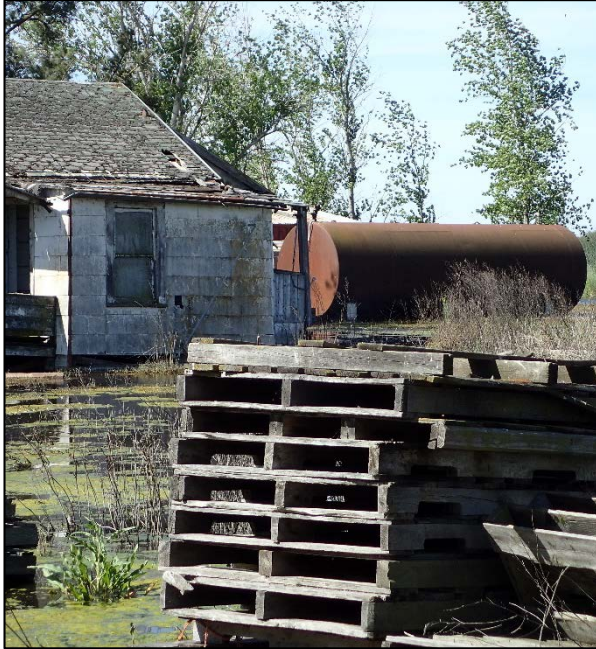
Photograph 53. Abandoned residence with wood pallets and AST (Figure 2e).
