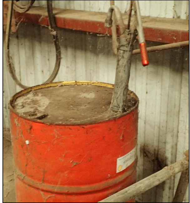
Photograph 30. Warehouse interior. Waste oil collection drum. Set over concrete foundation with no secondary containment observed (Figure 2d).
