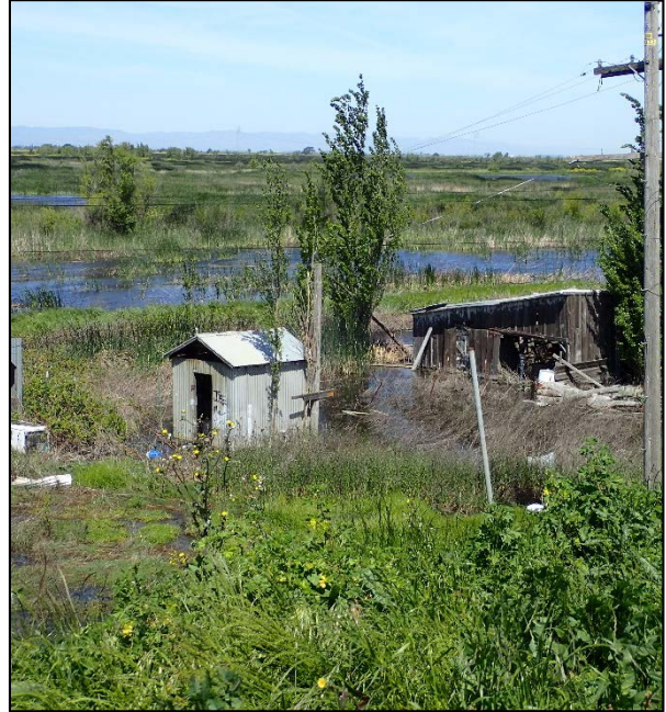
Photograph 66. Abandoned shed with LPG tank, dilapidated barn, and general debris (Figure 2e).
