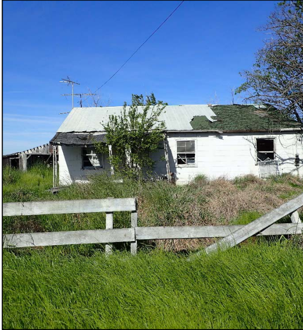
Photograph 45. Abandoned residence (Figure 2e).
