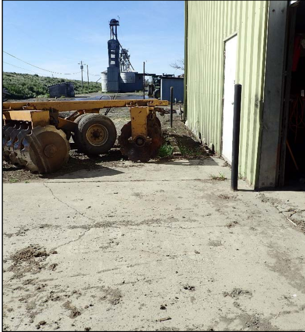
Photograph 17. View of exterior warehouse with tiller equipment, grain driers and storage; view south along the main driveway through developed portion of the Subject Property (Figure 2d).
