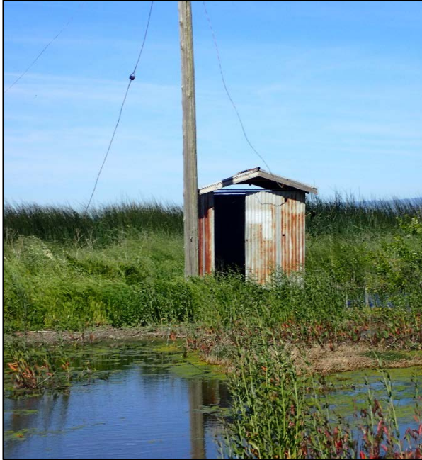
Photograph 41. Irrigation pump house (Figure 2d) .
