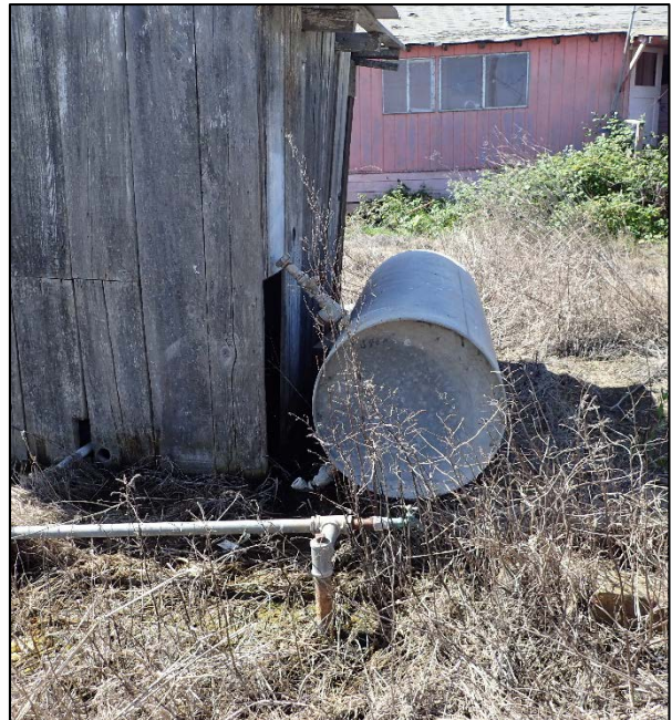
Photograph 60. Abandoned LPG tank associated with shed and abandoned residence (Figure 2e).
