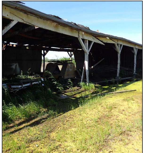
Photograph 56. Open-walled garage used for storage of farm equipment (Figure 2e).
