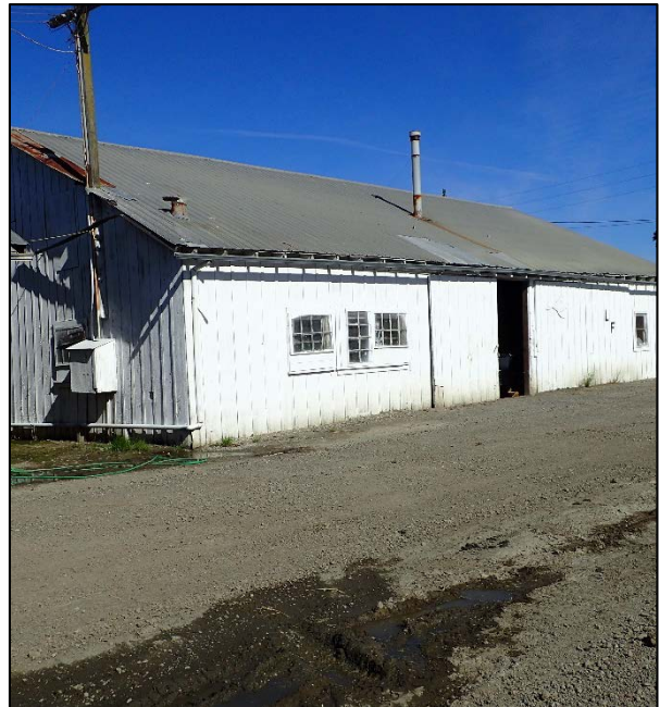
Photograph 16. Wood framed barn used for storage.
