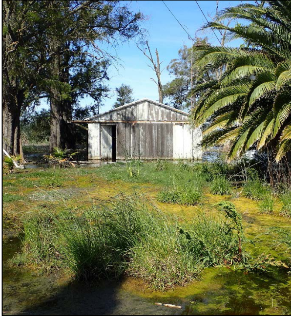
Photograph 49. Abandoned residence (Figure 2e).
