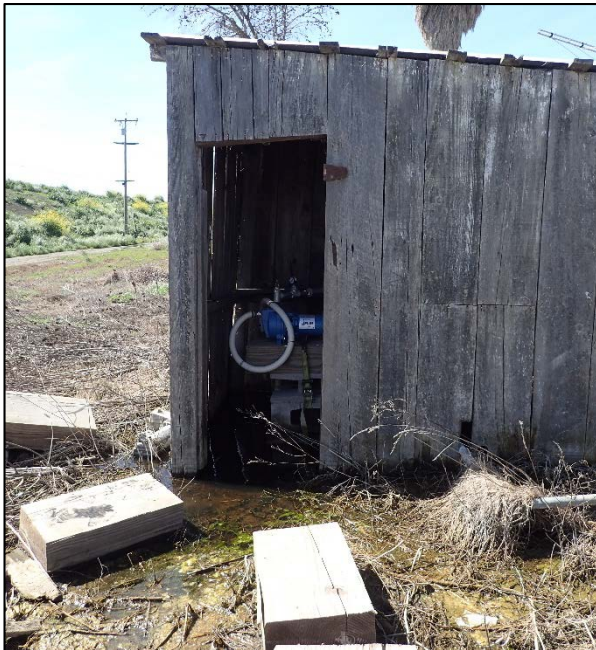
Photograph 59. Domestic well pump with casing inside storage shed (active; Figure 2e).
