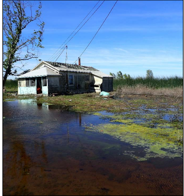
Photograph 62. Abandoned residence with LPG tank (Figure 2e).
