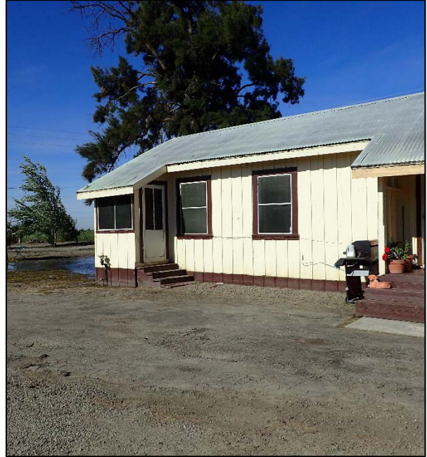
Photograph 10. View of the occupied caretaker’s residence (Figure 2d).
