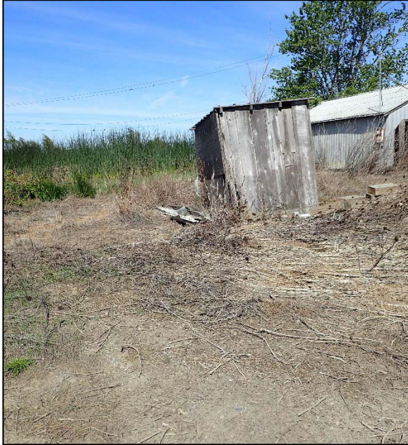
Photograph 57. Storage shed with domestic well pump near abandoned residence (Figure 2e).
