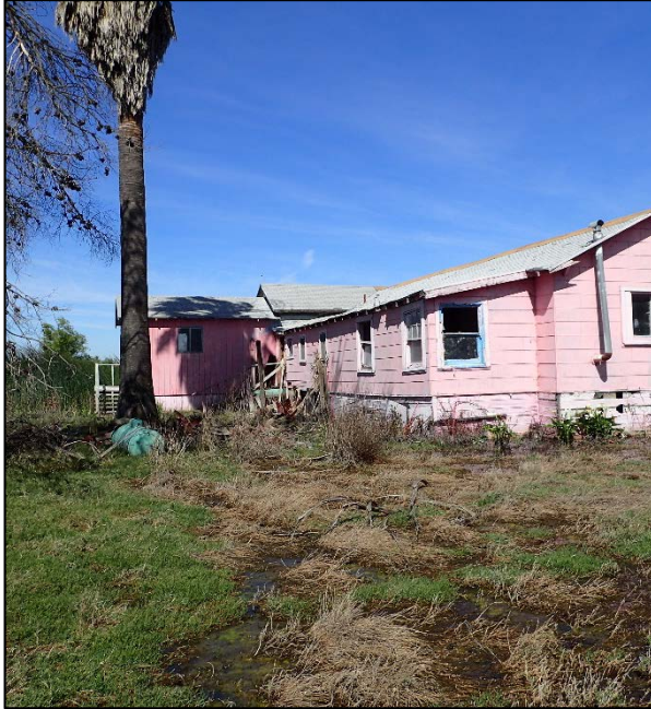
Photograph 61. Abandoned residence with LPG tank (Figure 2e).
