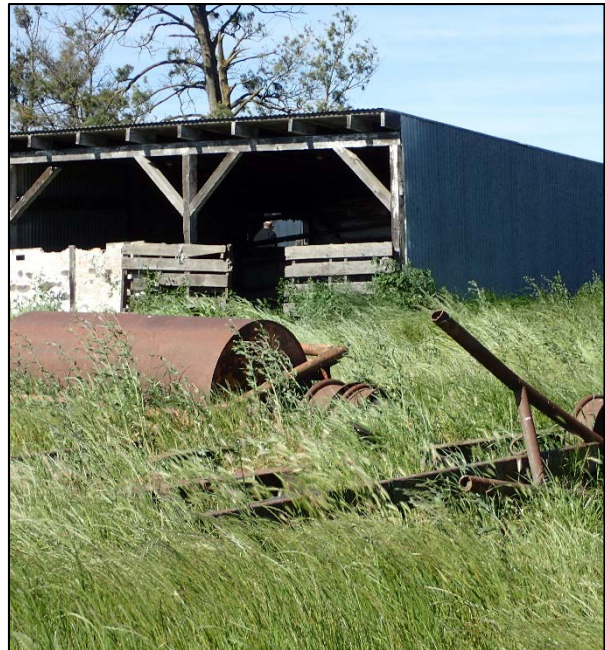
Photograph 36. Dilapidated barn with ferrous metal scrap in foreground. Scrap includes abandoned ASTs (Figure 2d).
