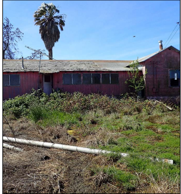
Photograph 58. Abandoned residence adjacent to shed (Figure 2e).
