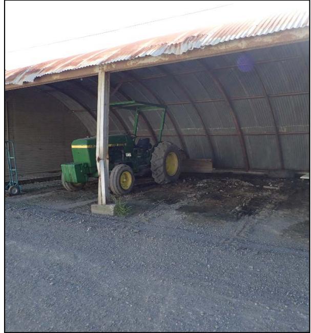
Photograph 14. View of the interior garage adjacent the fuel ASTs. Staining is visible on the ground surface (Figure 2d).
