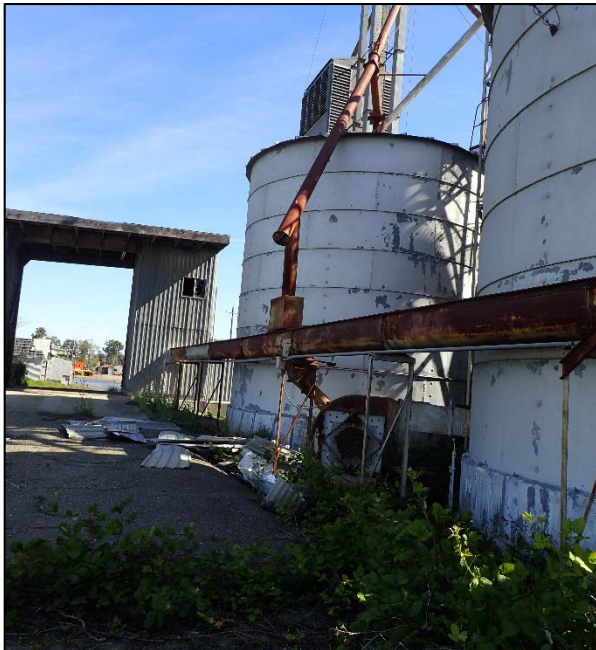
Photograph 39. View of grain driers, storage, and infrastructure (Figure 2d).
