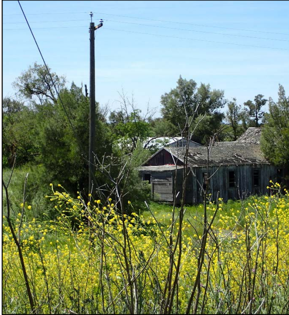
Photograph 1. Abandoned settlement in the northern section of the Subject Property. View of the abandoned barn, post office, and dwellings (Figure 2a).
