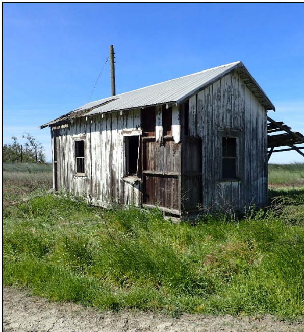
Photograph 35. Dilapidated shed; abandoned (Figure 2d).
