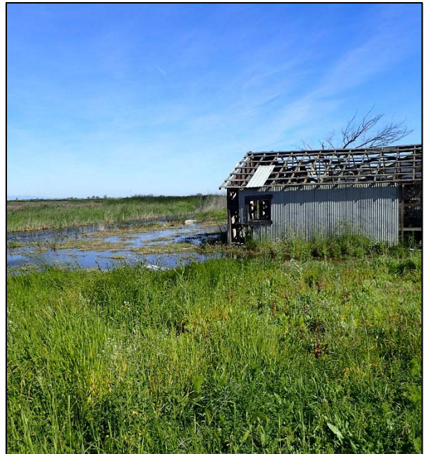
Photograph 20. View of abandoned shed and site flooding; view northwest (Figure 2d).
