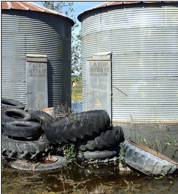
Photograph 51. Abandoned storage silos with used tires (Figure 2e).
