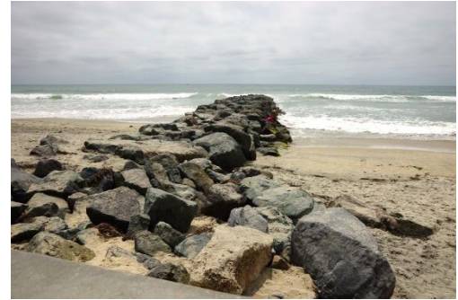
In the 1950s, groins were constructed in Imperial Beach in an effort to combat erosion.
