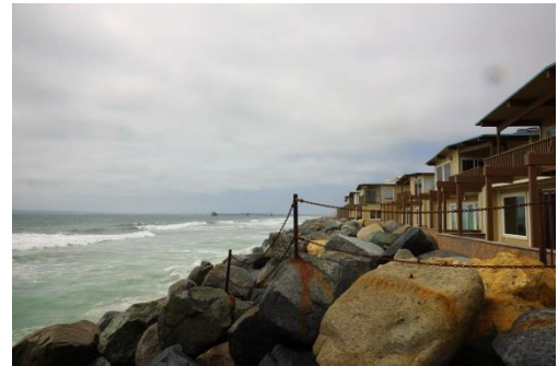
Past storms have resulted in adaptive responses such as the construction of hard armoring protection devices.
