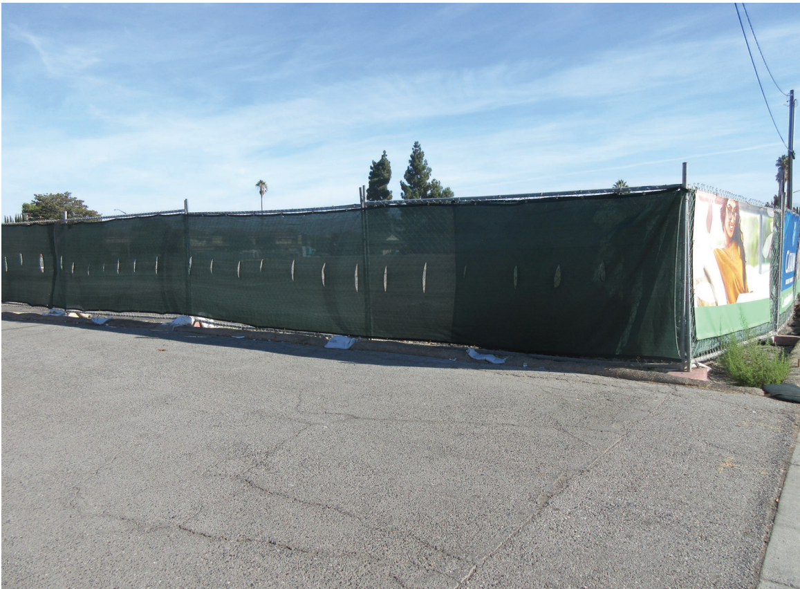
Photo 6 - View of the adjacent vacant site under construction looking northeast from the project site.
