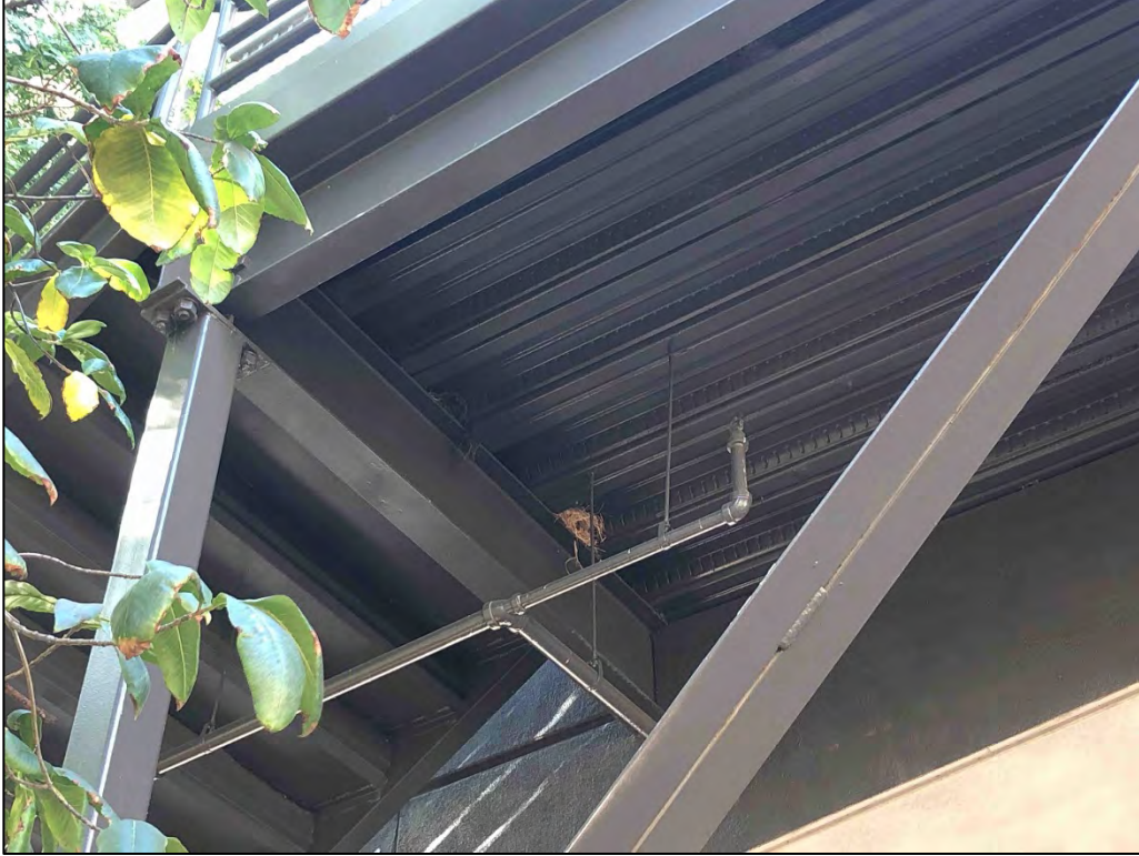
Photo 5. Birds Nest Under Stairway Along Olive Street
