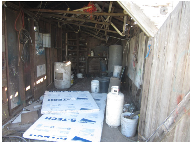
Photo 5: View of the interior of the garage.
