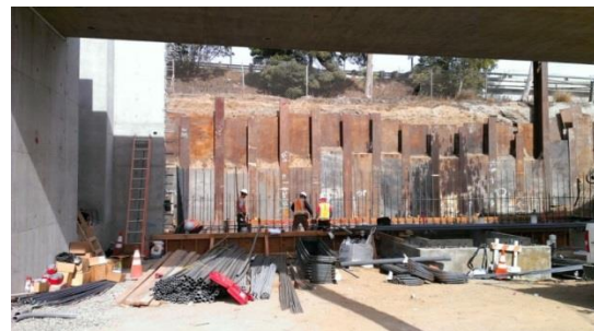
A soldier pile wall supports adjacent land during construction.
