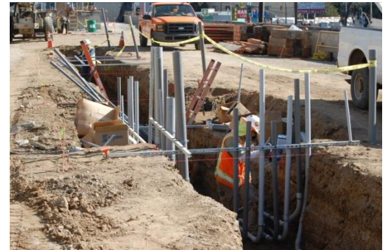
Coordination of underground utilities is critical.
