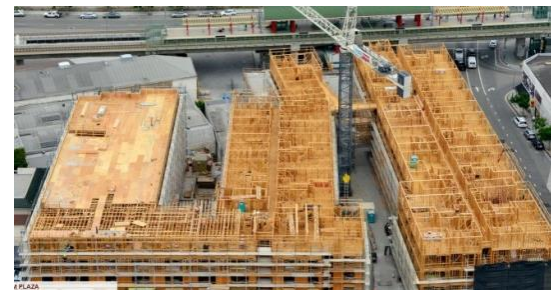
Construction adjacent to the Chinatown Rail Station.
