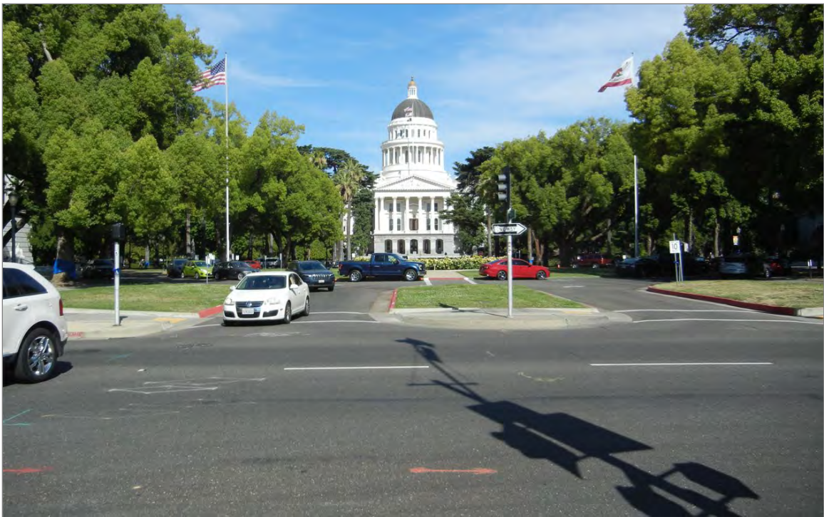
Source: Photograph taken by Ascent Environmental in 2019.
