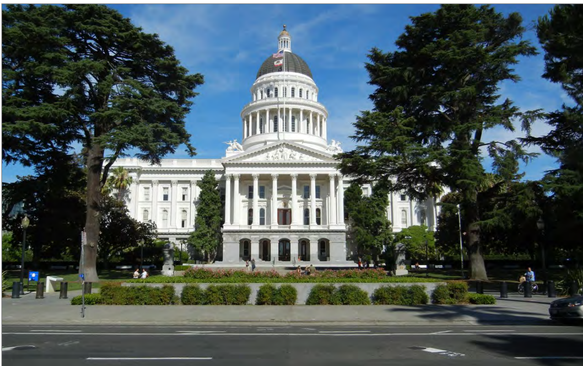
Source: Photograph taken by Ascent Environmental in 2019.
