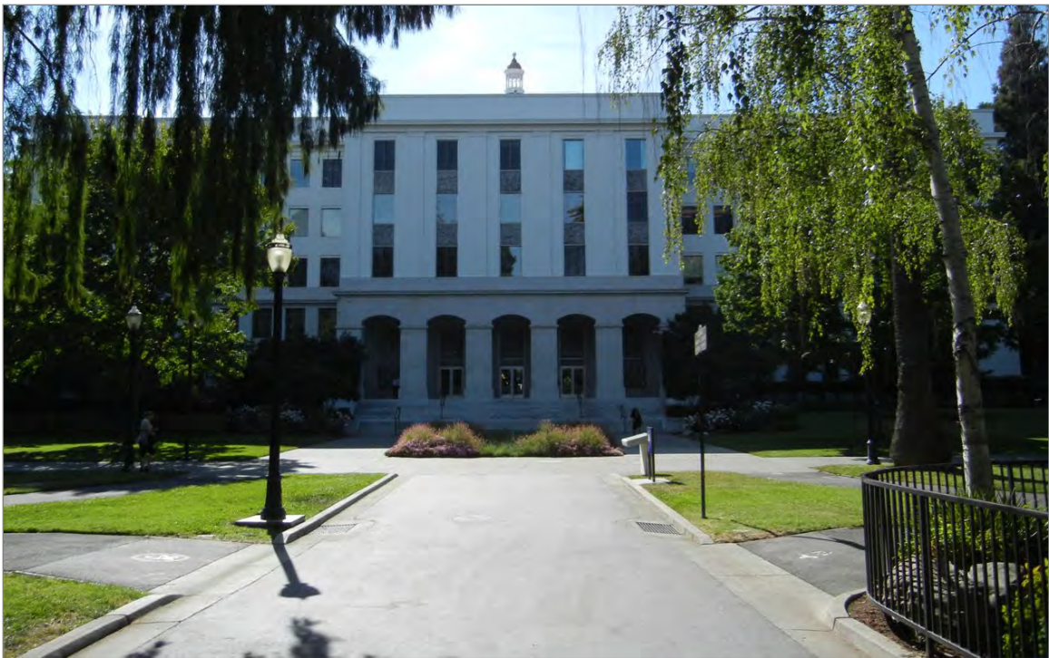
Source: Photograph taken by Ascent Environmental in 2019.
