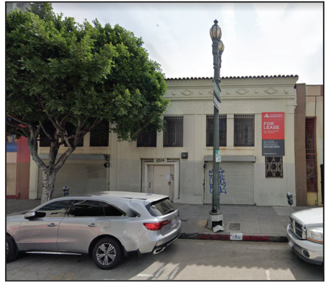
View 5: View looking southeast at commercial industrial building at 1224 South Hope Street.
