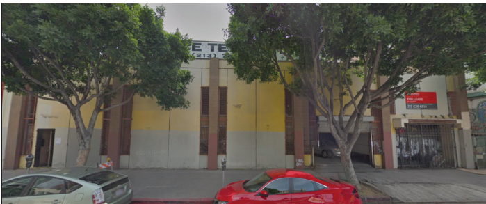
View 6: View looking southeast at commercial industrial building at 1240 South Hope Street.
