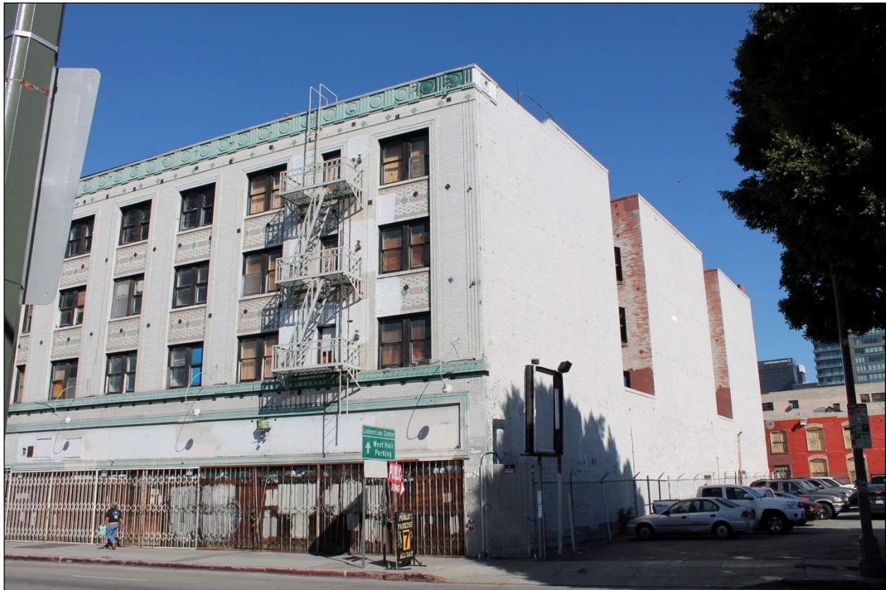
Figure 8: Western portion of Pico Blvd. elevation and east side elevation, view facing northwest, 2016 (Steinberg)
