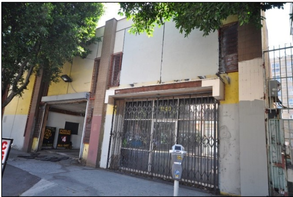
Figure 21: 1230-40 S. Hope Street, primary elevation garage bays, 2017 (GPA)
