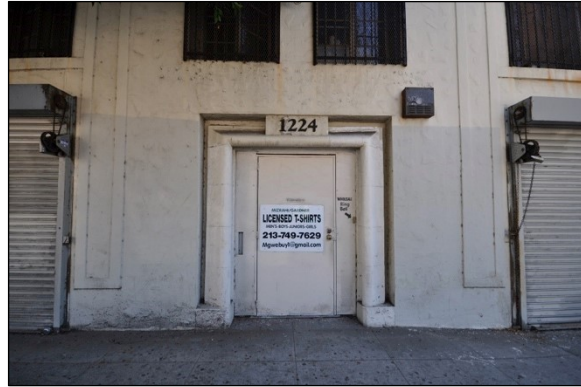
Figure 17: 1224 S. Hope Street, primary entrance, 2017 (GPA)
