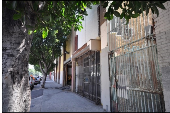
Figure 20: 1230-40 S. Hope Street, southernmost bay on primary elevation, 2017 (GPA)
