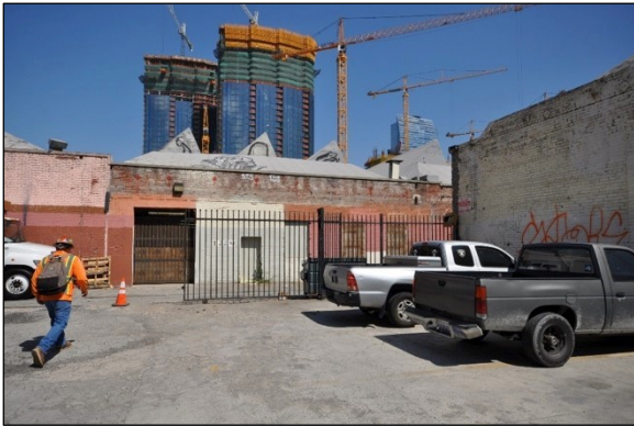
Figure 18: 1224 S. Hope Street, rear elevation, 2017 (GPA)
