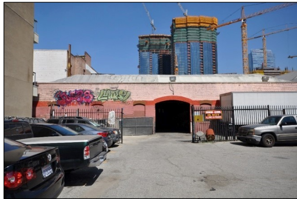
Figure 22: 1230-40 S. Hope Street, rear elevation, 2017 (GPA)
