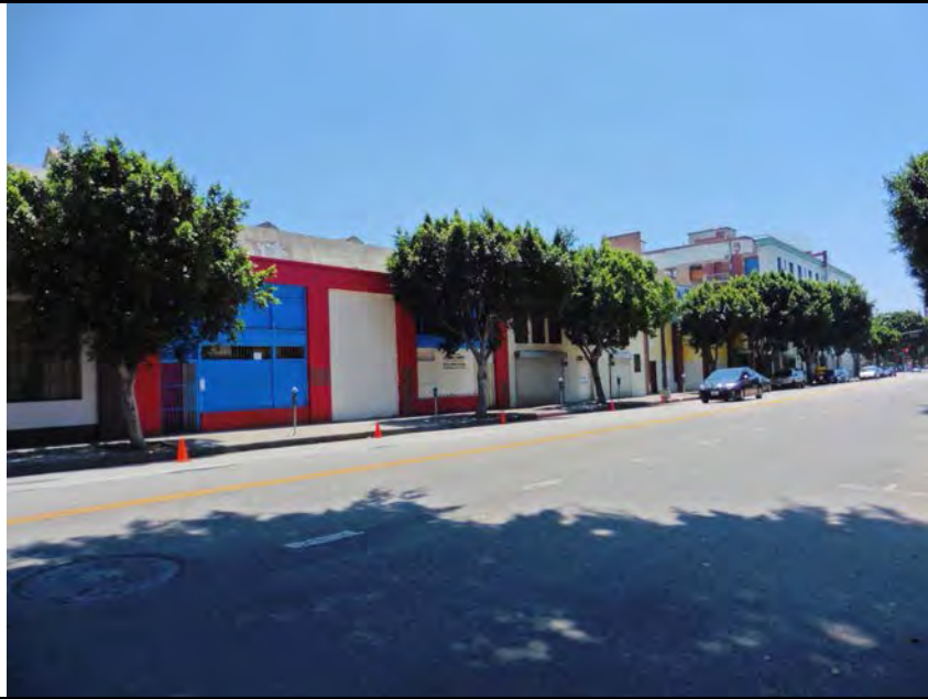
1. Site: View of the Site (industrial warehouse buildings and commercial hotel building), looking south across South Hope Street.
