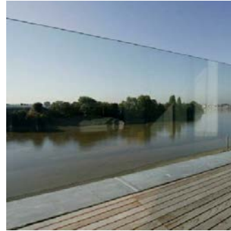
GLAZING #3: TEMPERED GLASS GUARDRAIL, LOW REFLECTIVE
