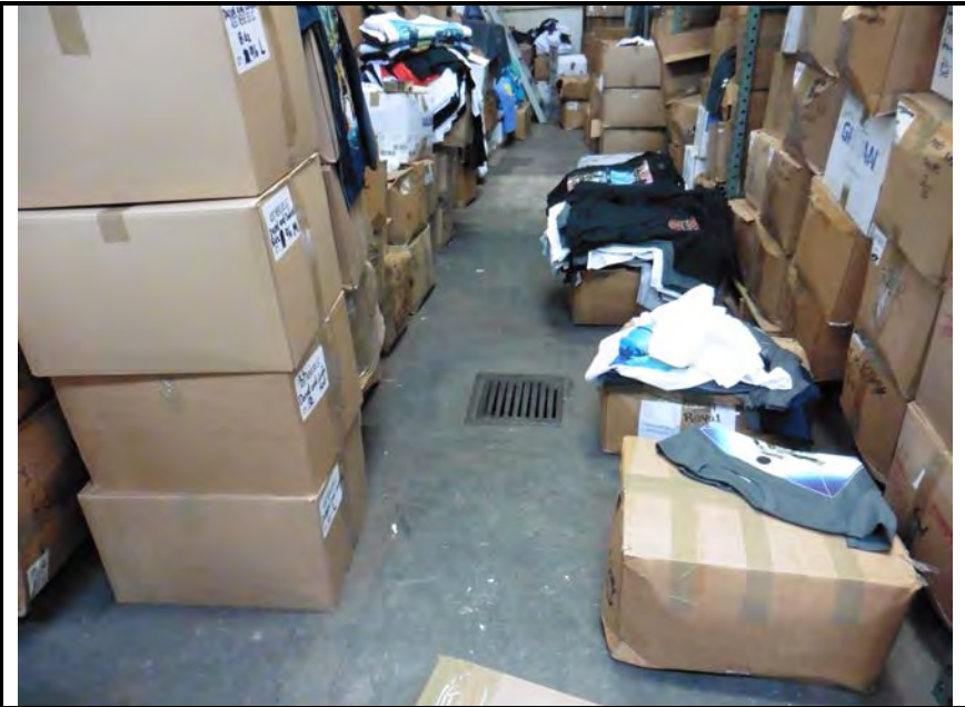
6. Site Interior: View of a small floor drain located in 1220 South Hope Street.
