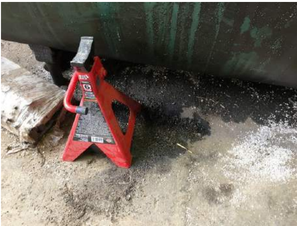
27. View of staining located near the new oil ASTs in the maintenance shop of the subject property.
