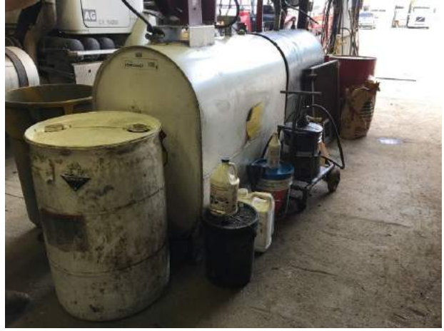
26. View of the 55-gallon drum of heavy emulsifying cleaner, 275-gallon new oil AST and 275-gallon hydraulic oil AST located in the maintenance shop.
