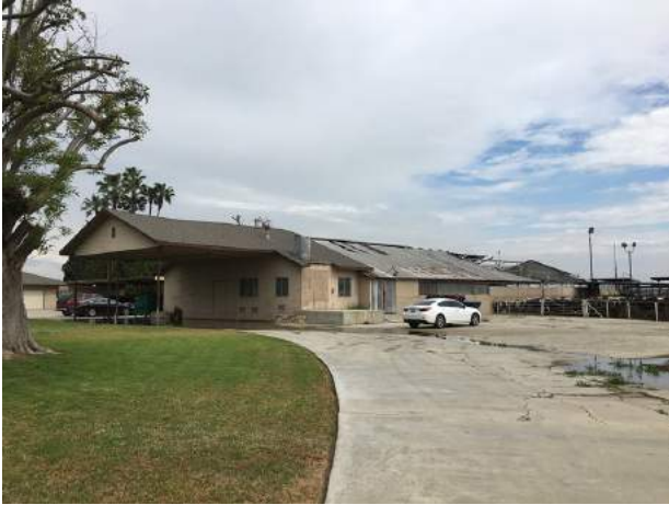
43. View of an abandoned milk barn located to the south of the office building of the subject property.
