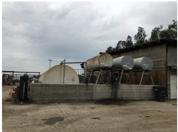
30. View of the 10,000-gallon and three 1,000-gallon diesel ASTs for fueling located to the south of the scale building located on the northern central portion of the subject property.
