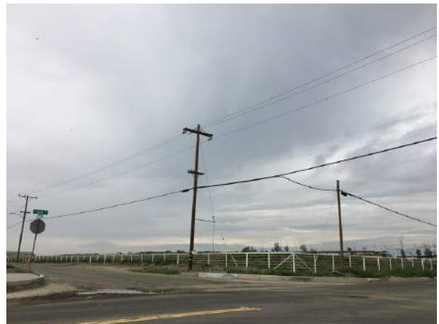
54. View of the northwestern adjacent property from across the intersection of South Grove Avenue and Eucalyptus Avenue.
