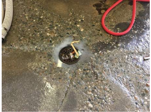
14. View of a typical drain located in the calf milk barn of the subject property.
