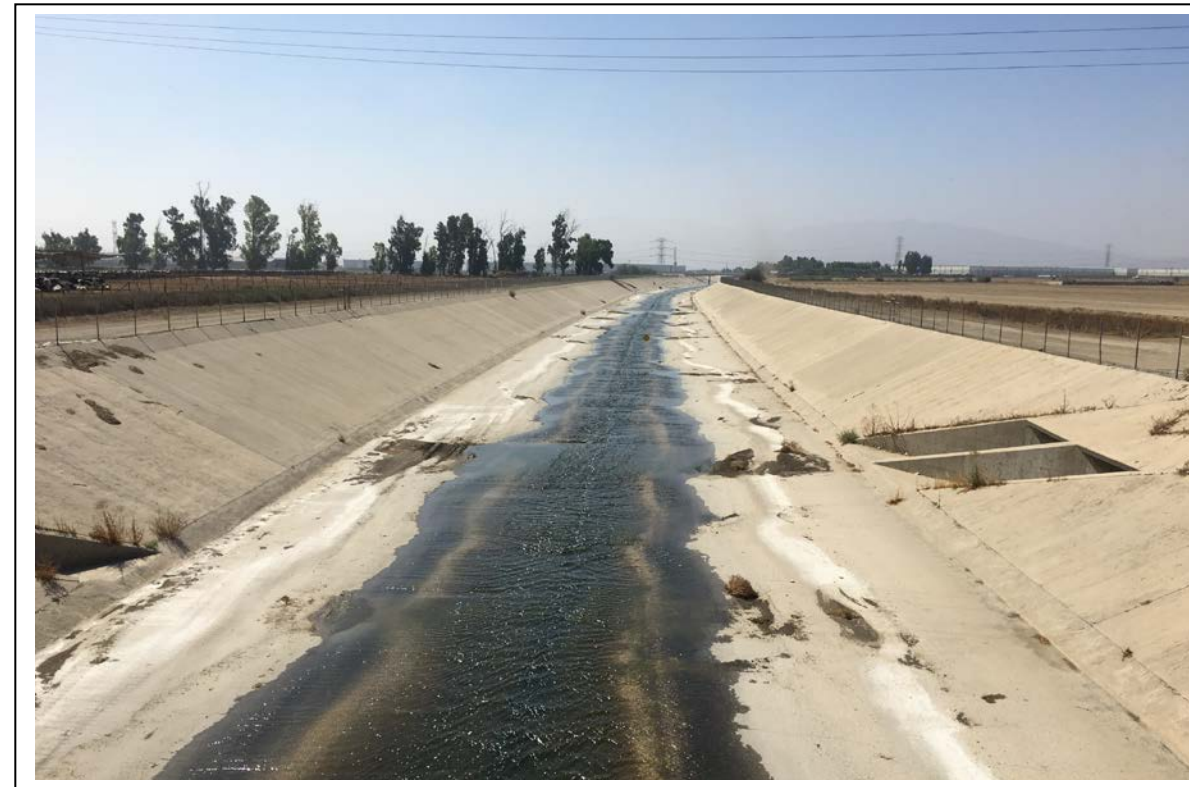
Photograph 8: View to the south of the Cucamonga Channel from the existing Merrill Avenue Bridge crossing.
