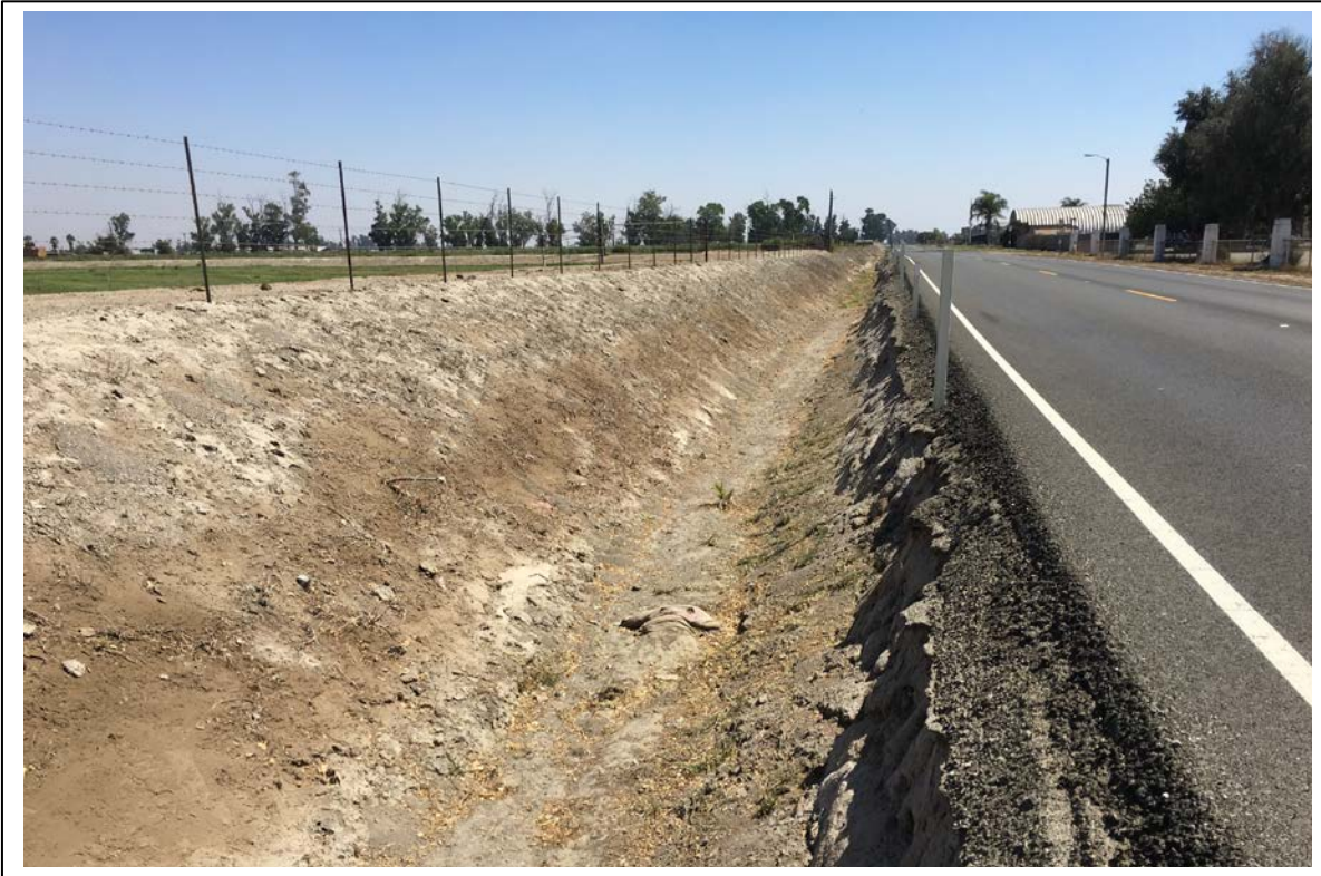
Photograph 11: View to the east of Ephemeral Drainage 1, located along the northern shoulder of Merrill Avenue.
