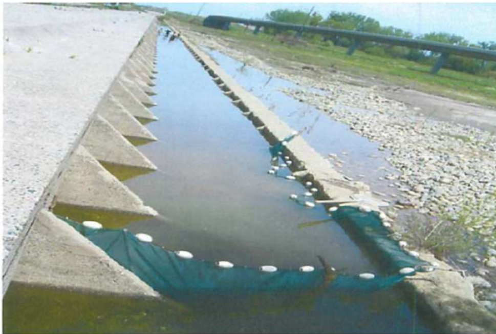
Figure 1 Photo C1-28 in DWR (2014) of the energy dissipation basin below Tisdale Weir.
