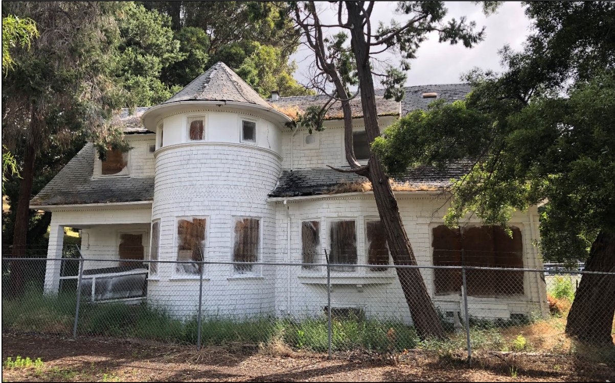
Photograph 3. West façade of Whitecotton Cottage , looking east
