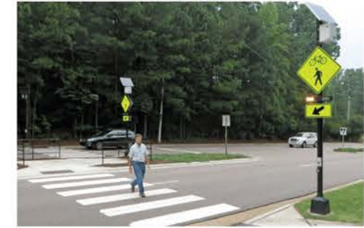
Rectangular Rapid Flashing Beacon (RRFB)
