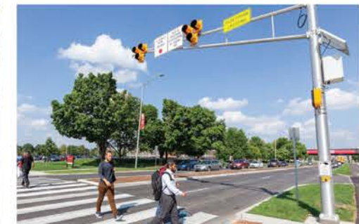
High-Intensity Activated crossWalk Beacon (HAWK)
