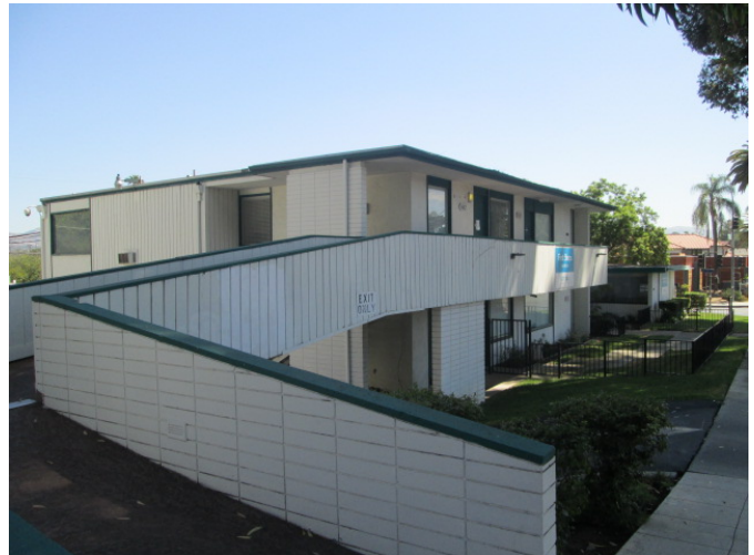
10. View of the eastern adjacent property looking east.
