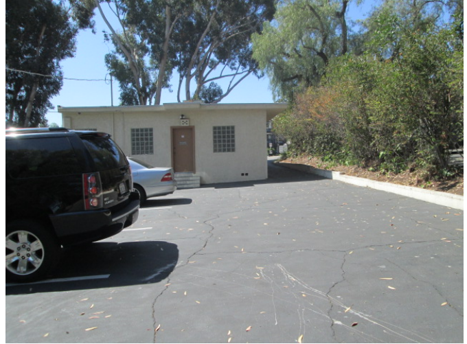
8. View of the parking area at the Site looking south.
