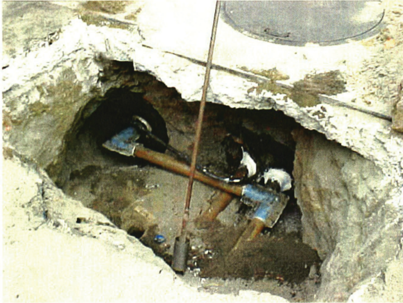
Sample at repair of piping at 3000 gallon tank
