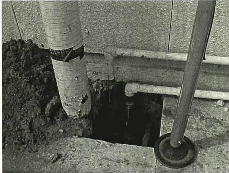
REPAIR TO SECONDARY PIPE AT UNDERGROUND/ABOVEGROUND TRANSITION
