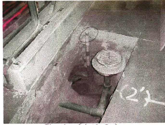
Floor drain (to clarifier) Waste oil fill pipe is circled (sampled at elbow base)
