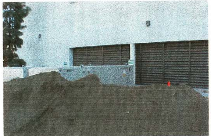
Stockpile, looking S. toward hospital
