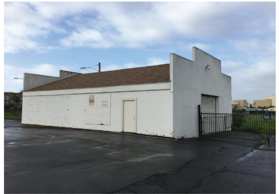
1009 North Coast Highway
