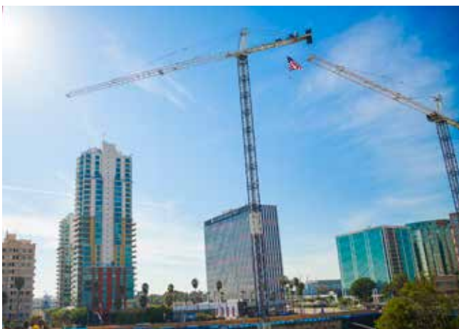
Construction of city hall
