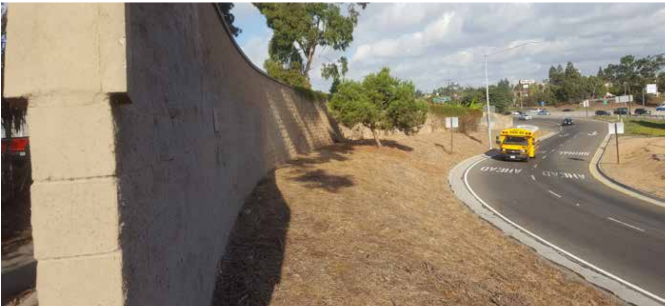
Sound wall to protect residential neighborhood from noise
