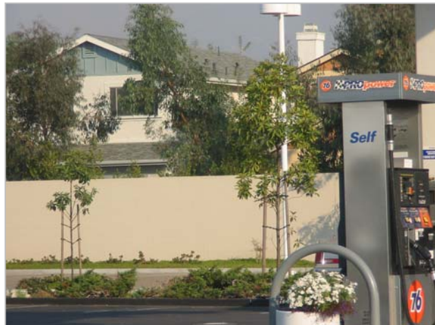
Sound Wall Separating Residential and Commercial Developments
