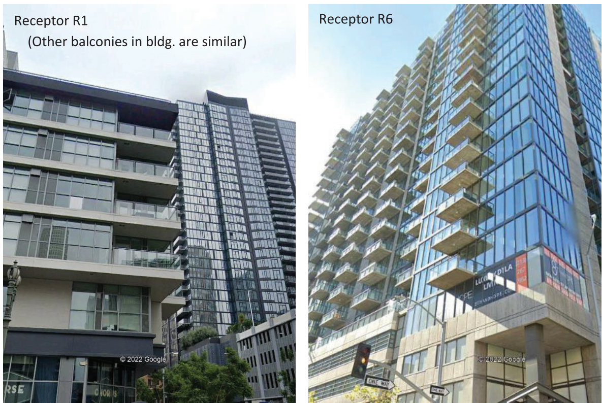
FIGURE 1 BALCONIES AT RESIDENTIAL RECEPTORS R1 AND R6
