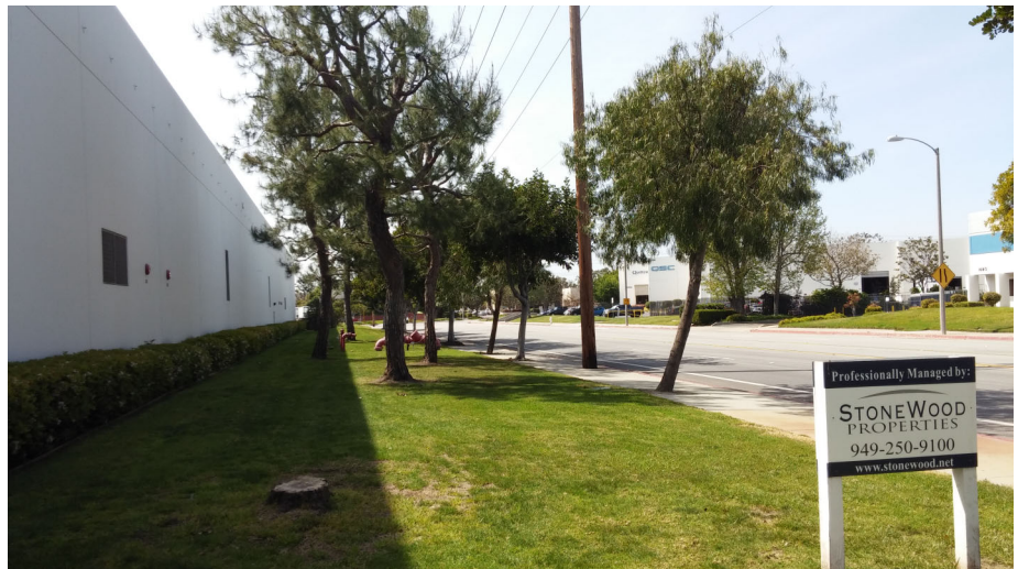
Photo 4 View looking west along northern border of site, Sunflower Ave. Except for the strip of turf grass and ornamental trees, this section is completely paved.
