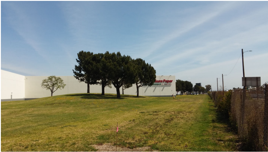
Photo1. View looking southeast along southern border of property, bordered by the 405 freeway.
