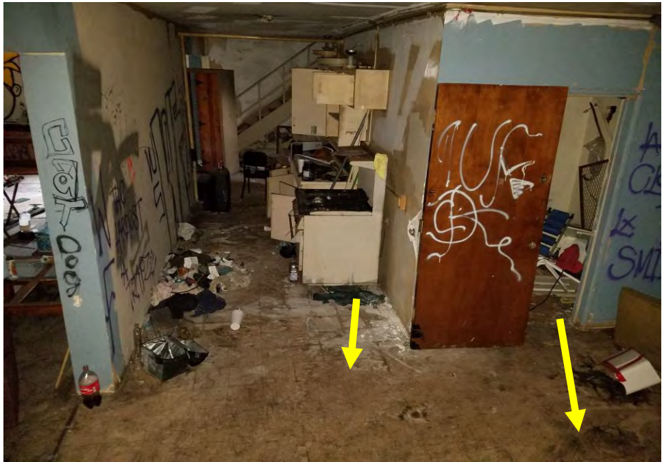
Photograph 6: Building 1: view of asbestos-containing 9'x9' vinyl floor tile.
