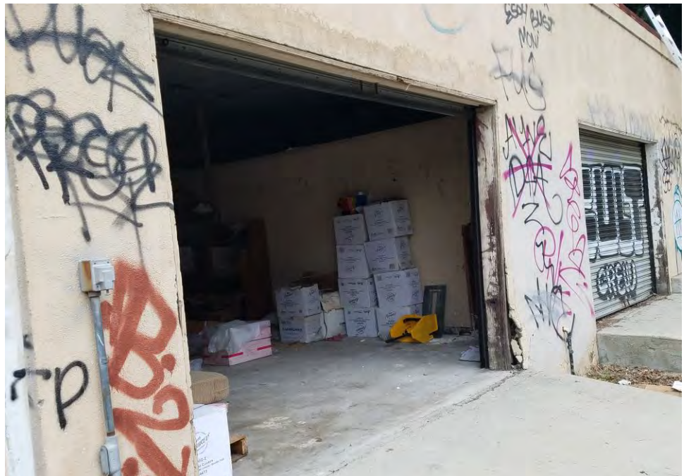
Photograph 10: General view of Building 2.
