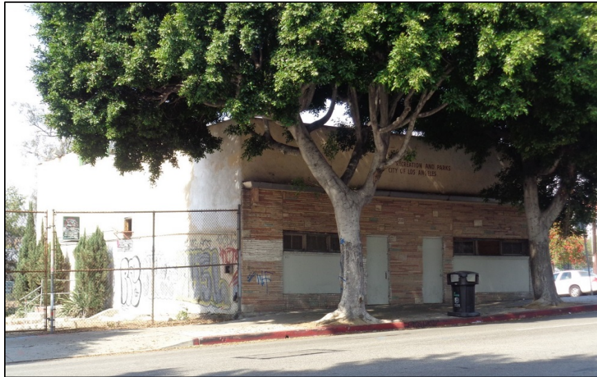
Figure 4: Primary and east elevation, camera facing south. ICF, 2018.
