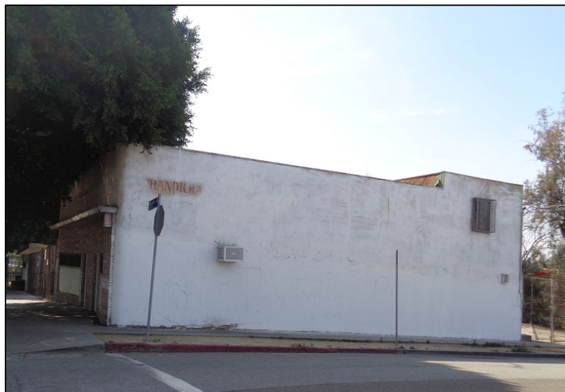
Figure 5: West elevation, camera facing southeast. ICF, 2018.
