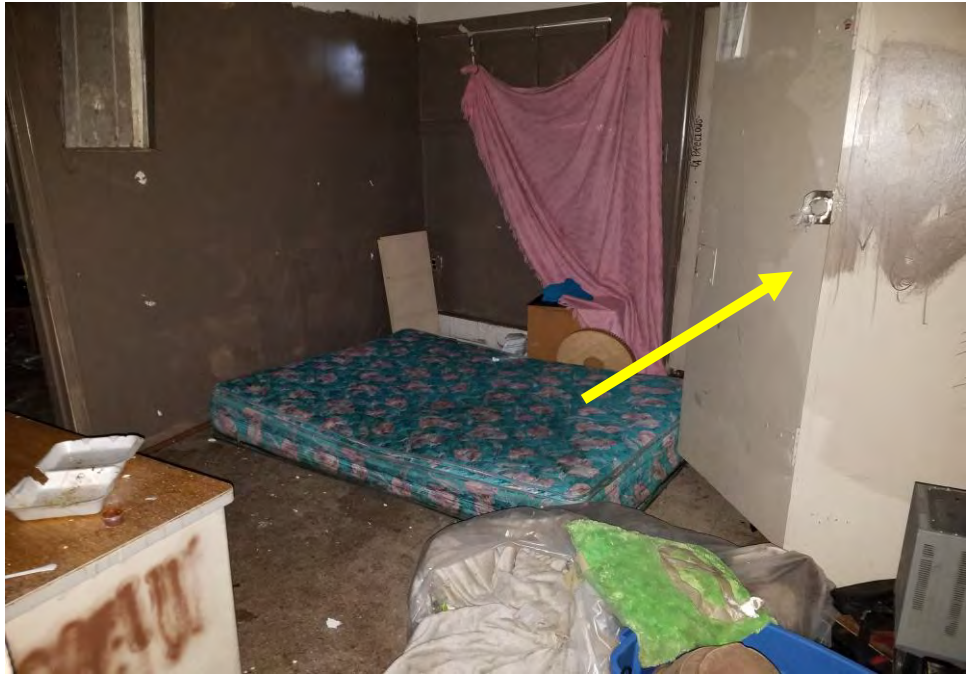
Photograph 9: Building 1: view of lead containing door.
