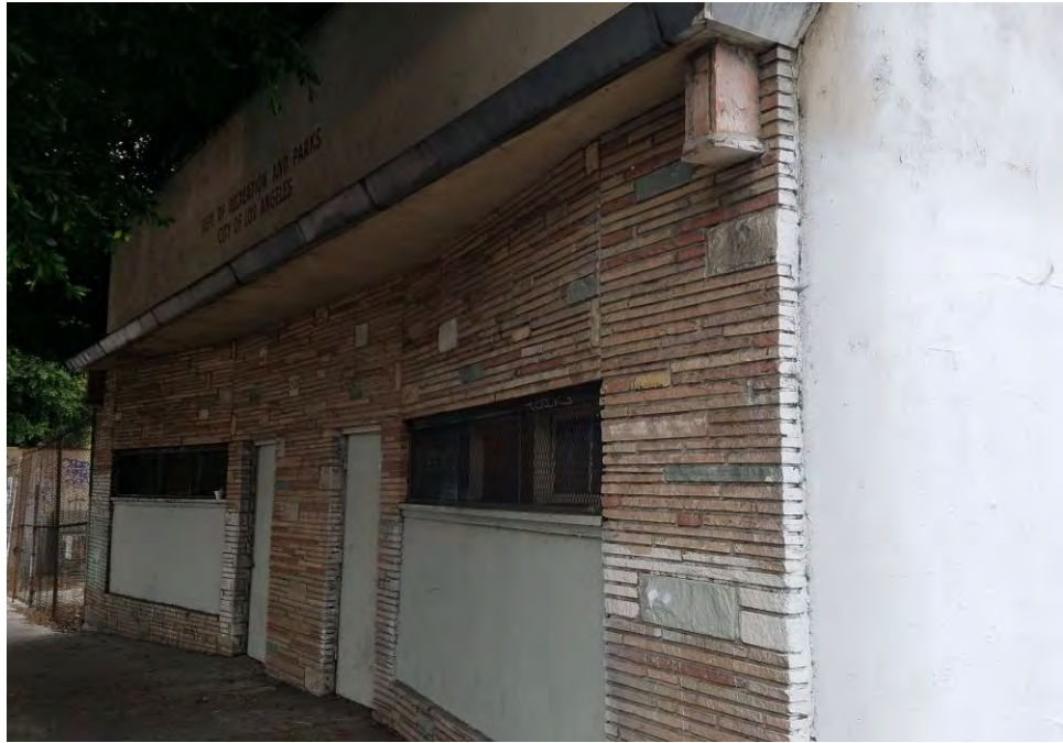
Photograph 1: General front view of Building 1.
