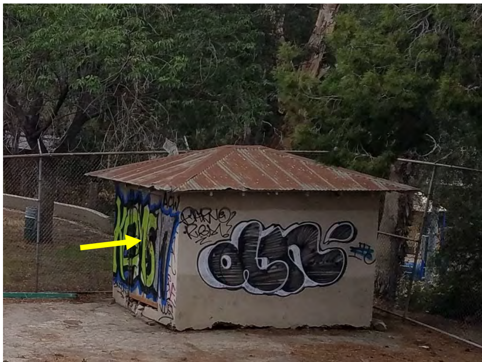
Photograph 14: Shed 1: view of lead-containing main door.
