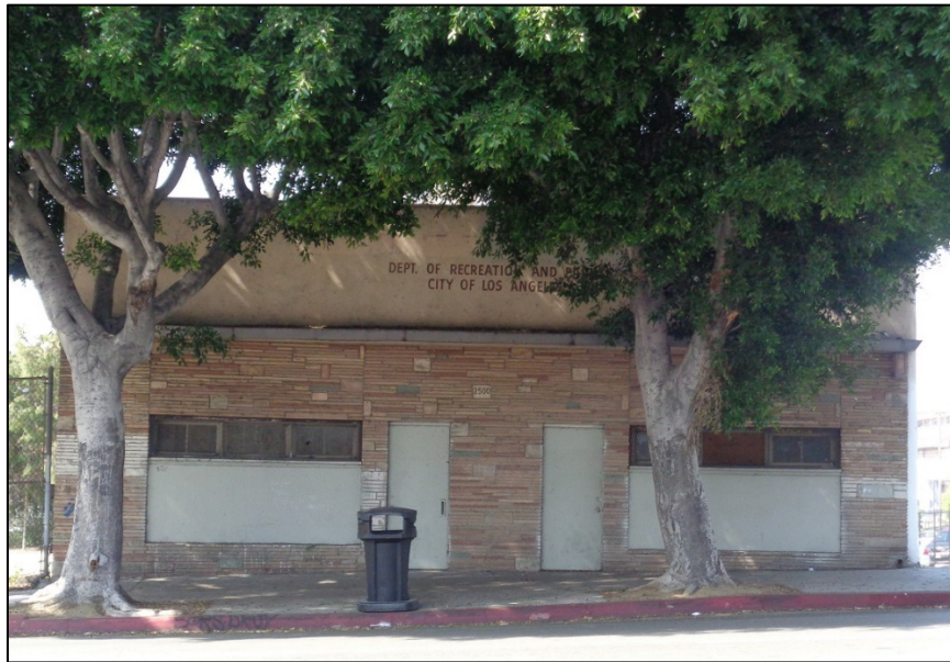
Figure 1: Primary elevation, detail, camera facing southwest. ICF, 2018.
