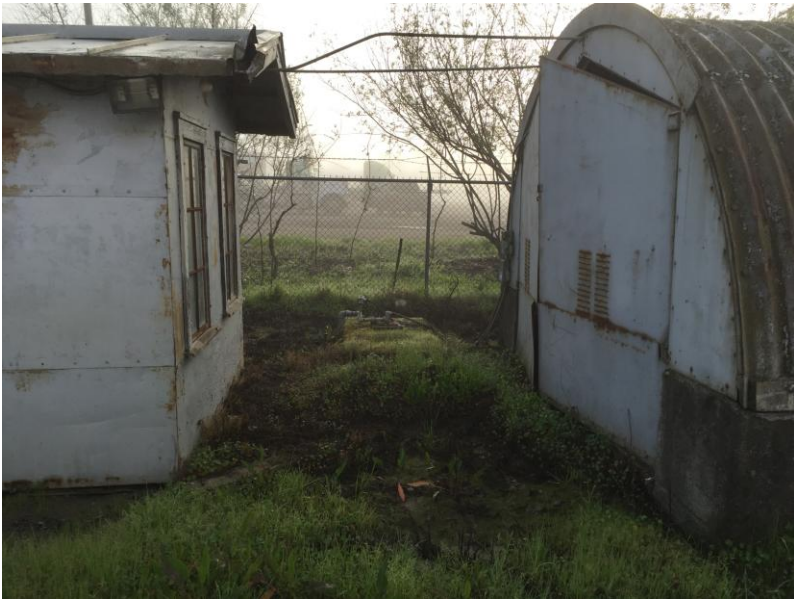
Photo 5: View showing domestic well casing at 325 Yolanda Avenue
