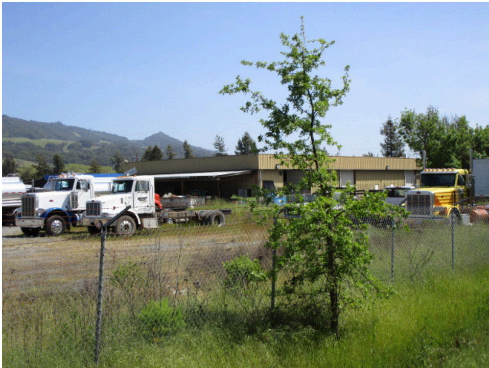
46. Warehouse (455 Yolanda Avenue) adjacent to the east
