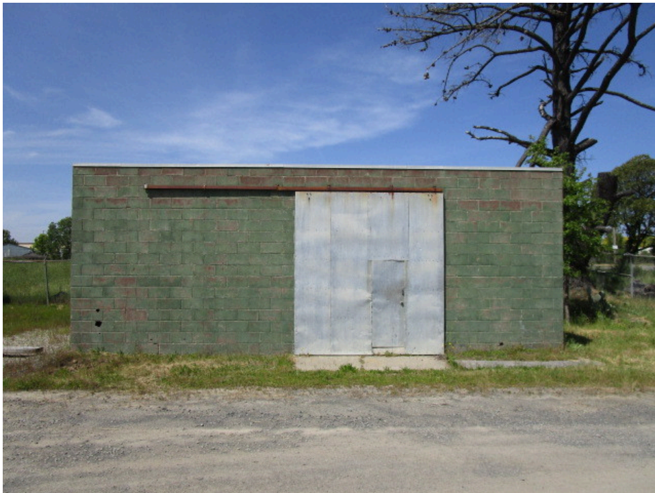
8. Concrete block building adjacent to the northwest of the gate
