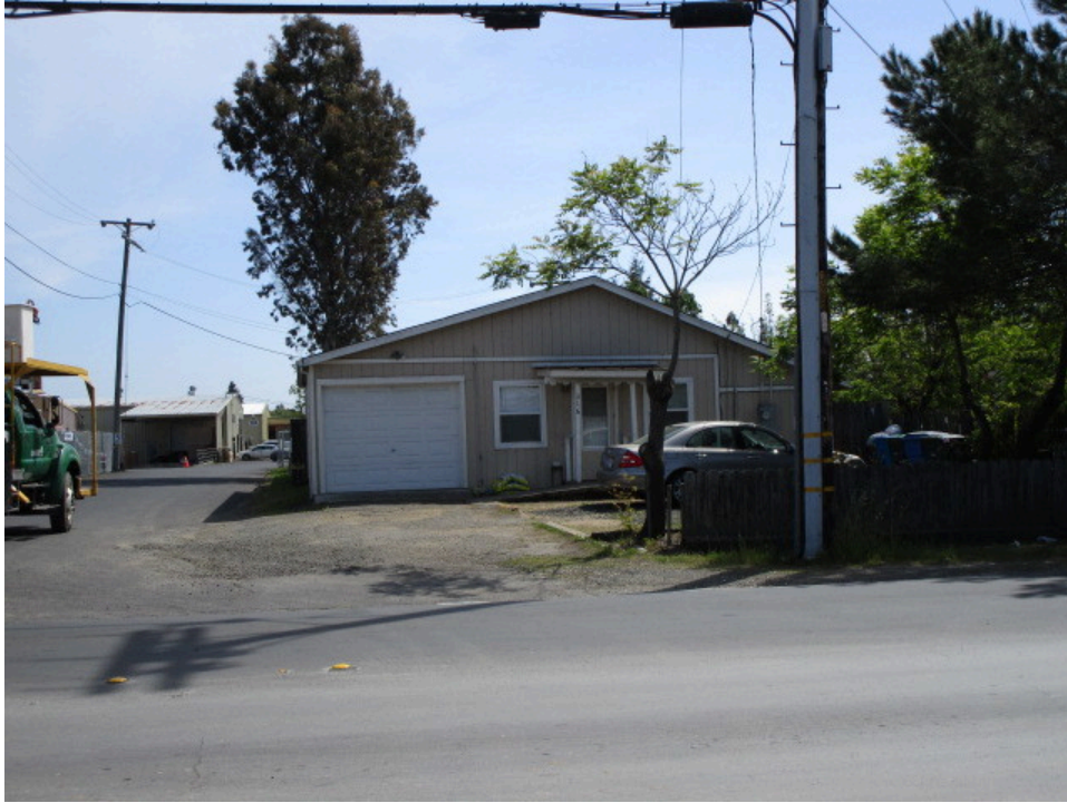
53. Residence adjacent to the south
