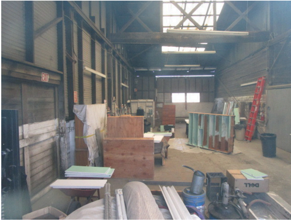
29. Interior of the former Hulsman Transportation building
