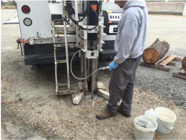
Photo 1: View of TEG advancing soil probe with 1-inch direct push rod, testing soil pressure, granular BenSeal and sand on right
