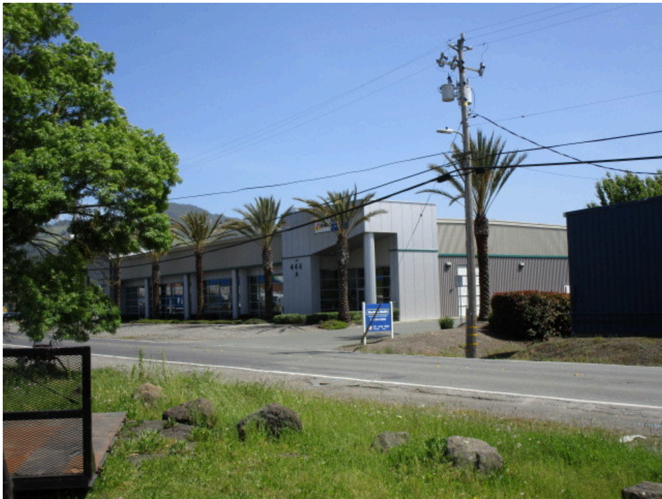
48. Flyers (444 Yolanda Avenue) adjacent to the south
