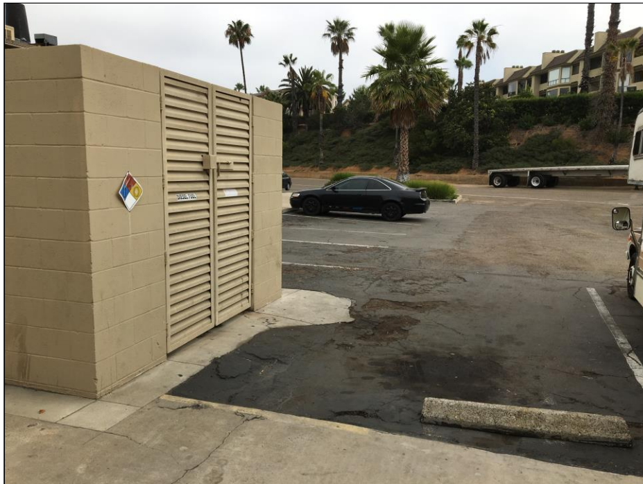
Photograph No. 28 View to the east of the entrance to the emergency generator storage area on the eastern side of the Site. De minimis staining was observed in the parking lot.
