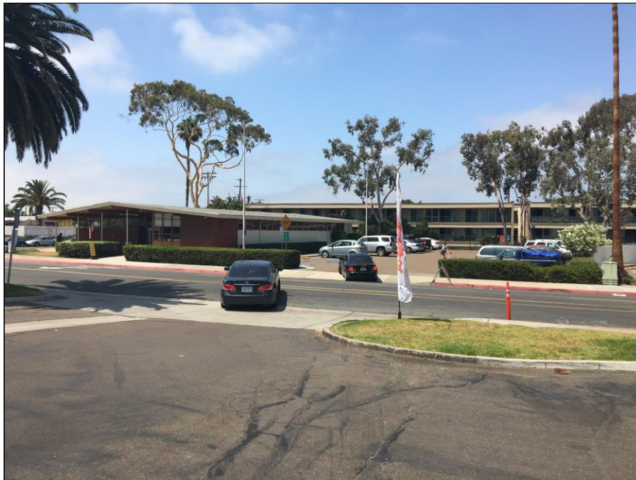
Photograph No. 38 View to the southwest of the Clairemont Branch Library across Burgener Boulevard.
