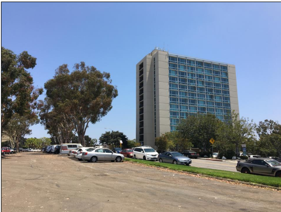
Photograph No. 36 View to the northeast of the eastern adjacent residential buildings from the eastern parking lot.
