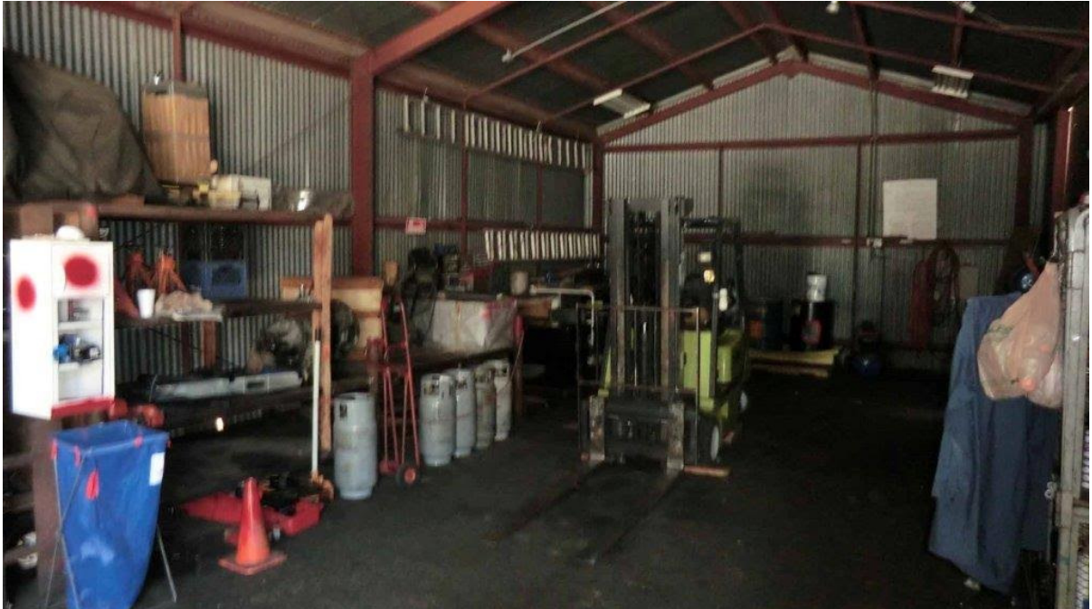
Facing east inside maintenance building. Typical automotive maintenance products were observed. The concrete floor here had petroleum product staining but no significant cracking. At rear are drums holding waste oil.
