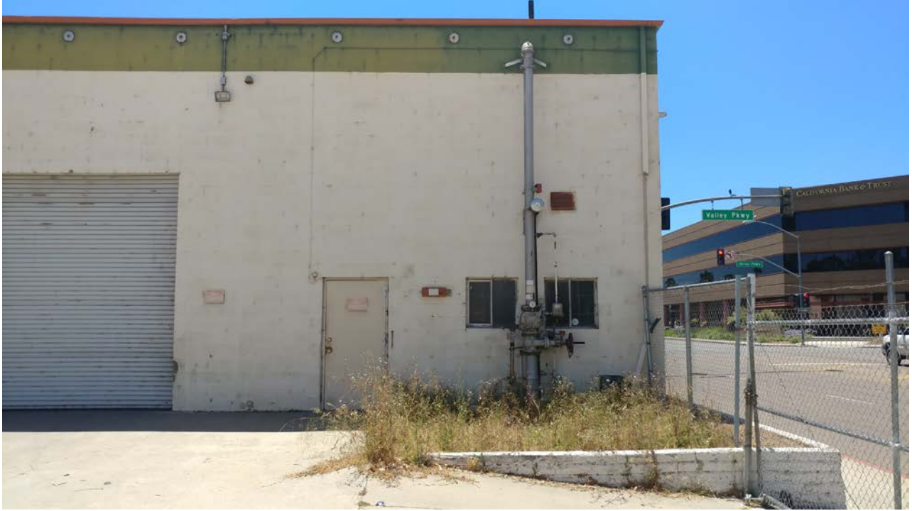
Overview of northwestern façade (utility area) of Warehouse C, looking southeast; N. Quince St. at right, driveway ramp and brick-walled planter shown in foreground.
