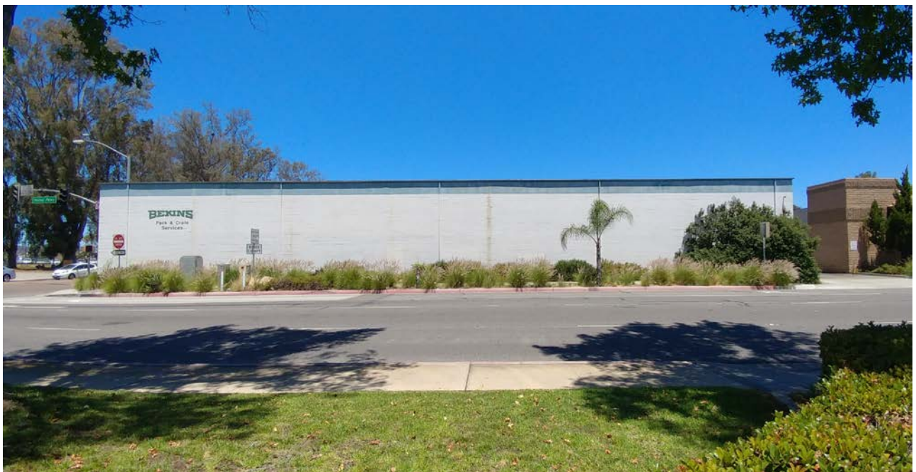
Overview of southern façade of Warehouse C, looking northwest; W. Valley Parkway in foreground, alleyway at right, and N. Quince St. shown at left.
