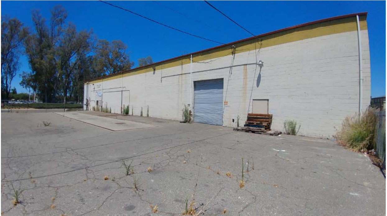
Overview of southern façade of Warehouse A, looking west from the eastern property boundary.
