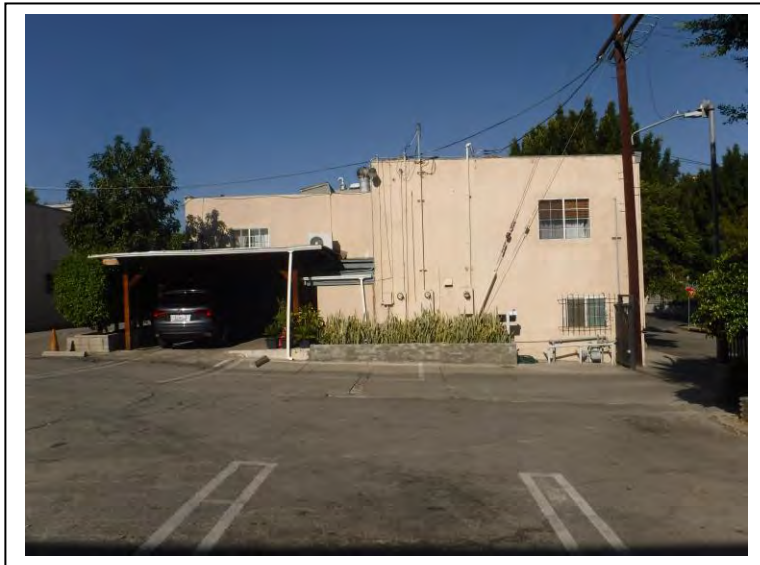
Picture (4). View of Pastor's Office/Residence, northeast portion of Site
