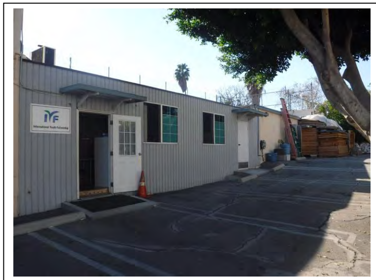
Picture (6). Storage Building at southwest corner of Site
