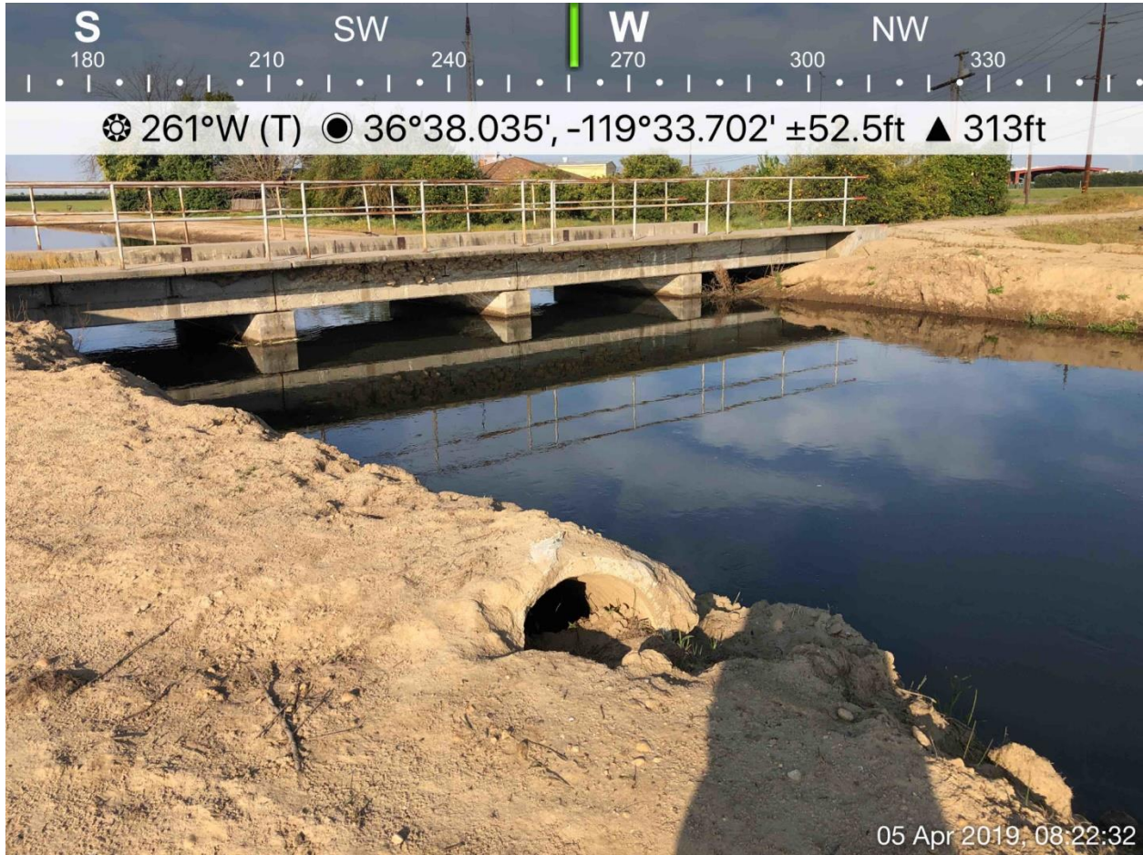
Photograph 3: Active swallow nests on structure over Mill Ditch.
