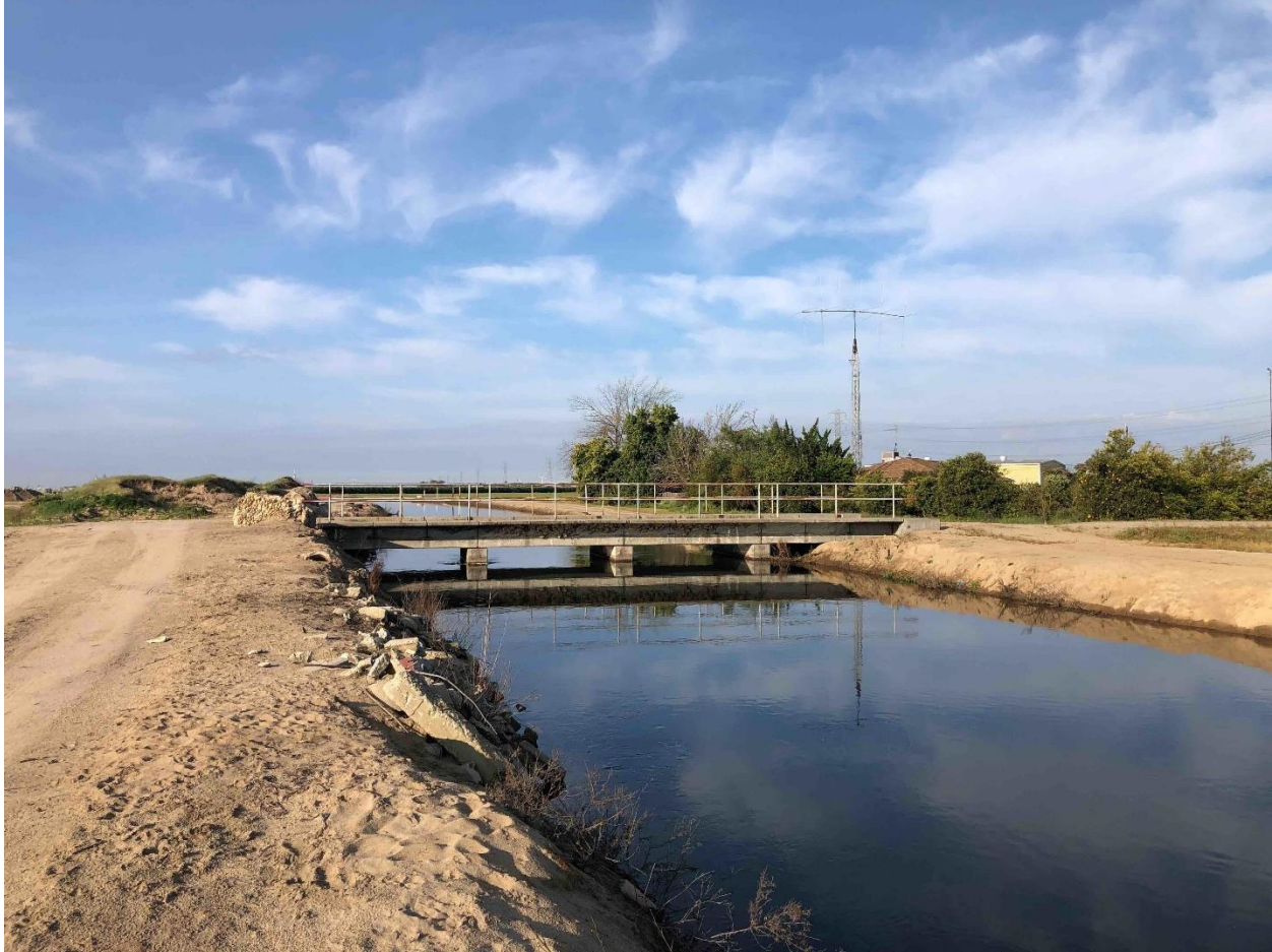
Figure 3-3. Mill Ditch Canal
