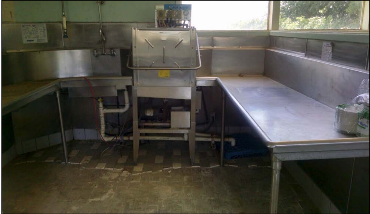
Figure 34. Kitchen dish-washing area with stainless steel equipment in place.
