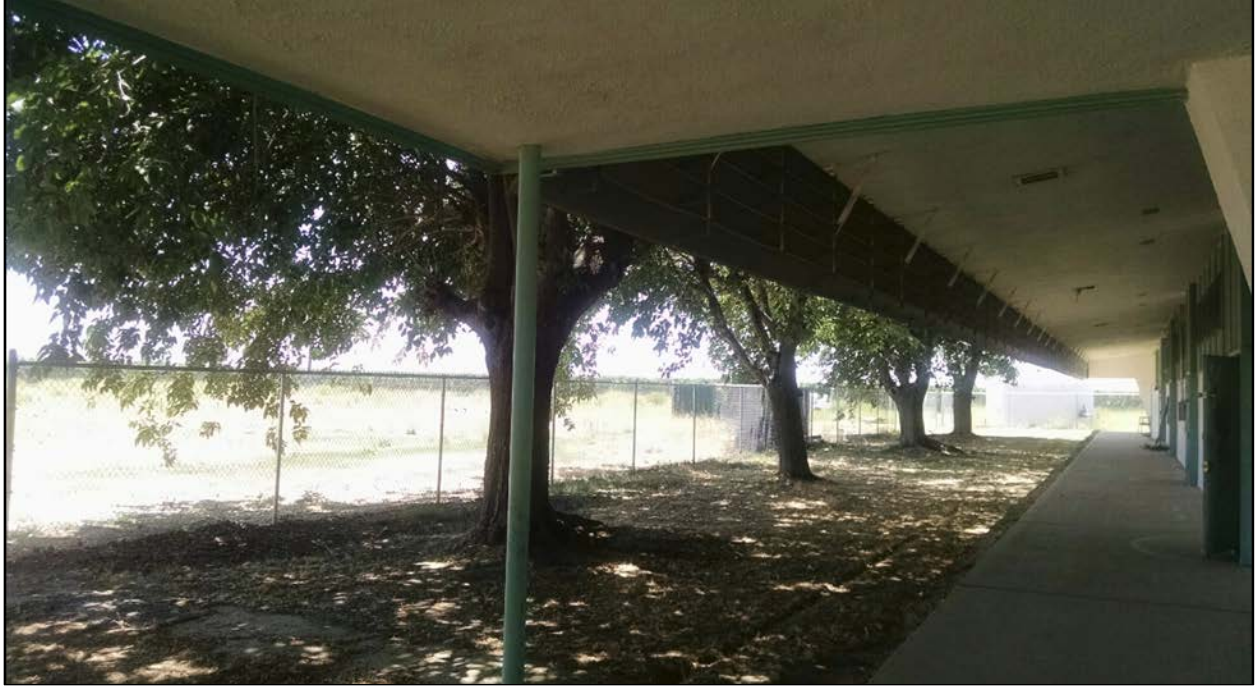
Figure 74. Corridor and row of trees on south side of Classroom Building D.
