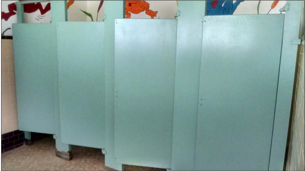
Figure 68. Original stalls in girls' bathroom, Classroom Building D.
