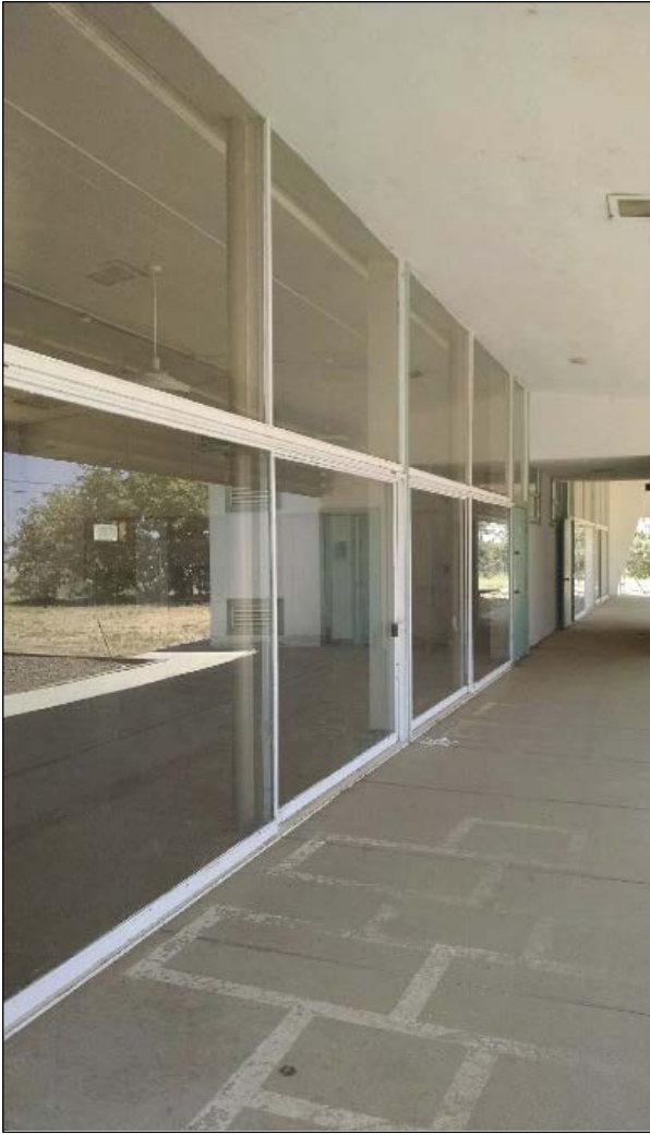
Figure 38. Oblique view of north side of Kindergarten Building B, showing glass-walled classrooms sheltered by covered corridor.
