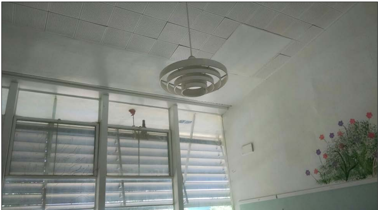
Figure 73. Original classroom interior (except decorative painting), Classroom Building D.
