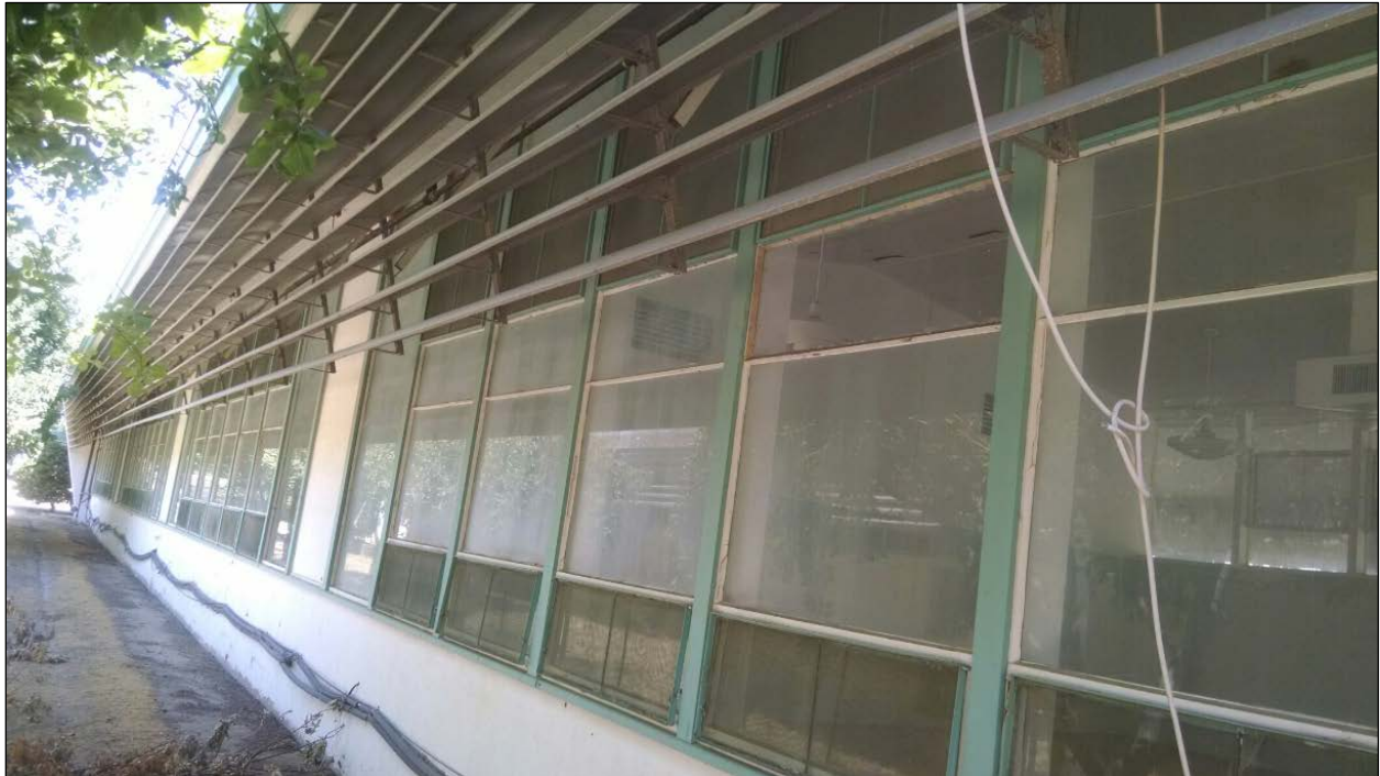
Figure 62. North elevation of Classroom Building D, showing original windows and louvers.
