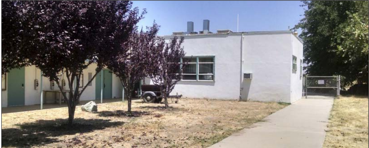
Figure 22. Flat-roofed kitchen annex on south side of multi-purpose room
