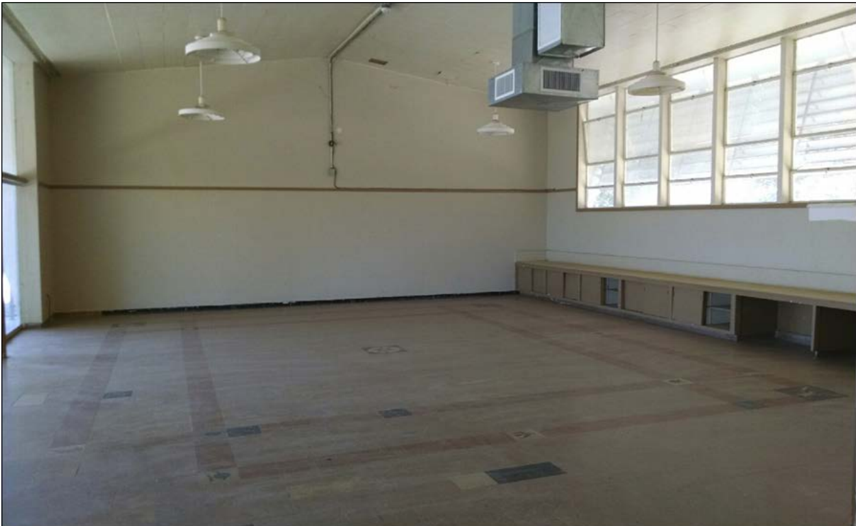
Figure 43. Kindergarten classroom at east end of Building B. Except for the heating, ventilation, and air conditioning (HVAC) and sprinkler system, all materials are original. Massed four-light windows on the south wall have operable hopper sash.
