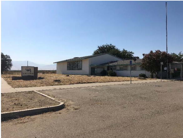
Photo #1 View of the Site from David Road, facing southeast.
