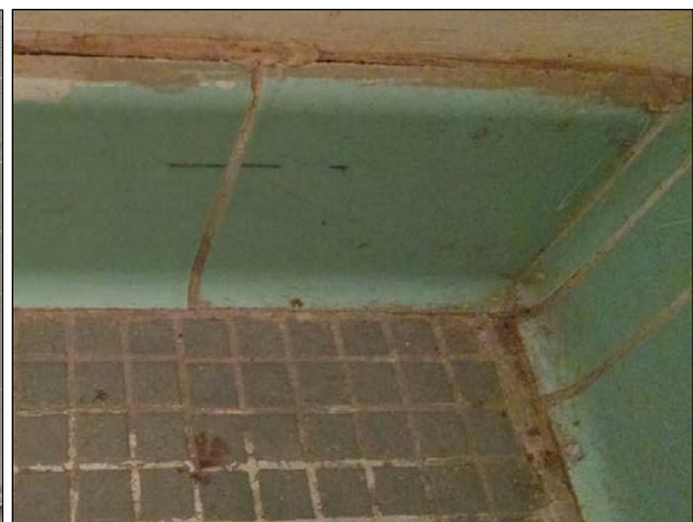
Figure 49. Original ceramic tile flooring and baseboard in bathroom.
