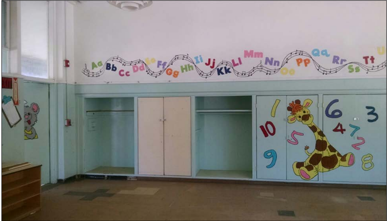
Figure 72. Original classroom interior (except decorative painting), Classroom Building D.
