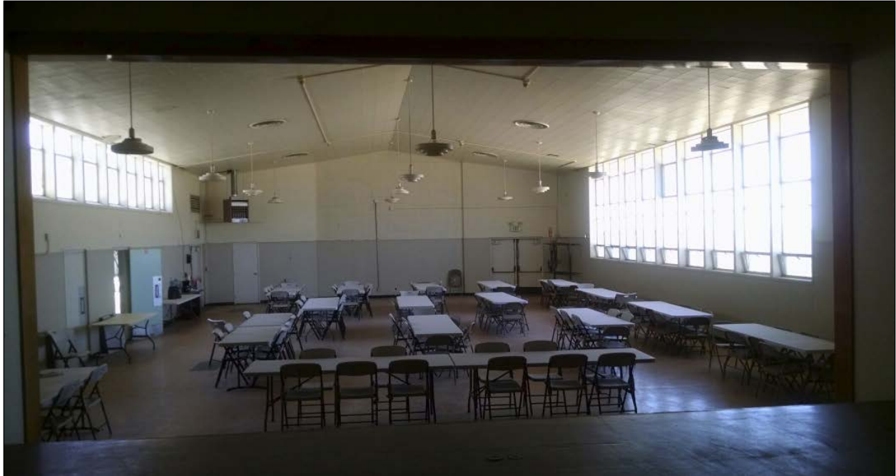
Figure 30. View from stage across multi-purpose room to west wall.
