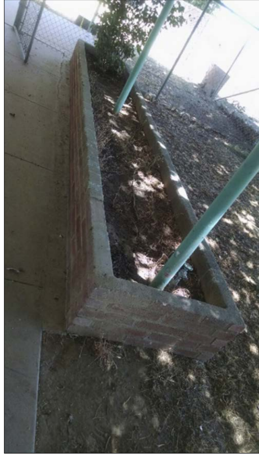
Figure 64. Brick planter at southwest corner of Classroom Building D.
