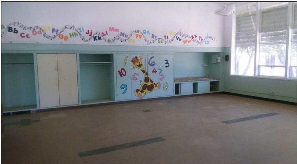
Figure 71. Original classroom interior (except decorative painting), Classroom Building D.
