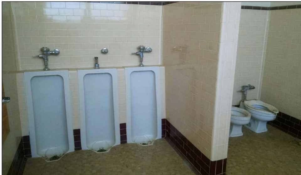
Figure 65. Boys' bathroom in Classroom Building D, with original ceramic wall tile and fixtures.
