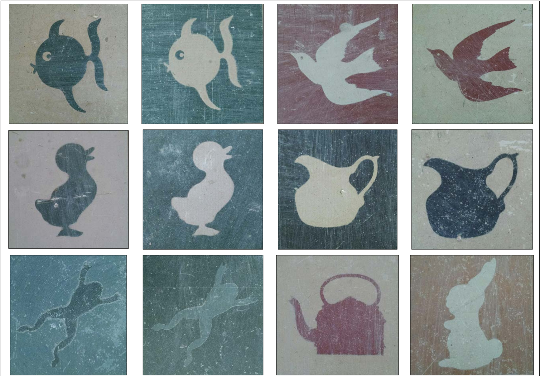
Figure 46. Kentile vinyl-asbestos “ThemeTile” installed in kindergarten classroom flooring.
