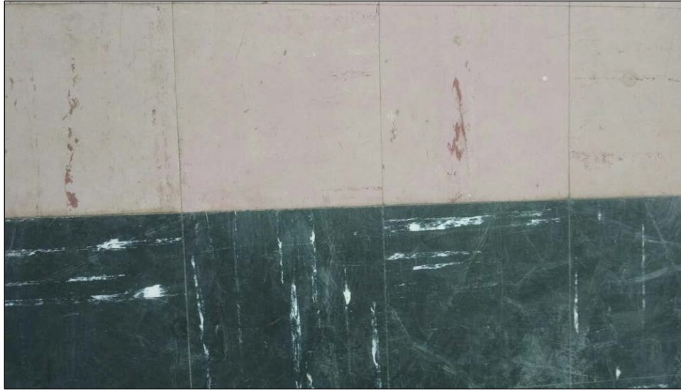
Figure 32. Floor tiles (probably manufactured by Kentile) at entrance to kitchen annex.
