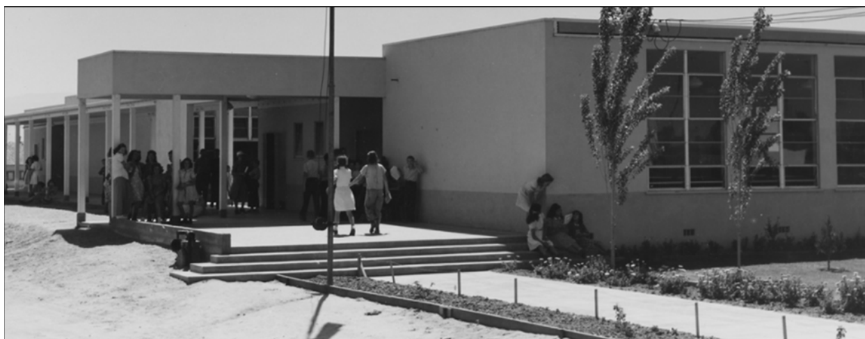
Figure 5. The new Arvin School buildings, designed by Frank Wynkoop and Associates, were photographed by famed New deal photographer Dorothea Lange on April 11, 1940.
