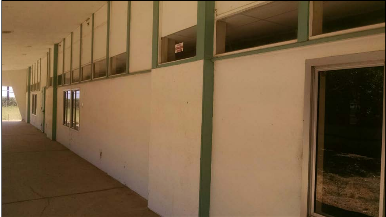
Figure 60. View down corridor of Classroom Building C, showing altered window openings.
