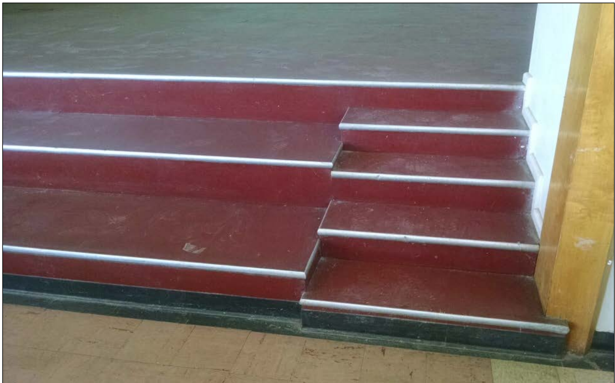
Figure 29. Steps and risers at front edge of stage.
