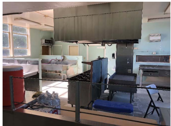
Photo #12 Interior of the kitchen, facing southwest.
