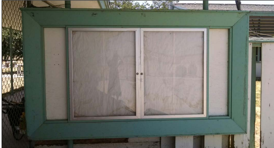
Figure 14. Wood-framed bulletin board with inset metal-framed glass doors, mounted on steel poles, at front entrance to campus.
