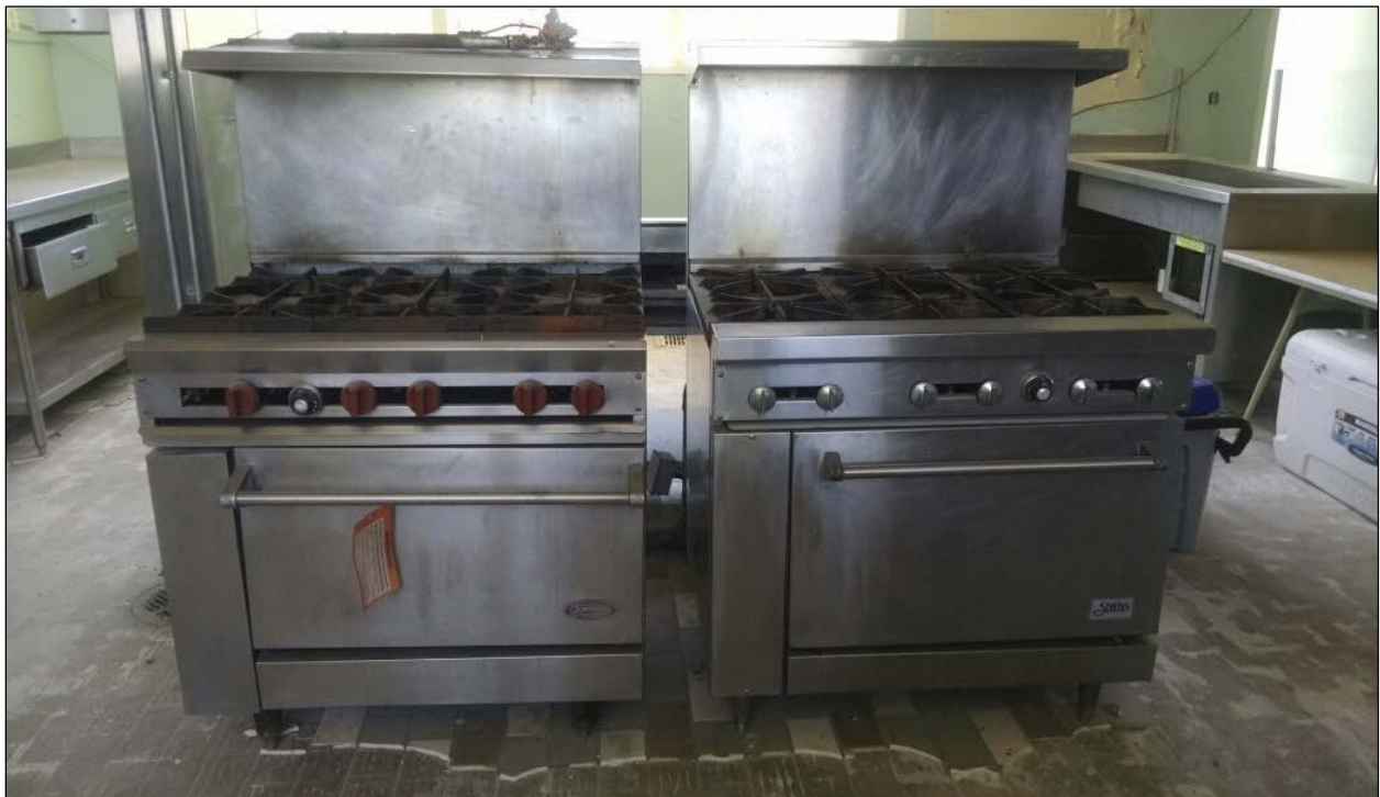
Figure 35. Kitchen ranges; tile flooring partially removed.
