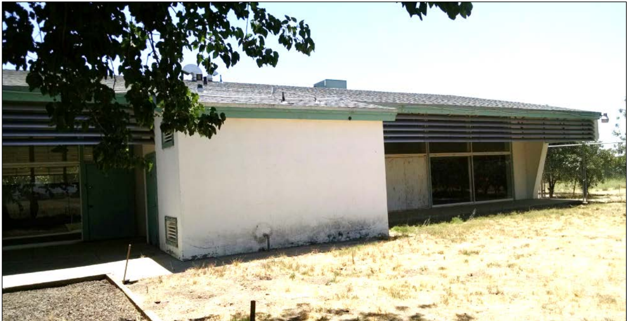
Figure 41. West end of Kindergarten Building B; note angled architectural element supporting corridor roof. This architectural detail appears at the ends of all classroom corridors.
