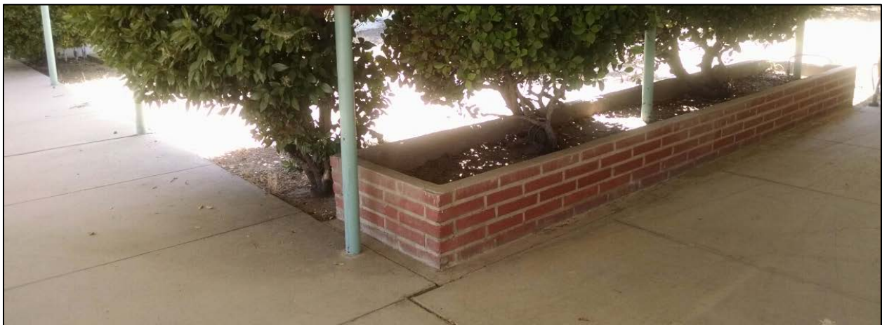
Figure 61. Brick planter at intersection of main covered walkway and corridor of Classroom Building C; bricks, laid in running bond, are more elongated than common brick.
