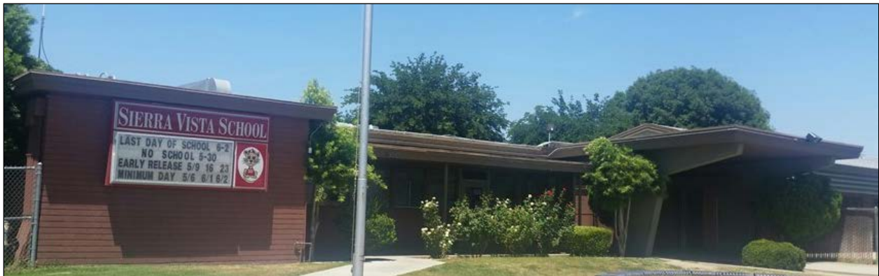
Figure 79. Entrance to Sierra Vista School completed in January 1954. The cantilevered entrance canopy opens directly onto the axial covered walkway.
