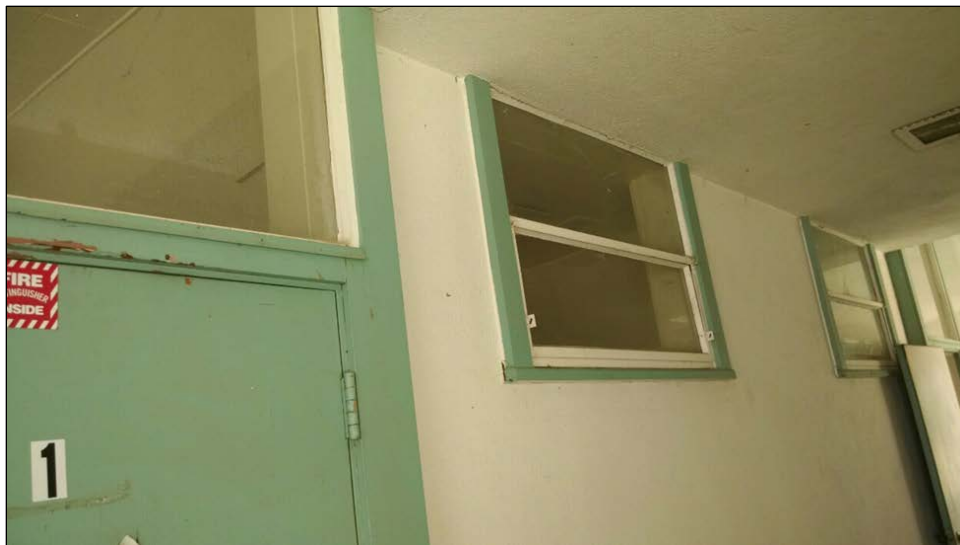
Figure 59. Windows (including glazed transoms) on Classroom Building C corridor.
