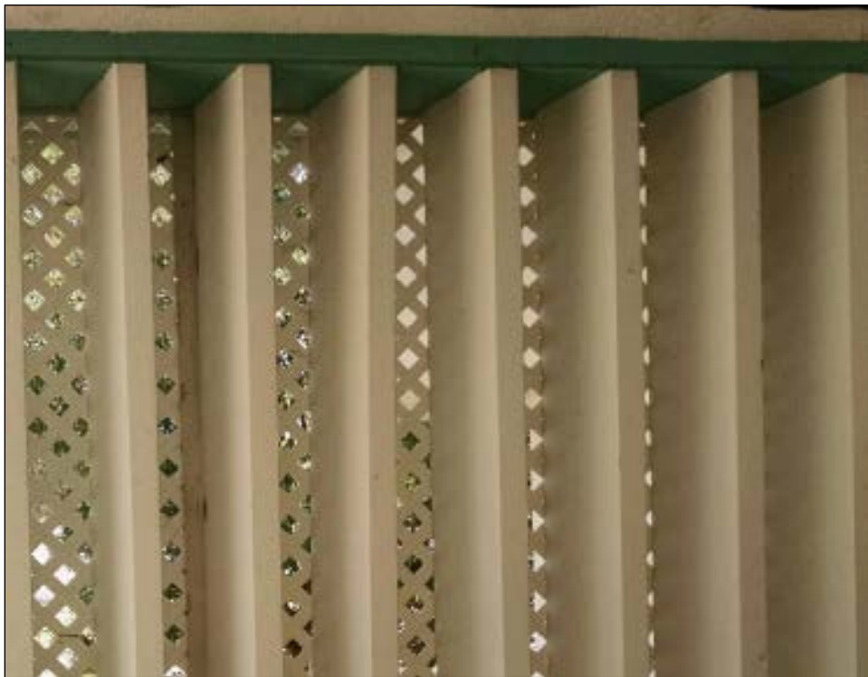
Figure 17. Detail of vertical louvered screen; lattice added at a later date.
