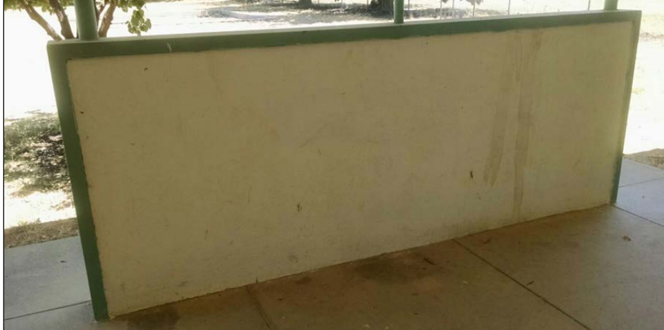
Figure 76. Half wall element on main covered walkway, screening bathroom doorways.
