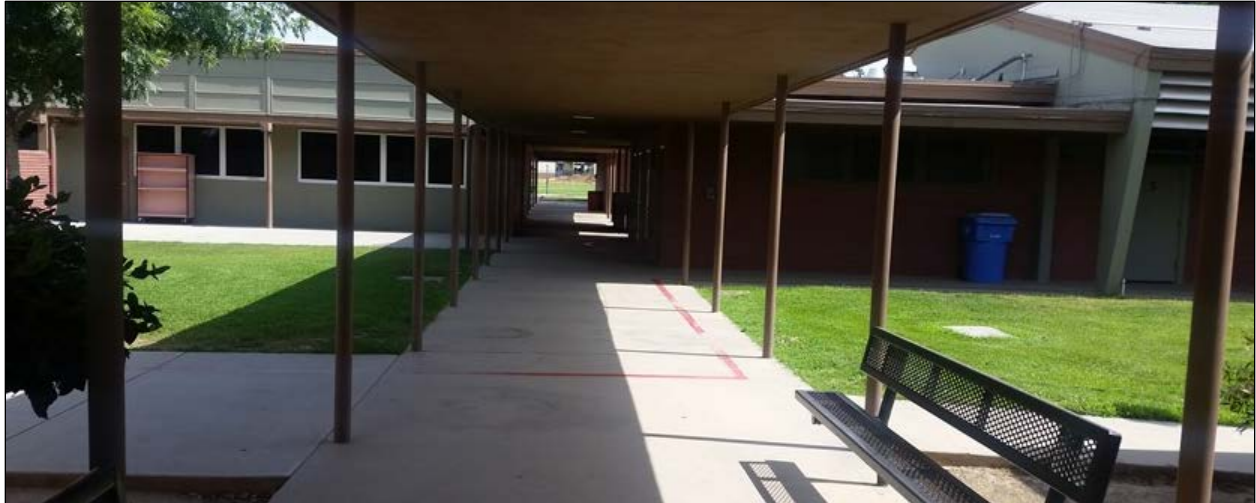
Figure 80. Main axial covered walkway that leads to Sierra Vista School classroom wings arranged in “finger-plan” layout.”
