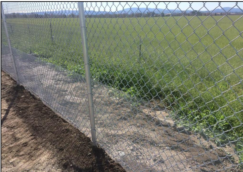
Photo 4: Recently installed small mammal exclusion fence attached to the chain link boundary fence on February 6, 2019.
