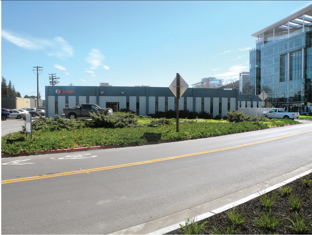
Photo 1: Existing building, as seen from Independence Drive/Constitution Drive
