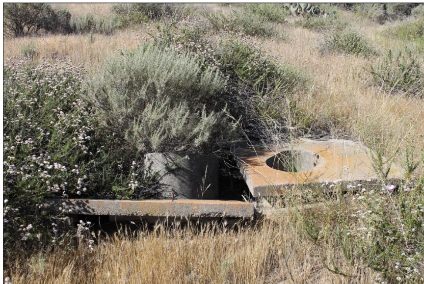
Photograph 10. Overview of P-30-001200 and vegetation coverage, facing south.
