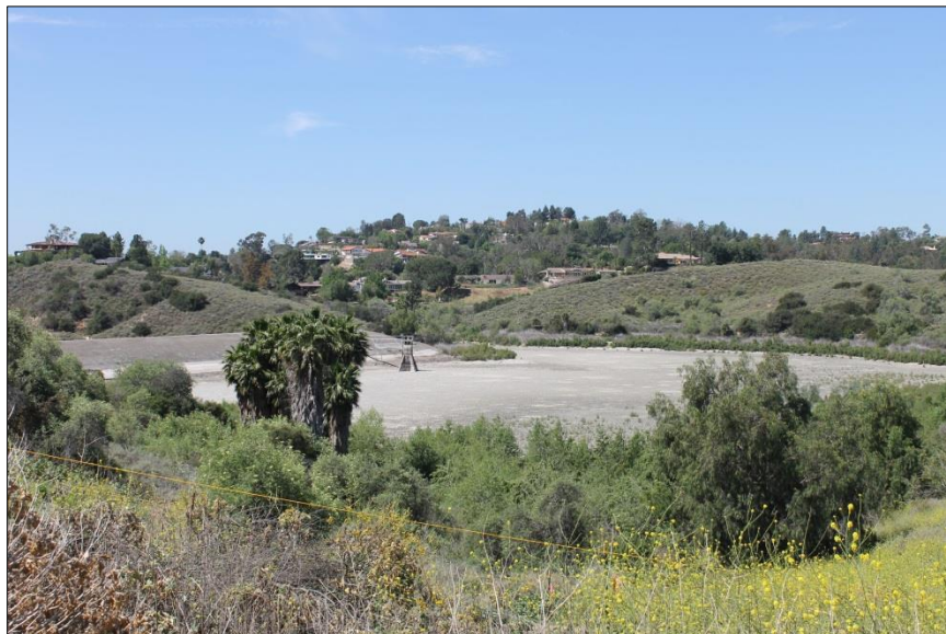
Photograph 4. View of Upper Peters Canyon Reservoir and Dam, facing west.
