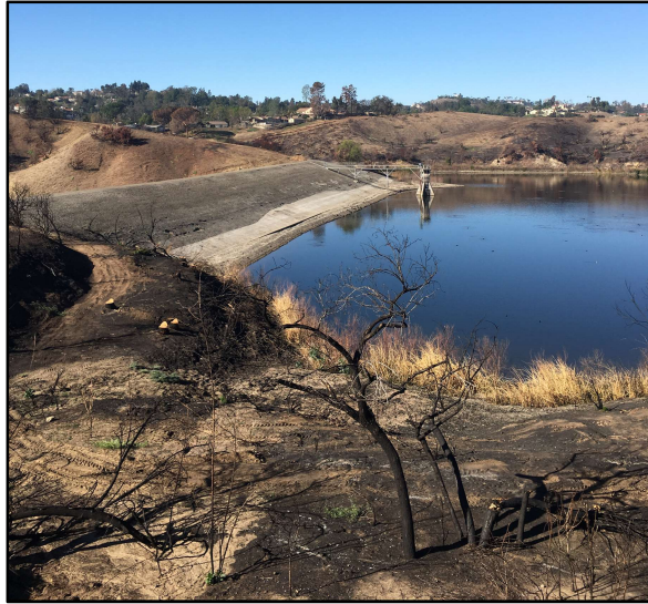
Photograph 1. Peters Canyon Dam and Reservoir with standpipe visible, facing west.
