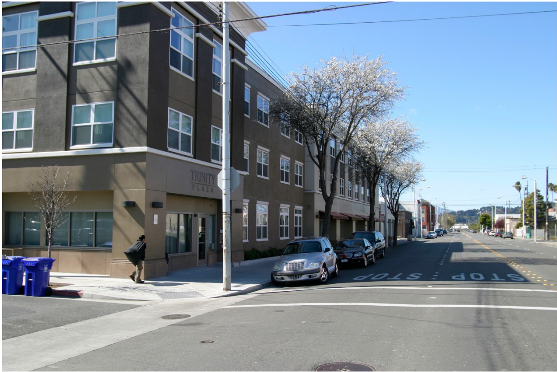
a) Senior apartments in the 300 block of Macdonald Avenue, one block east of the project site
