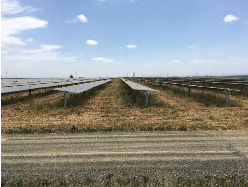
Photo 1. View of the solar panels in the existing RE Mustang SGF showing spacing between rows and mowed herbaceous cover under and between the rows of panels. The photo was taken looking east from the western boundary of the site.
