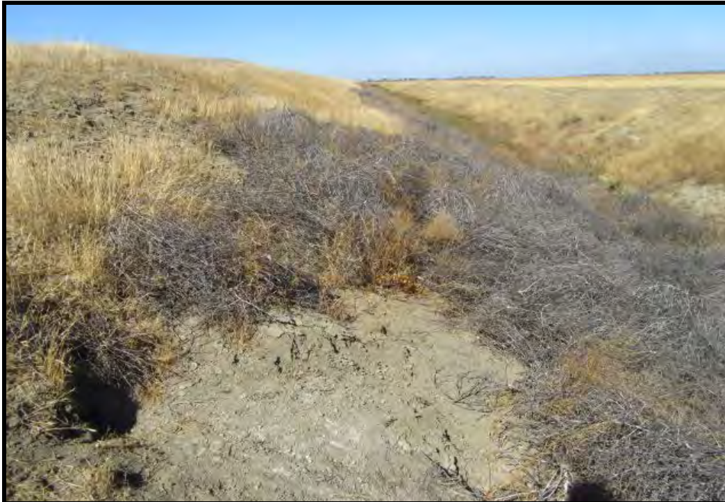
Photograph 2: Representative dry canal and berm with ground squirrel burrows.
