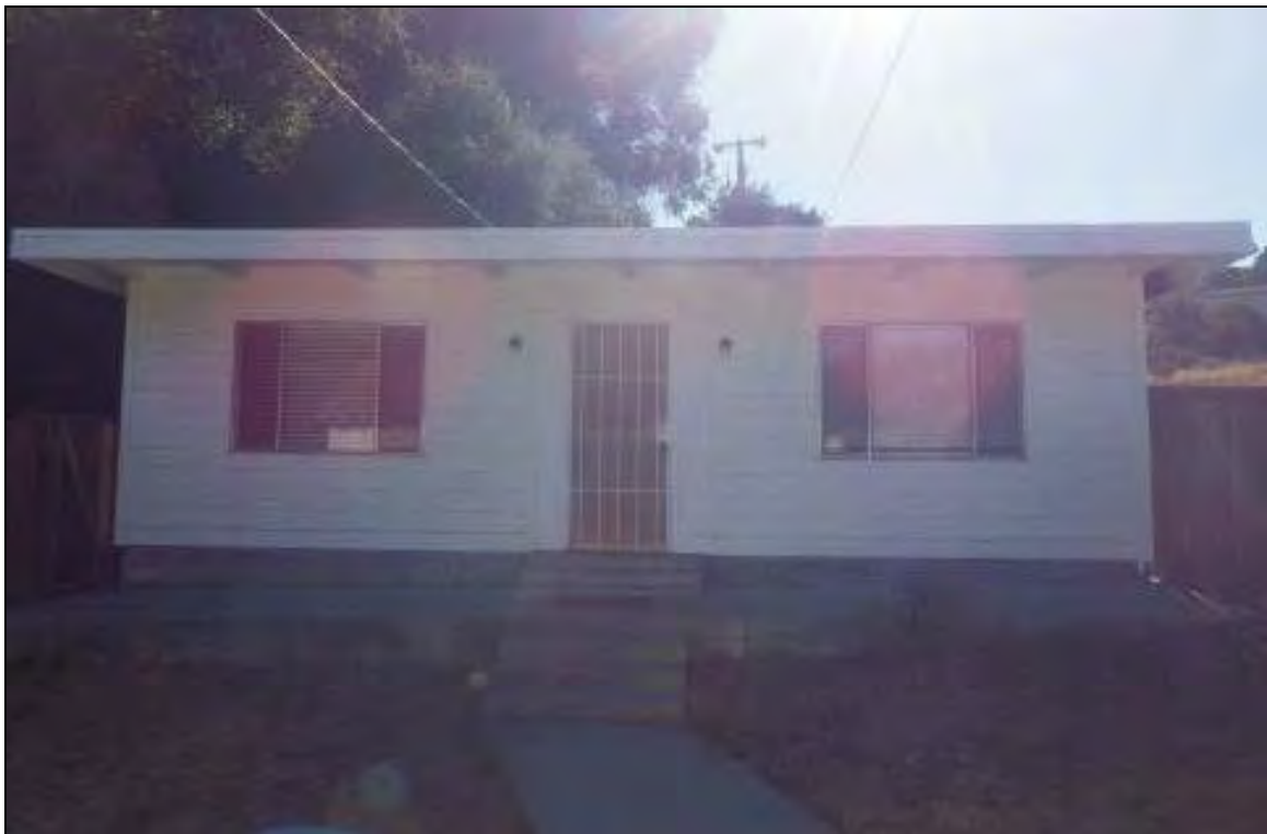
Figure 4-12 Structure 2 - shed residence front, west elevation, facing east.
