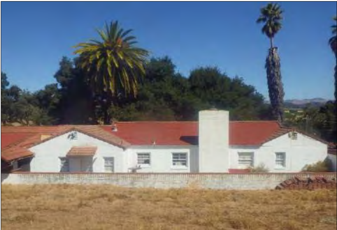
Figure 4-6 Structure 1 - primary residence rear, south elevation, facing north.
