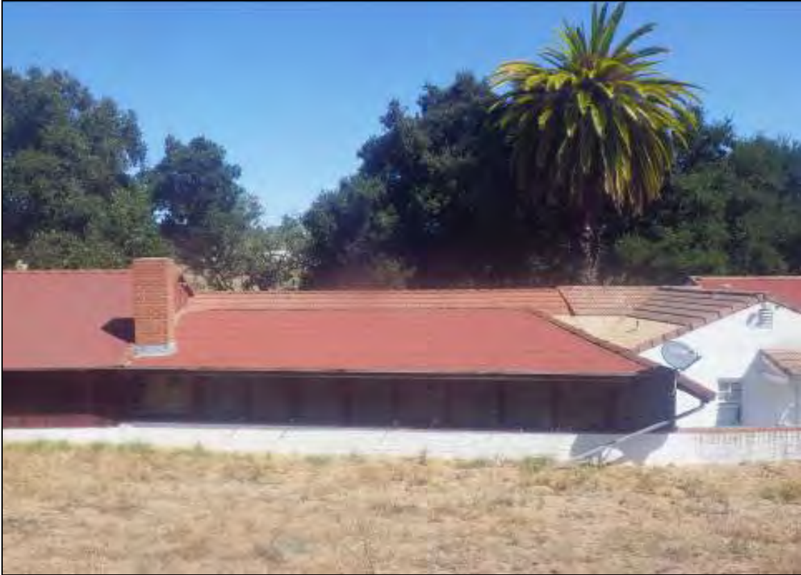
Figure 4-9 Structure 1 - sun room rear, south elevation, facing north.
