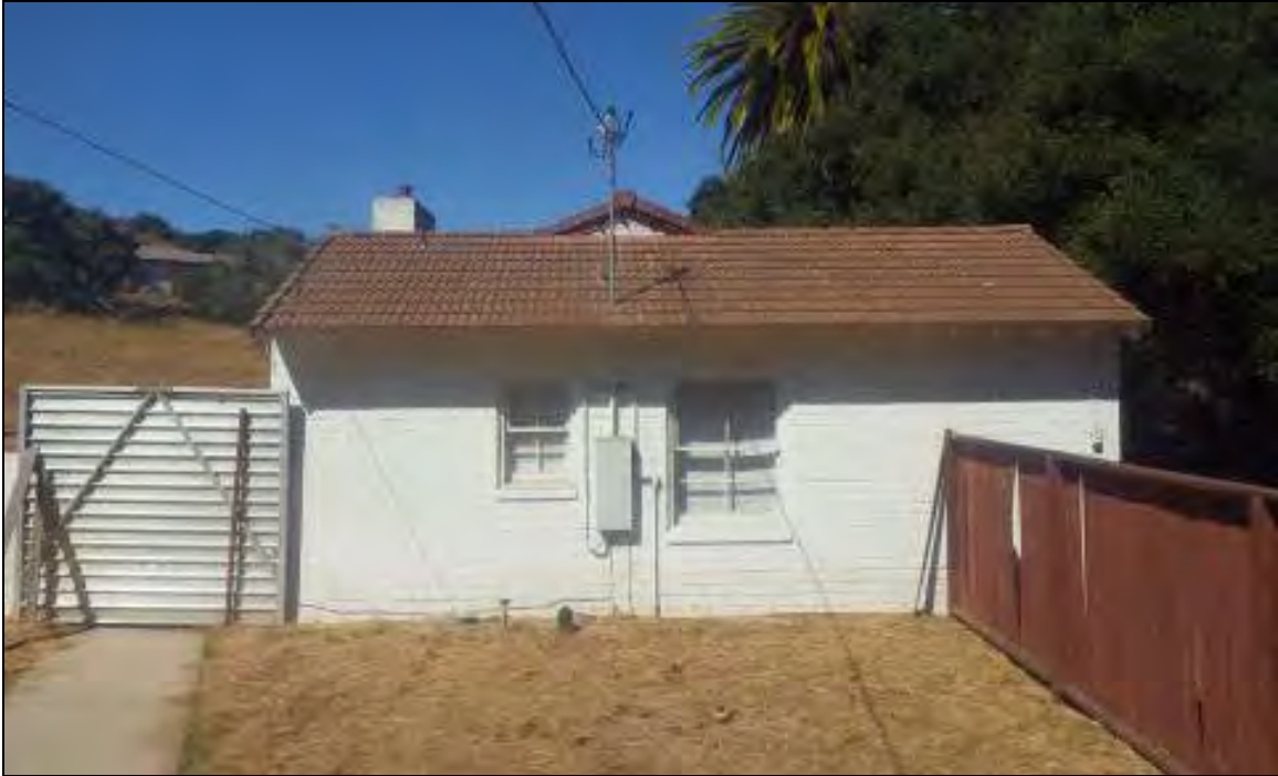
Figure 4-7 Structure 1 - primary residence, side, east elevation, facing west.
