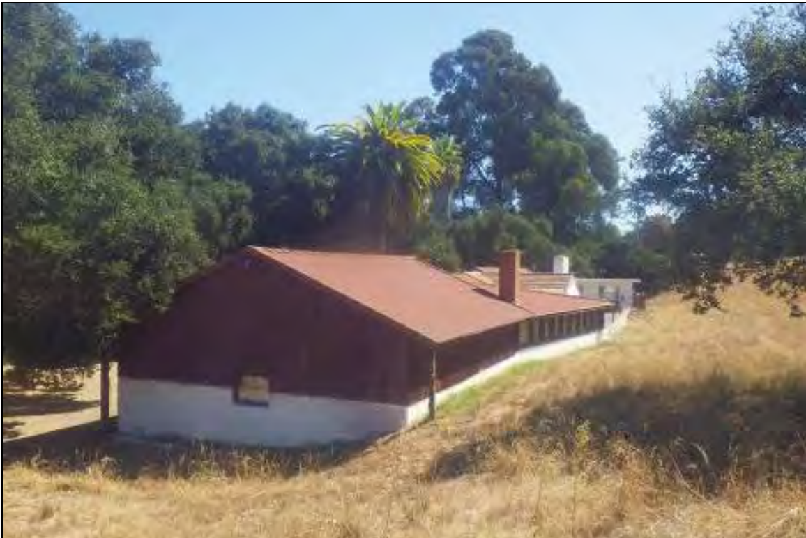
Figure 4-11 Structure 1 - garage addition, side (west) and rear (south) elevations, facing northeast.
