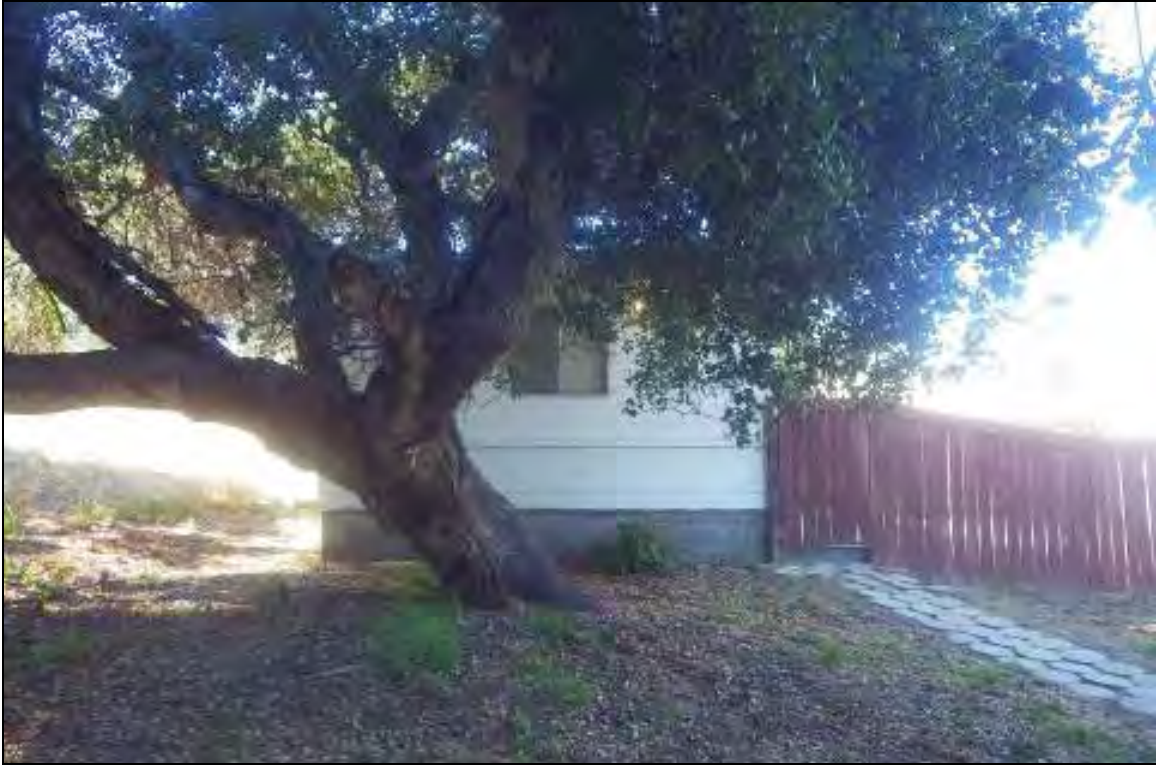
Figure 4-13 Structure 2 - shed residence side, north elevation, facing south.
