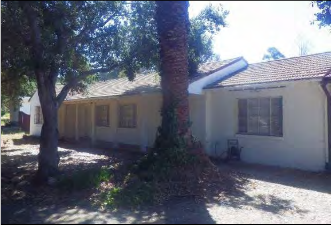
Figure 4-5 Structure 1 - primary residence front, north elevation, facing east, southeast.
