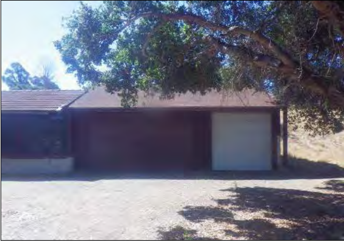
Figure 4-10 Structure 1 - garage addition front, north elevation, facing south.
