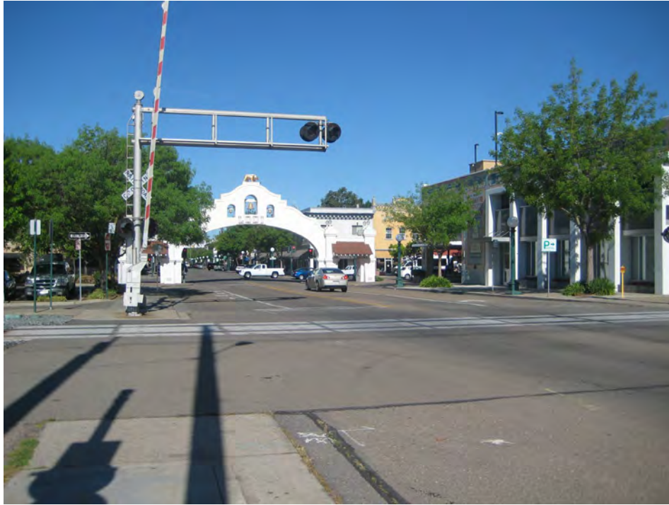
Photograph 2. View of south elevation of parking garage and Mission Arch, facing northwest.
