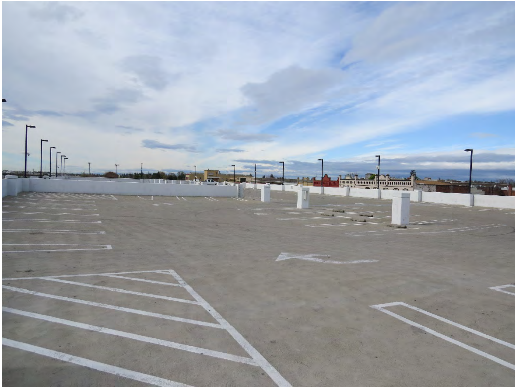
Photograph 4: From the northwest corner of the Parking Garage site looking south.
