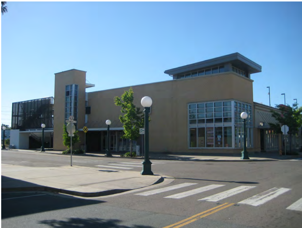
Photograph 3. North elevation of parking garage, facing south-southeast.
