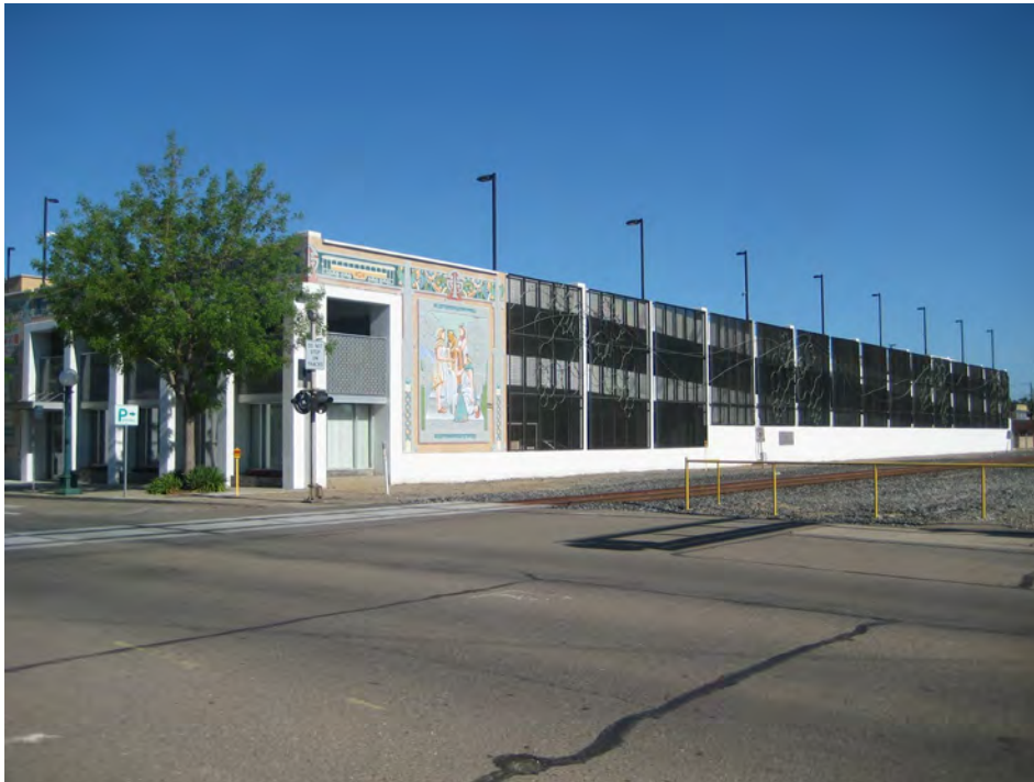
Photograph 1. Overview of east side of project site, facing northwest.
