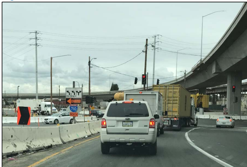
Figure 2.4 EB W Ocean Boulevard / I-710 NB Off-Ramp to Pico Avenue
