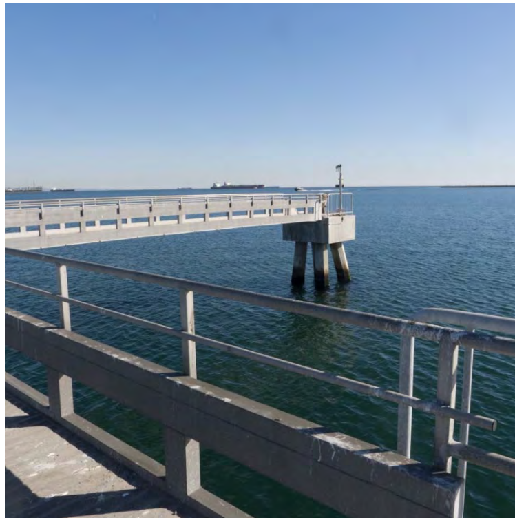
Photo 17: Facing southeast- View of southern catwalk to southern mooring dolphin.
