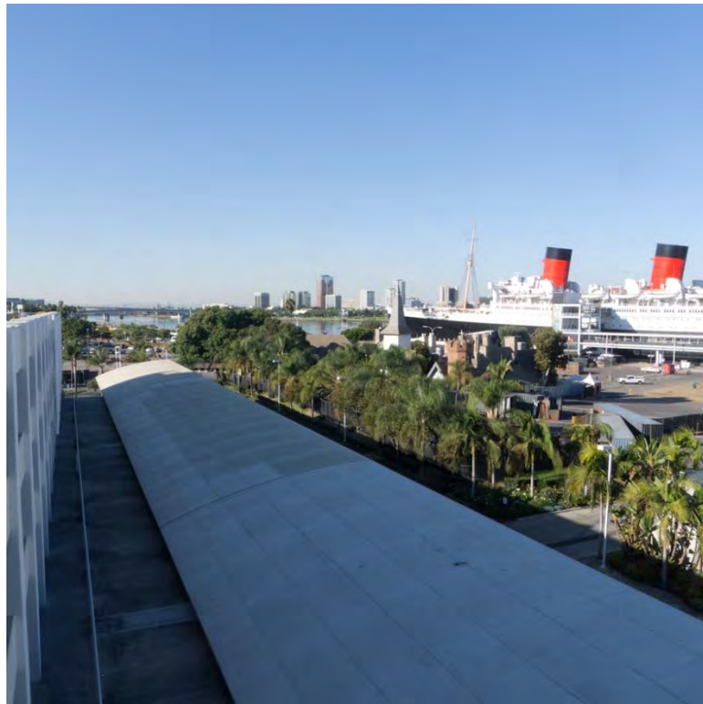
Photo 21: Facing northwest - Overview of parking expansion area and Queen Mary.
