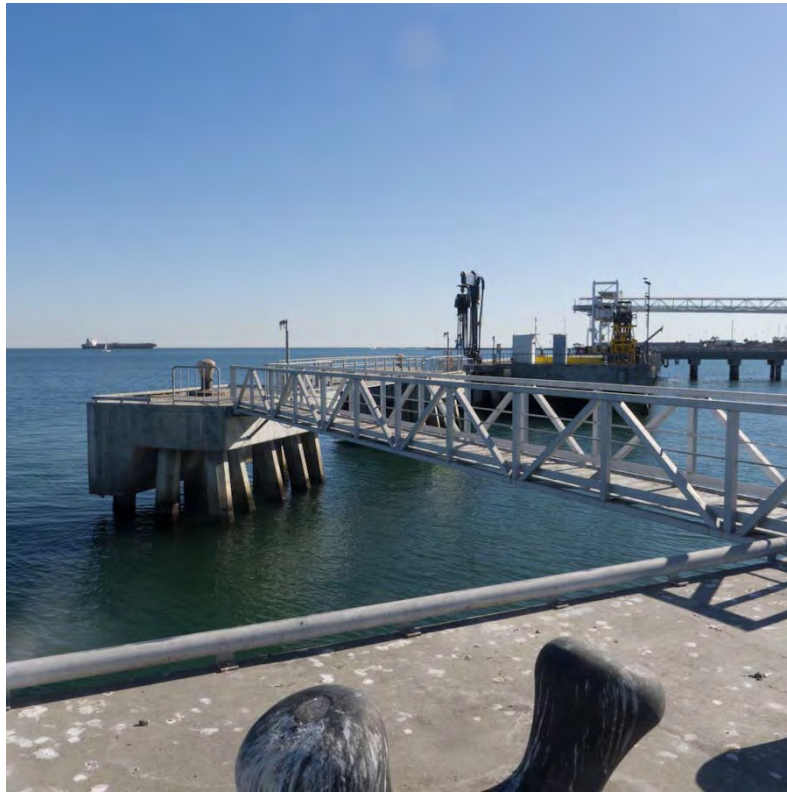
Photo 7: Facing south- View of catwalk to passenger gangway.
