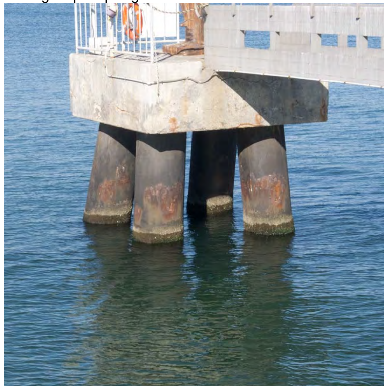
Photo 38: Facing northeast- View of mooring dolphin pilings.
