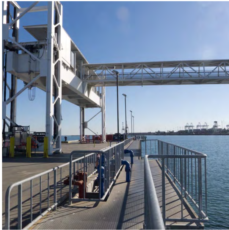
Photo 13: Facing northwest- Close-up view of passenger gangway.
