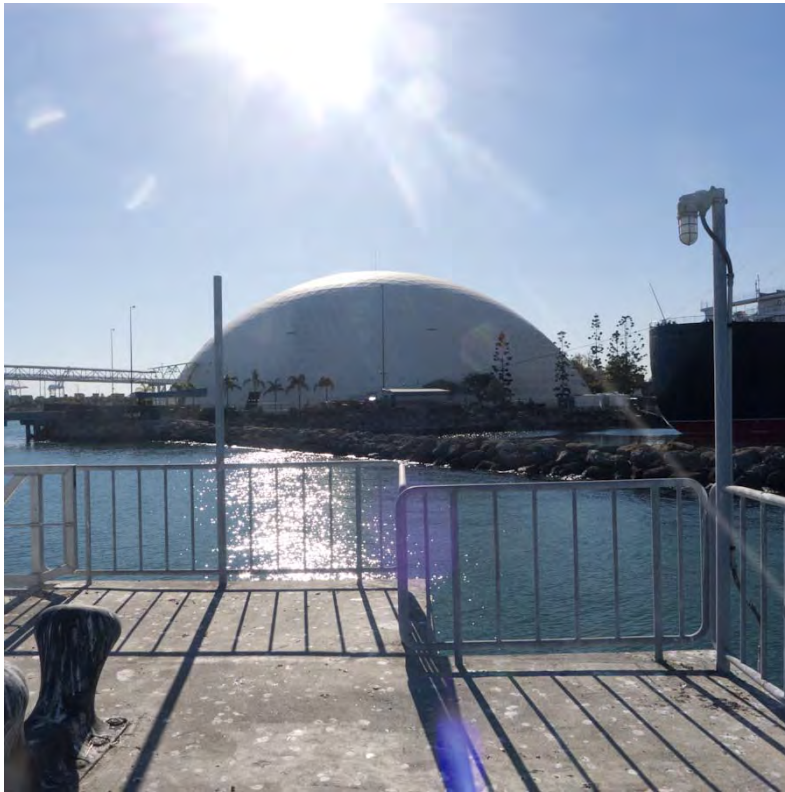
Photo 5: Facing southwest- View of Long Beach Cruise Terminal building seen from dock.
