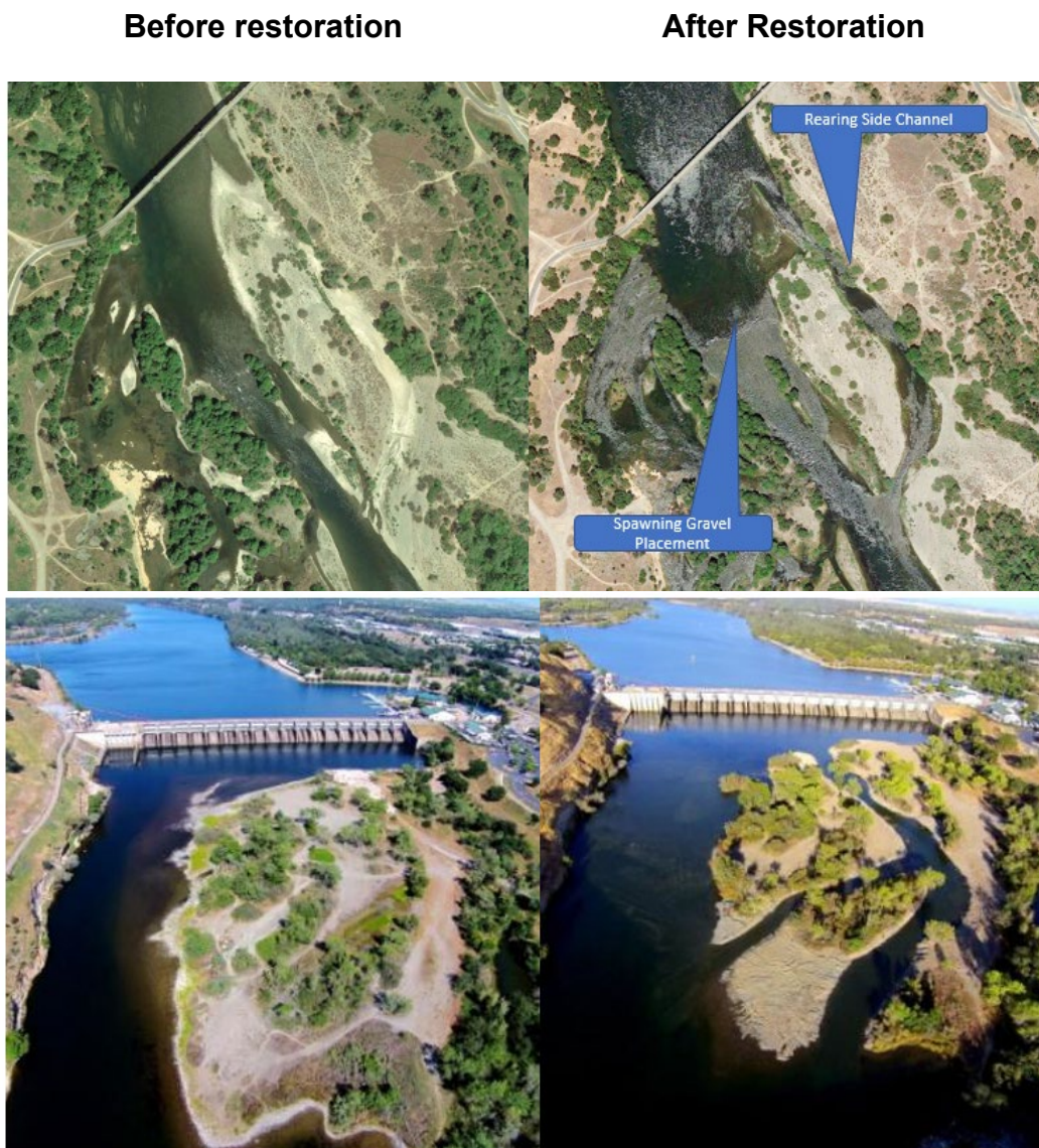
Figure 2-1. Example Floodplain and Side Channel Creation at River Bend (top photos) and Nimbus Basin (bottom photos)
