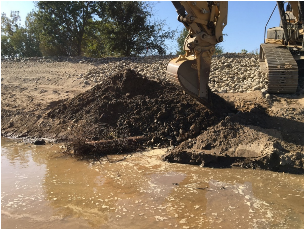
Figure 2-3. Woody Material Placement from Sacramento Bar, 2016
