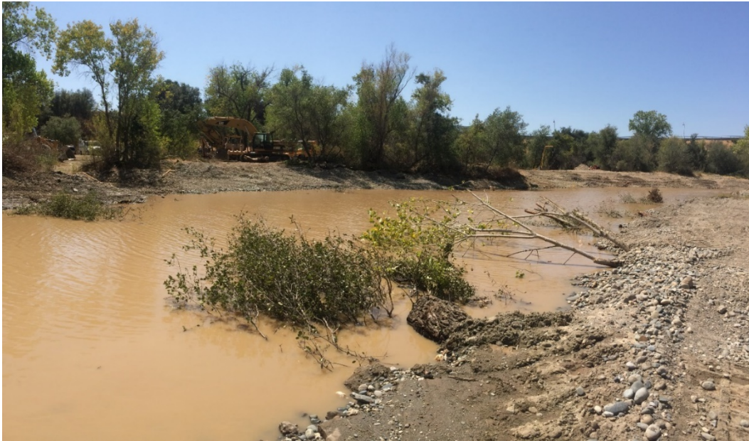
Figure 2-2. Example of Woody Material Placement - Nimbus Basin, 2014
