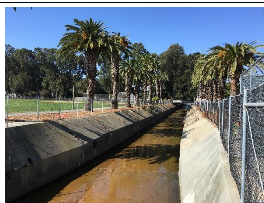
Photo 1. The Project site is located along Colma Creek, a concrete lined channel that traverses the southern half of Orange Memorial Park near two ballfields (left).
