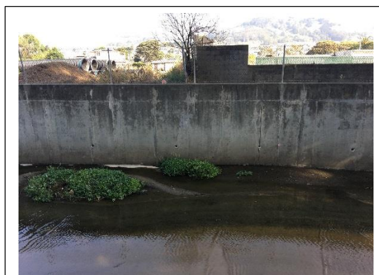
Photo 7. Narrow strips of riparian vegetation are visible along the concrete bottom channel where patches of sediment accumulated.
