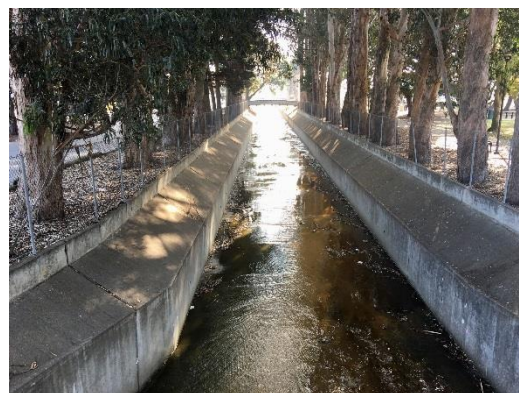
Photo 6. Colma Creek consists of a perennial and intermittent drainage within a concrete lined channel that bisects Orange Memorial Park.
