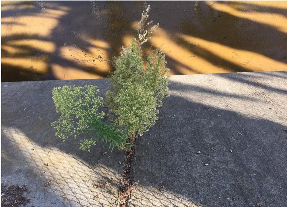
Photograph 17. Vegetation growing out of the crack between concrete slabs lining Colma Creek channel.
