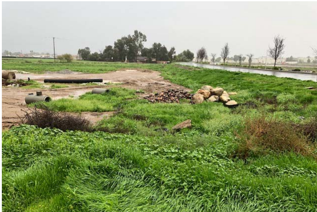
Photograph 6: Photograph depicting off site improvement areas.
