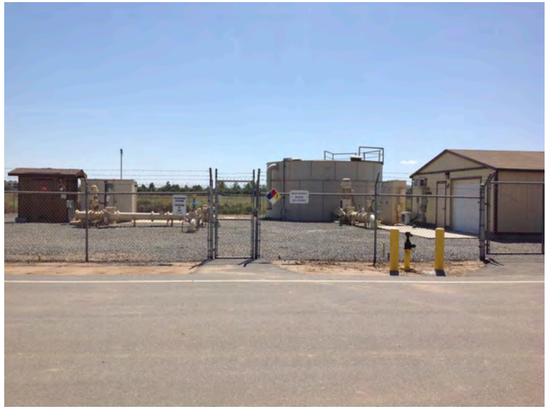
Looking at EWMD Well Site North of Site
