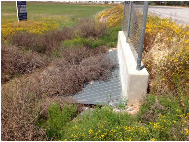
Location of storm drain inlet at Southeast corner
