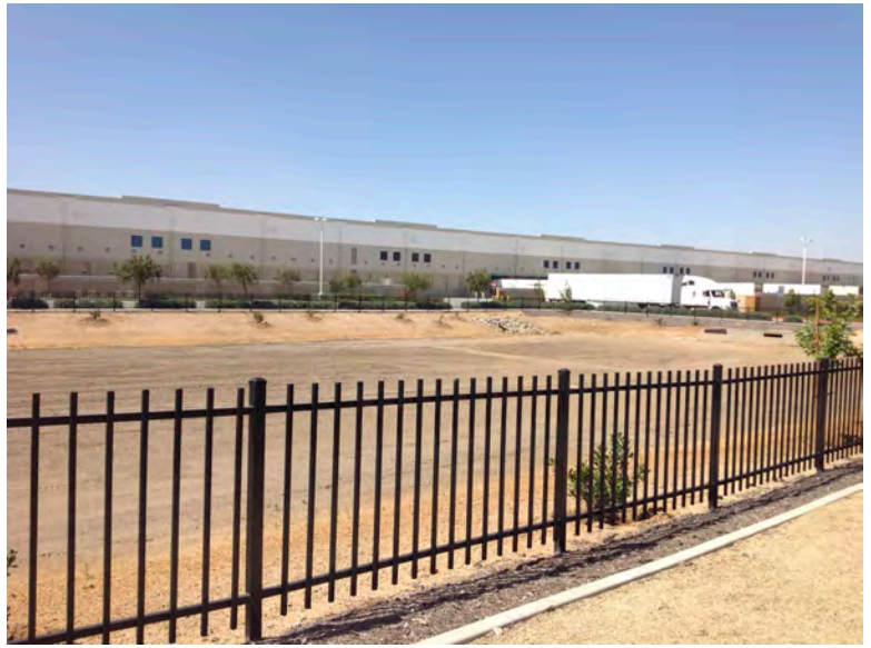
Stormwater retention system at Site boundary
