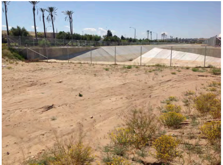
Stormdrain at Southwest corner
