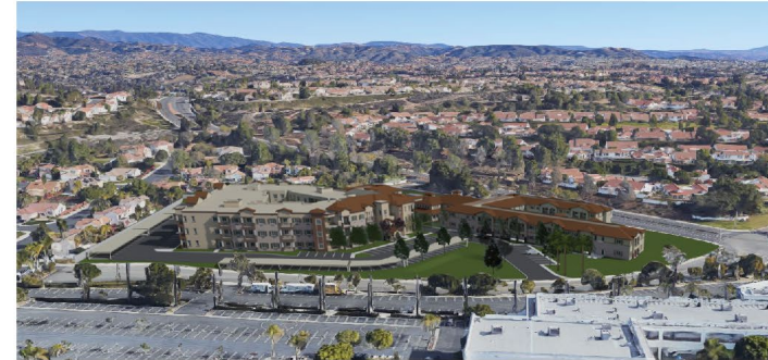
Ocean Hills Senior Living Phase II - Aerial from the West
