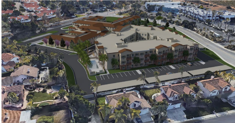
Ocean Hills Senior Living Phase II - Aerial from North
