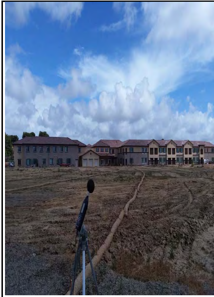
NM2 looking SE across graded land towards the project site.
