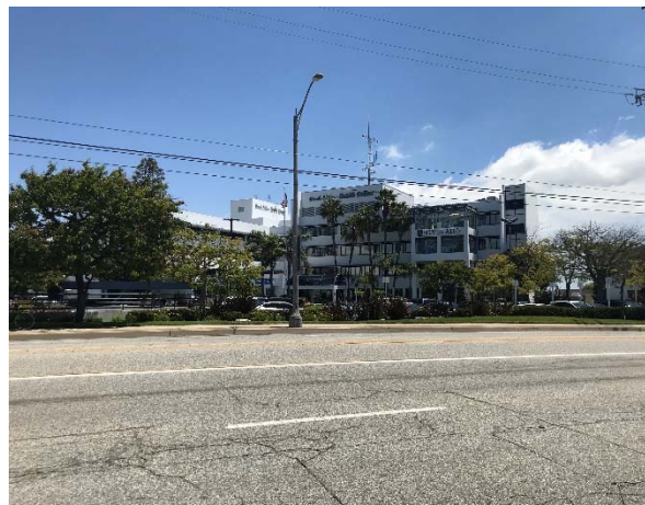
Photo 9. The existing Beach Cities Health Center is highly visible from surrounding roads, sidewalks, and similar public spaces. This five-story building would be demolished and replaced with a four-story RCFE building and a three-story CWP that would both reach a maximum height of 60 feet.
