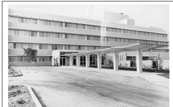
Photo 12. The former South Bay Hospital was originally constructed beginning in May 1958 and was opened in August 1960, providing 150 beds, three major surgery rooms, minor surgery rooms, emergency operating areas, administrative facilities, offices, small stores and coffee shops, and other similar type uses.
