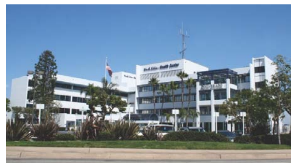
Photo 1. The existing BCHD campus features the former five-story South Bay Hospital that was closed in 1998 and is currently operated as the Beach Cities Health Center, providing community wellness and senior care services (e.g., memory care).
