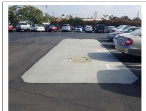
Photo 13. The existing campus includes a 10,000-gallon former underground storage tank located beneath the surface parking lot. Soil samples collected in January 2008 during the replacement of piping lines identified the presence of petroleum hydrocarbons that exceeded established maximum concentrations.
