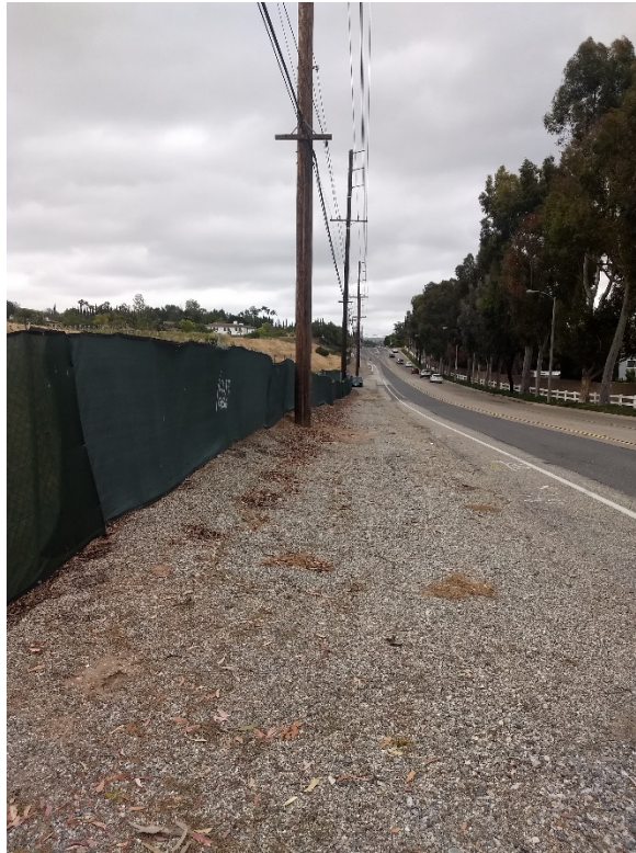
Northwest end of Project Site, view to the East
