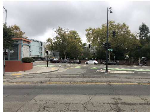
Photo 17- View of the northern portion of the project site from College Avenue
