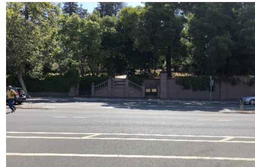
Photo 19- View of the entry staircase from College Avenue.
