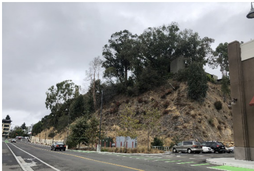
Photo 12- View of project site's southern precipice from Access Road below
