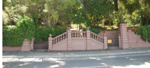
Broadway Wall and Stairs
