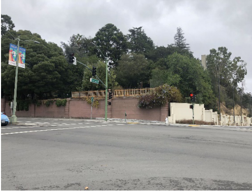
Photo 16- View of the southwestern corner of the project site from the corner of Broadway and Coronado Avenue
