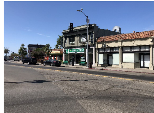
Photo 8- Older 1- and 2-story commercial buildings
