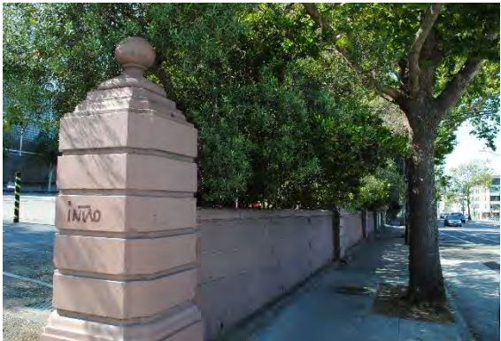
Figure 27. Broadway Wall, northernmost pier, facing southeast.
