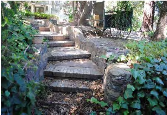
Figure 165. Staircase paved with Carnegie bricks, flanked by masonry retaining walls with ceramic pots.
