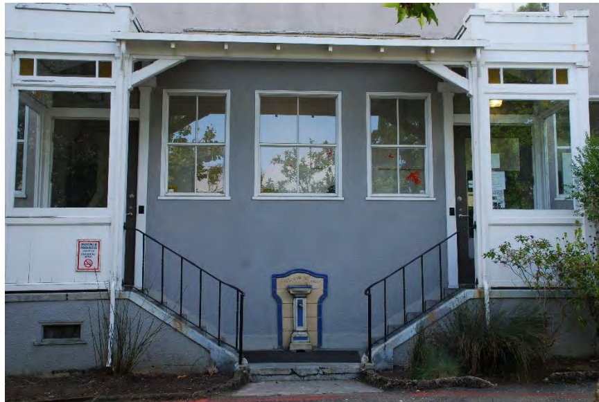
Figure 44. The B Building, west façade detail, primary entrances and tile fountain, facing east.
