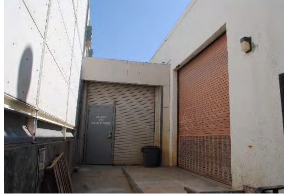
Figure 144. Metal roll-up door accessed via a concrete ramp on the north side of the hyphen between Barclay Simpson Sculpture Studio (left) and the Shaklee Building (right).
