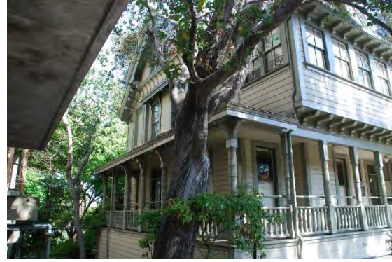
Figure 14. Macky Hall, south façade, first story, partial view, facing northwest.
