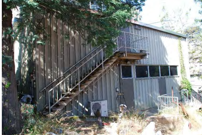
Figure 95. North façade of Martinez Hall Annex, looking southwest.
