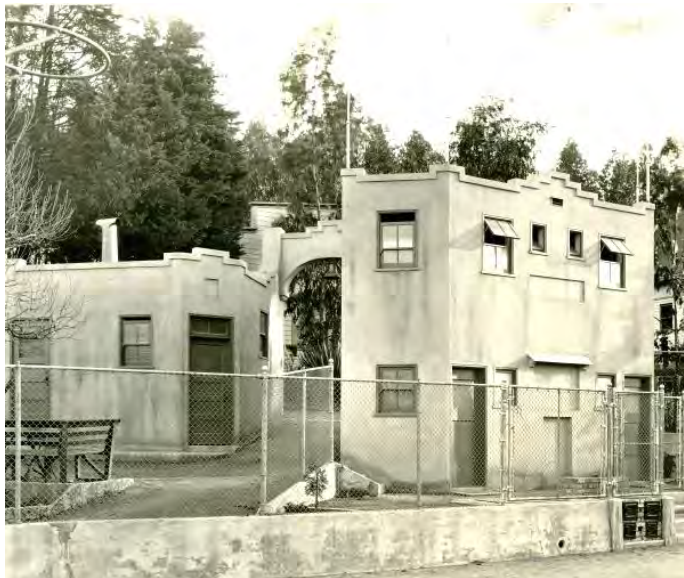
Figure 228. Shower Building, 1930, facing southeast, no longer extant.
