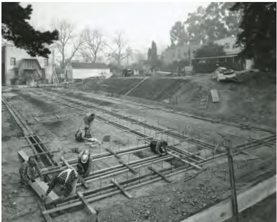
Figure 60. Irwin Hall under construction, 1958. Source: CCA Libraries Special Collections.
