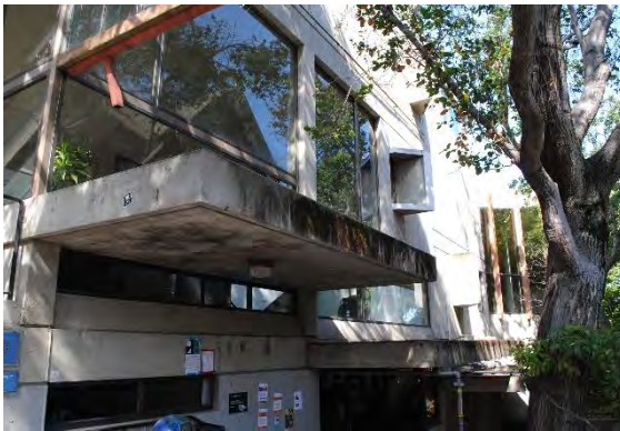
Figure 84. Founders Hall, north façade, facing southwest.
