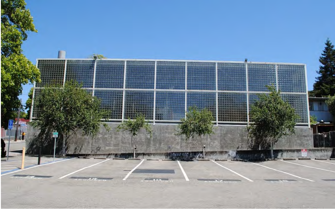
Figure 137. West façade of the Barclay Simpson Sculpture Studio, looking east.
