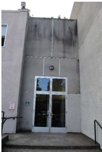
Figure 132. Hyphen volume with ADA-accessible entrance at the north end of the west façade of the Oliver & Ralls Building, abutting the B Building (left), looking east.
