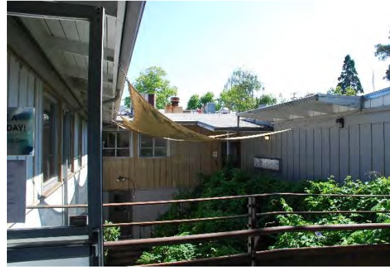
Figure 57. South façade of the east-west wing of Irwin Student Center (center) and A-2 Café addition (left), looking north.
