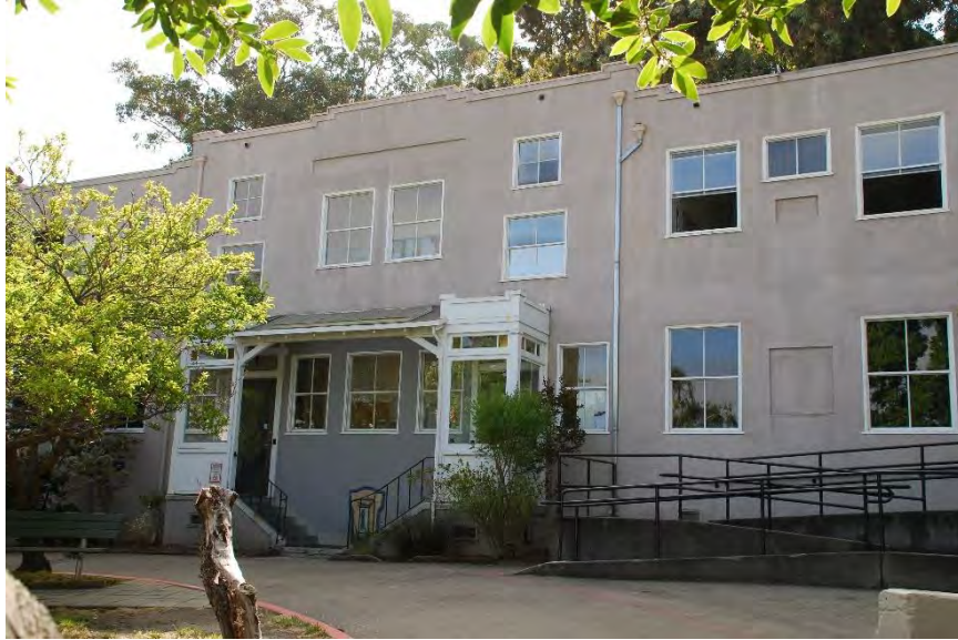
Figure 43. The B Building, west façade, facing northeast.
