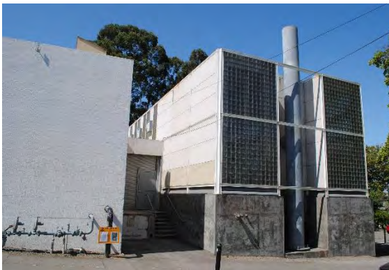
Figure 141. East and north facades of the Barclay Simpson Sculpture Studio, looking southwest. The Shaklee Building (left) is attached by the central hyphen volume.
