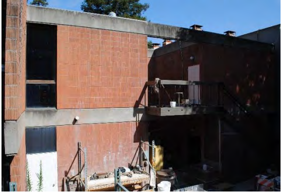
Figure 108. Ceramic Arts Center, portion of east façade with concrete balcony and stair, looking northwest.
