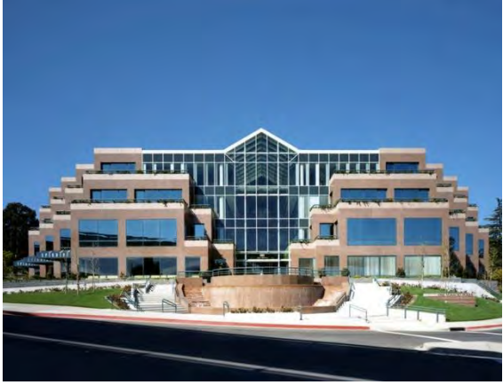
Figure 240. One Ygnacio Plaza, Walnut Creek. Source: Swatt|Miers Architects,
