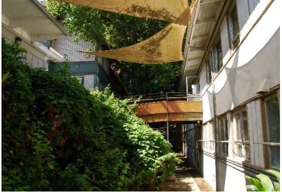
Figure 50. Bridge to the primary entrance of Irwin Student Center on the second floor, looking south.
