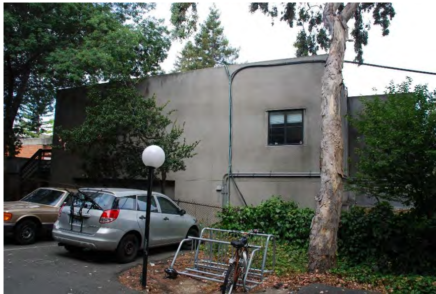
Figure 136. Partial view of the east façade of the Oliver & Ralls Building, facing west.
