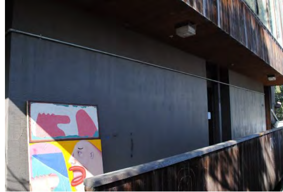
Figure 76. Martinez Hall, north façade second story, looking west.
