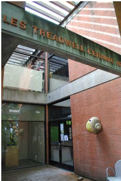
Figure 101. Recessed primary entrance to the Ceramic Arts Center, looking southeast.
