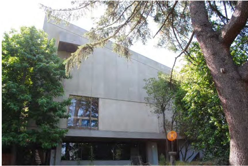
Figure 88. Founders Hall, west façade, facing southeast.
