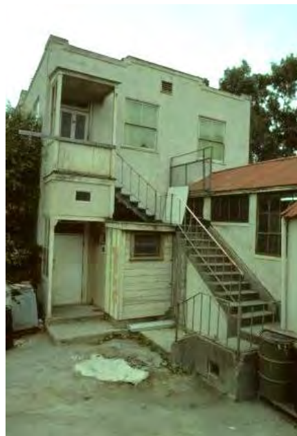
Figure 49. South façade of B Building , showing additions that were removed in renovation, no date, before 1975. Source: CCA Libraries Special Collections.
