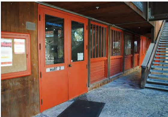
Figure 66. Martinez Hall, primary façade first story detail, facing southeast.
