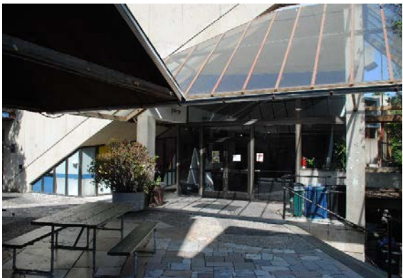
Figure 18. Recessed entry of Founders Hall, covered by a projecting glass canopy which meets the wood canopy of Martinez Hall, looking west.
