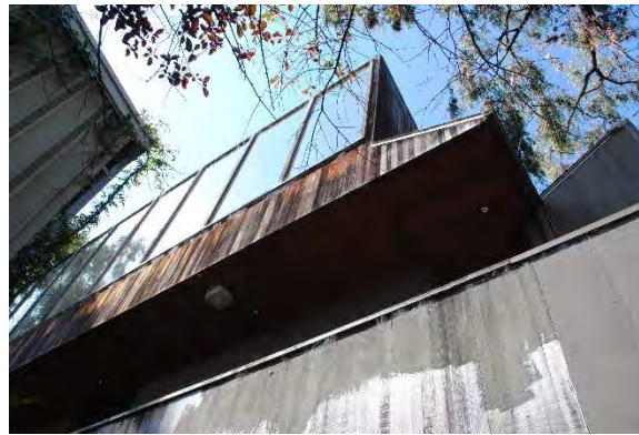
Figure 77. Clerestory windows of the sawtooth roof at the north façade, looking southeast.
