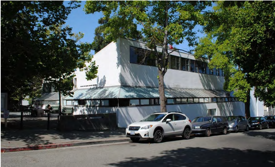
Figure 114. Shaklee Building, oblique view of primary (east) and north facades, looking southwest. North shed roof volume is visible.
