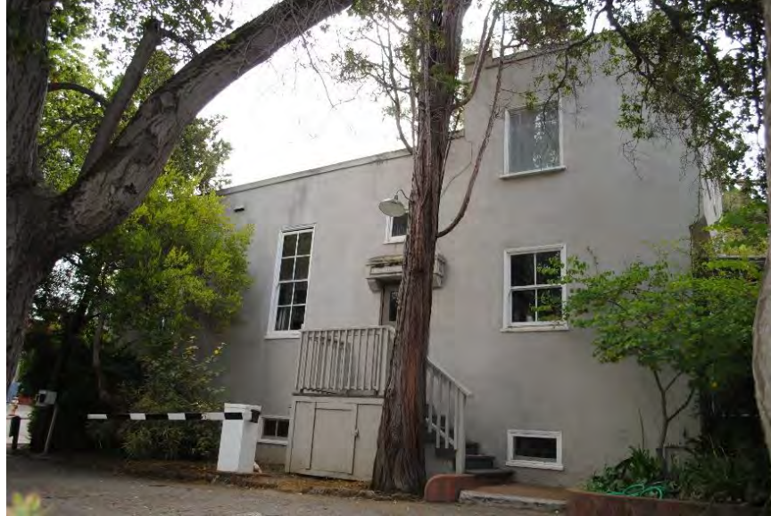
Figure 39. Facilities Building, west façade, facing east.
