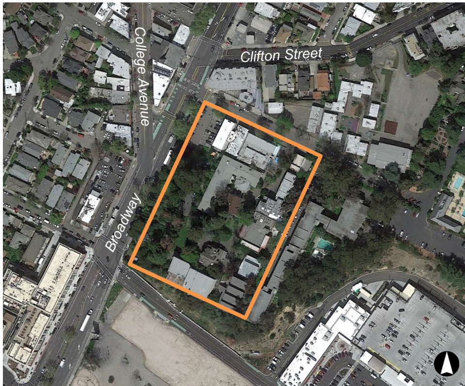
Figure 1. Aerial view of the California College of Art campus in Oakland, outlined in orange. Source: Google Earth Pro, 2019. Edited by Page & Turnbull.
