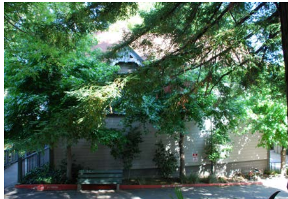
Figure 11. Carriage House, partial view of east façade, facing west.
