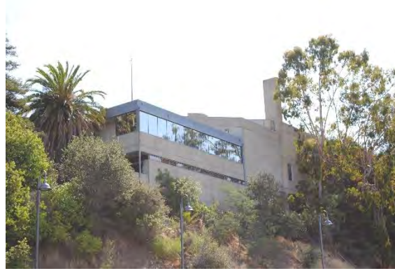
Figure 90. Founders Hall south façade, including 1978 addition, facing northeast.
