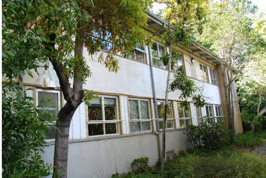
Figure 53. Irwin Student Center, west façade, partial view facing southeast.
