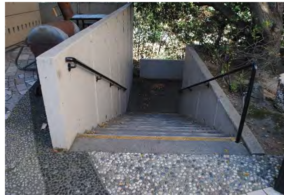
Figure 83. Concrete stairs at the southeast corner of Founders Hall, accessing the south side of the building.
