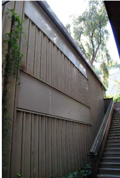
Figure 96. South façade of Martinez Hall Annex, looking east.
