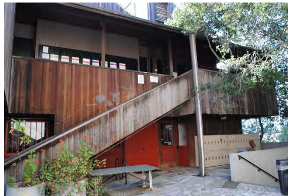
Figure 67. Martinez Hall, primary façade detail, south portion of the first and second stories, facing southeast.
