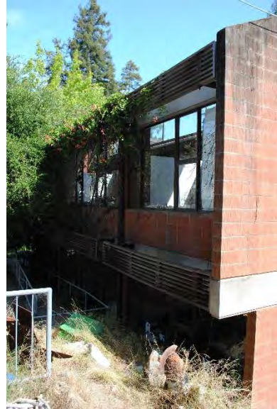
Figure 105. Projecting second story of the south façade, including belt course, wood trellis, and shed roof form, looking northwest.
