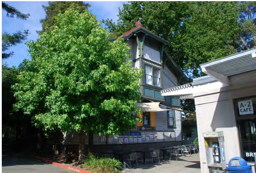
Figure 20. Carriage House, north façade, facing southwest.
