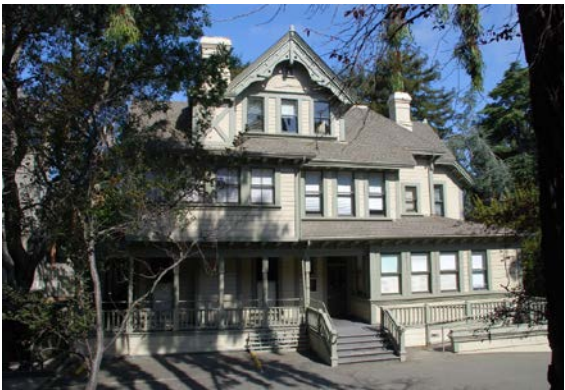
Figure 6. Macky Hall, east (rear) façade, facing west.
