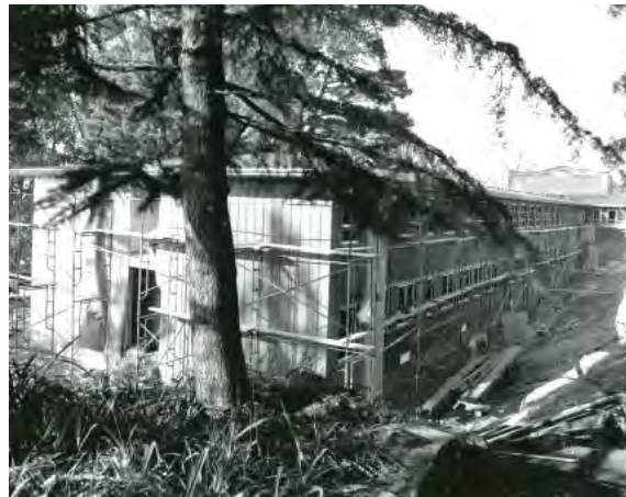
Figure 61. Irwin Hall under construction, 1958. Source: CCA Libraries Special Collections
