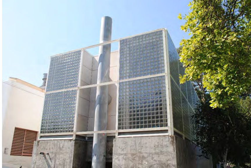
Figure 140. North façade of the Barclay Simpson Sculpture Studio, looking south.
