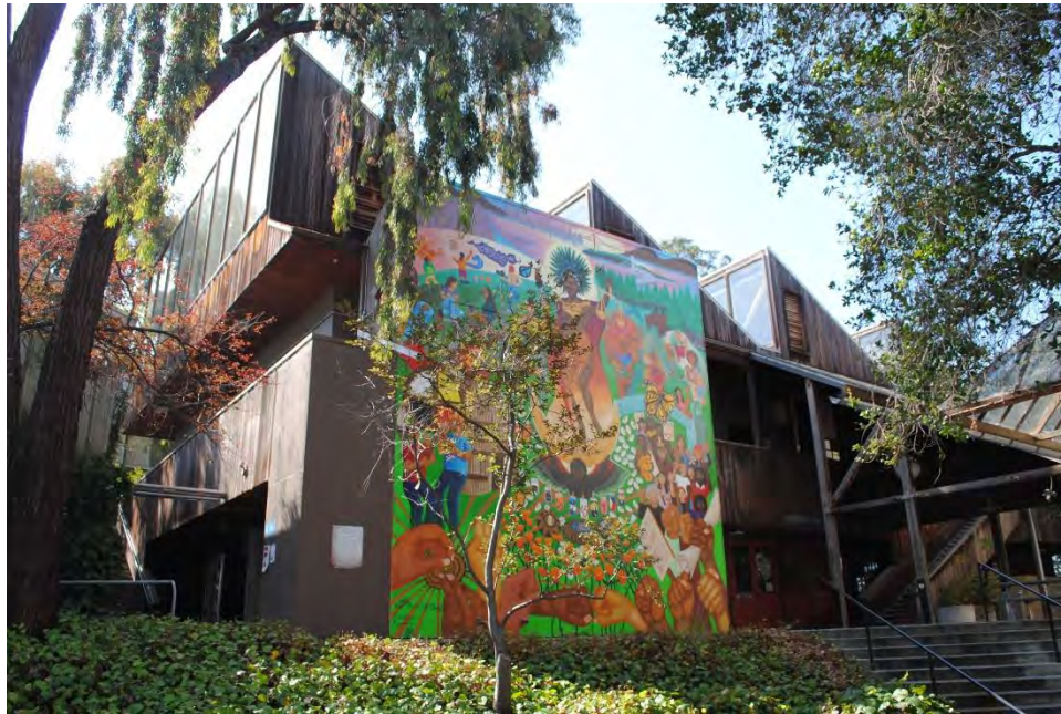
Figure 63. Martinez Hall, west (primary) façade and partial view of north façade, facing southeast.
