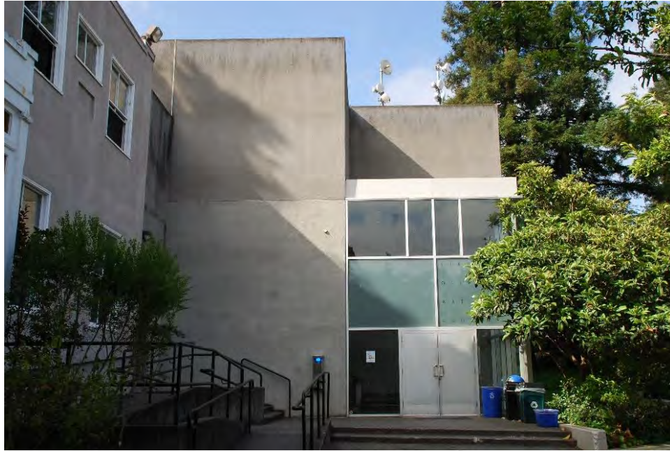
Figure 131. Primary (north) façade of the Oliver & Ralls Building, looking south.
