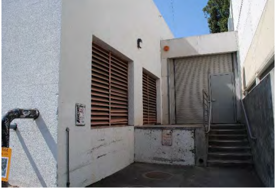
Figure 143. Metal roll-up door accessed via concrete steps on the north side of the hyphen between Barclay Simpson Sculpture Studio (right) and the Shaklee Building (left).
