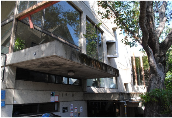
Figure 16. Founders Hall, north façade, facing southwest.
