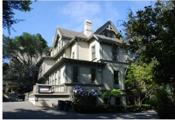
Figure 5. Macky Hall, north façade, partial view, facing southwest.
