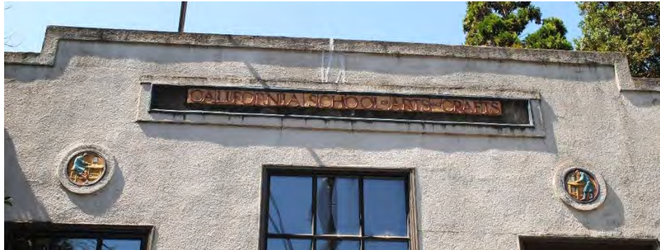
Figure 38. Facilities Building, primary (north) façade, detail, facing south.
