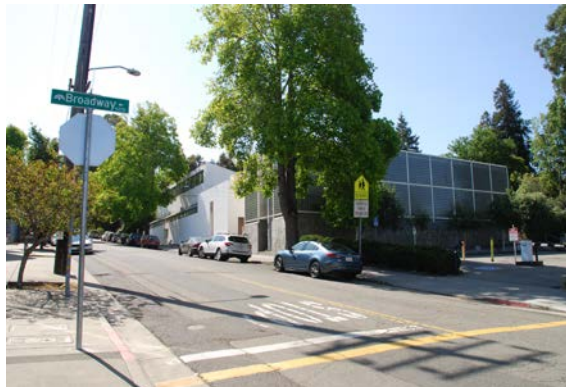
Figure 27. View southeast toward north and west façades.
