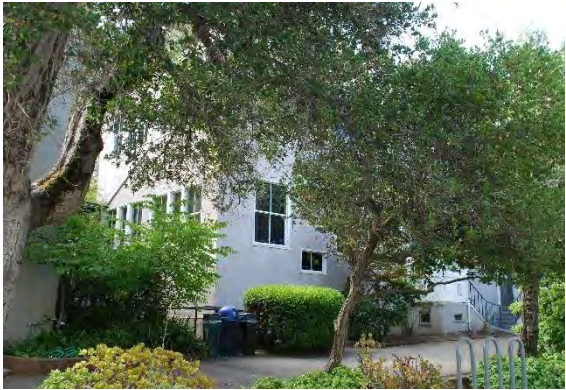
Figure 45. The B Building north and west façades, partial view, facing southeast.
