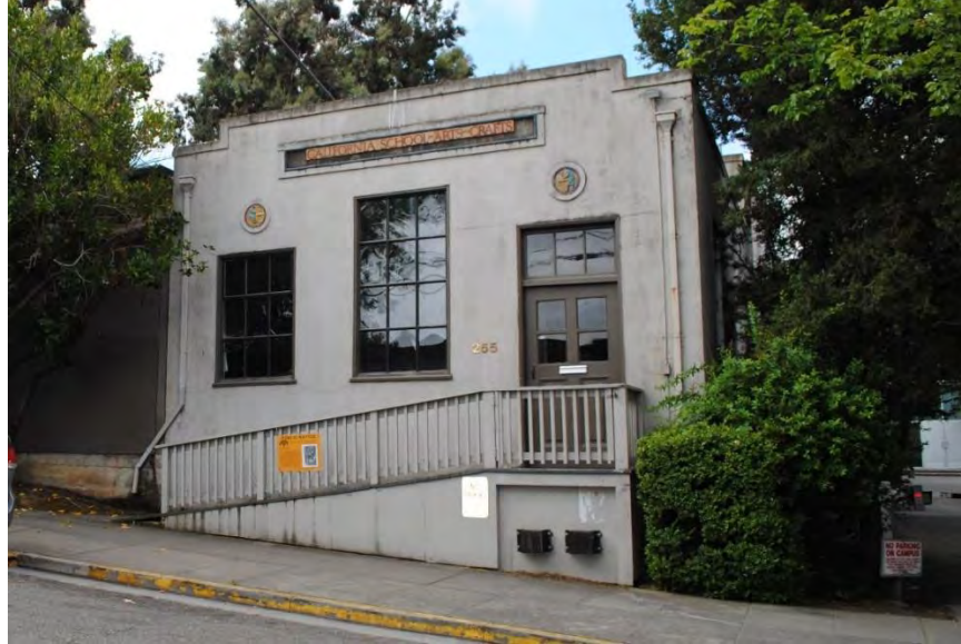
Figure 37. Facilities Building, primary (north) façade, facing south.
