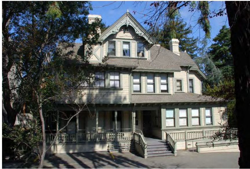
Figure 12. Macky Hall, east (rear) façade, facing west.
