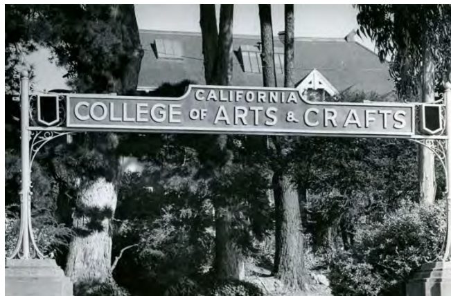
Figure 35. View of the vehicle entrance sign, with neon lettering removed, 1973. Source: CCA Libraries Special Collections.
