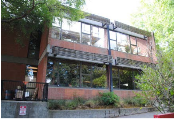
Figure 20. Ceramic Arts Center, south portion of primary (west) façade, facing east.
