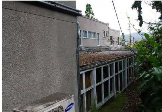
Figure 46: The B Building east façade, facing north.
