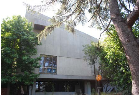
Figure 17. Founders Hall, west façade, facing southeast.
