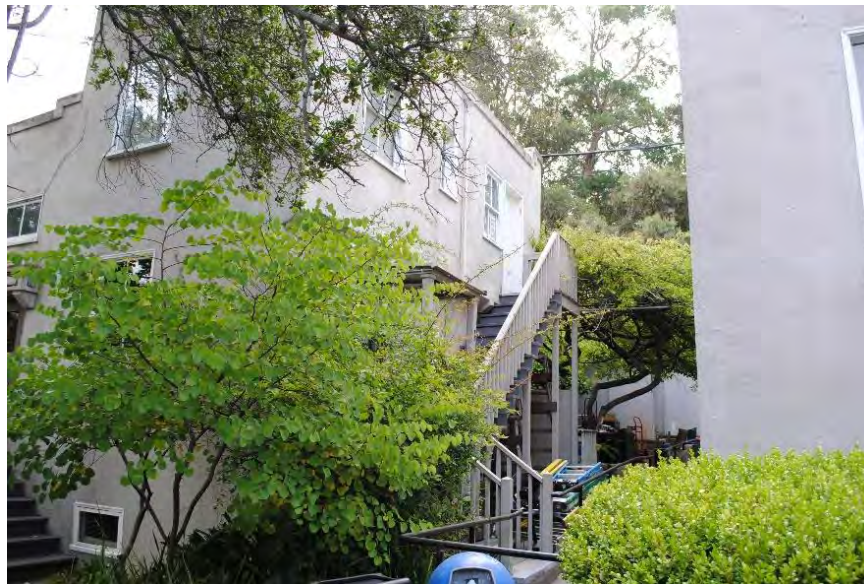
Figure 40. Facilities Building, south façade, partial view, facing northeast.
