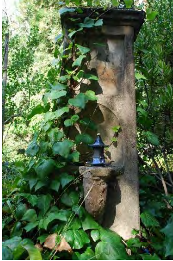
Figure 162. Concrete water fountain south of the Carriage House (2019).
