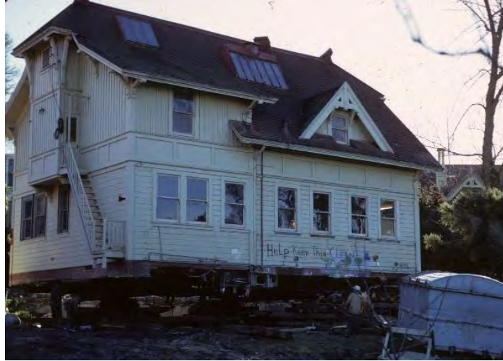
Figure 24. West and north facades of the Carriage House raised up on temporary foundation for relocation, 1973. Source: CCA Libraries Special Collections.
