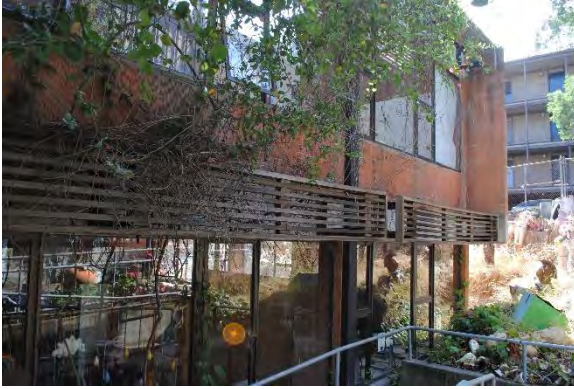
Figure 104. Ceramic Arts Center, portion of south façade with trellis detail, looking northeast.
