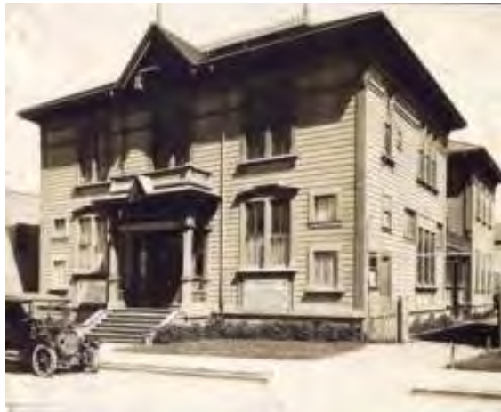
Figure 190. 2119 Allston Way, Berkeley, home of the California School of Arts and Crafts from 1910 to 1926, n.d. Source: CCA Library Special Collections.
