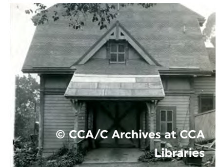
Figure 2.7: Carriage House original opening on east facade
