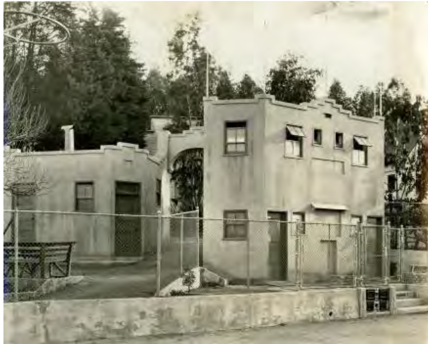
Figure 201. Shower House and tool house, constructed between 1925 and 1930 (not extant), photograph dated 1930. Source: CCA Libraries Special Collections.
