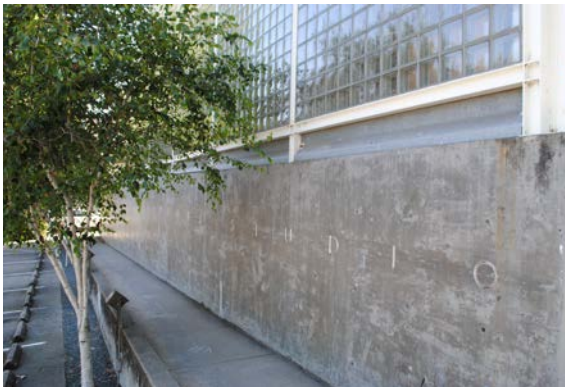
Figure 26. Detail of inscribed, polished concrete base, west façade, looking northeast.
