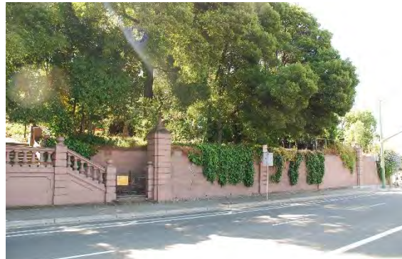
Figure 28. Broadway Wall, southernmost three piers, facing southeast.
