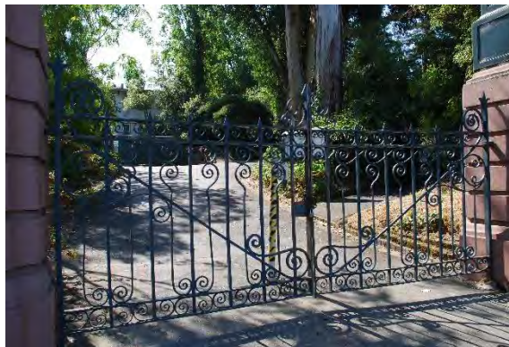
Figure 32. Original two-leaf wrought iron gates at the carriage entrance of the Broadway Wall, looking east.
