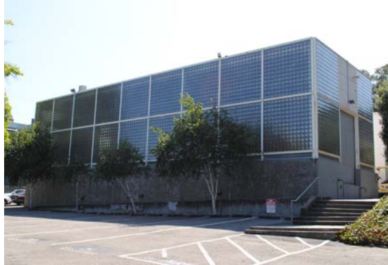
Figure 25. West and south façades of the Barclay Simpson Sculpture Studio, looking northeast
