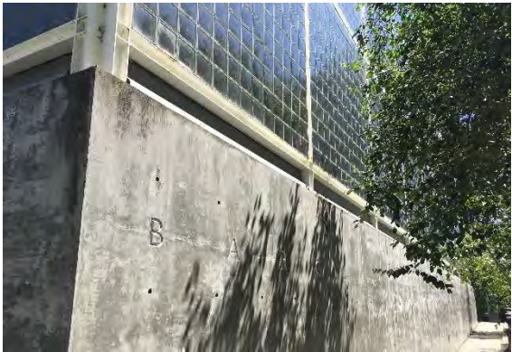
Figure 138. Polished concrete base with exposed concrete formwork tie-holes and incised, silver-painted lettering, looking southeast.
