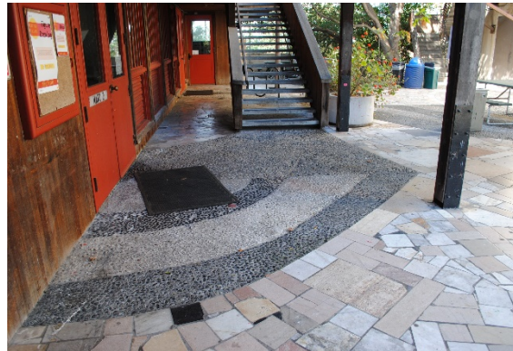
Figure 15. Irregular, polychromatic flagstone and pebble patio between Martinez Hall and Founders Hall, looking south
