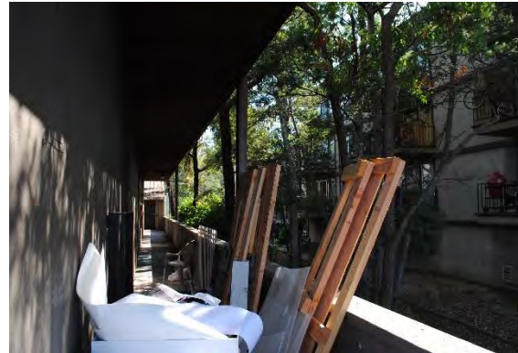
Figure 74. Martinez Hall, east façade, second story, looking north.
