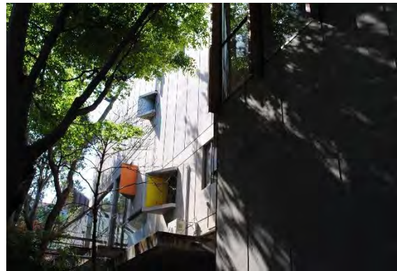
Figure 85. Founders Hall, north façade, second story detail, facing south.
