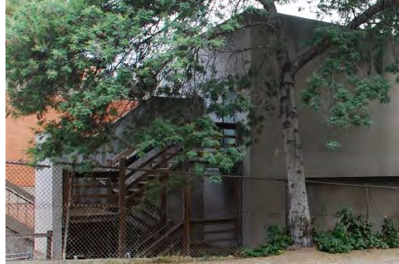
Figure 135. Exterior stair tower at the southeast corner of the Oliver & Ralls Building, accessing doors on the south façade, looking northwest.
