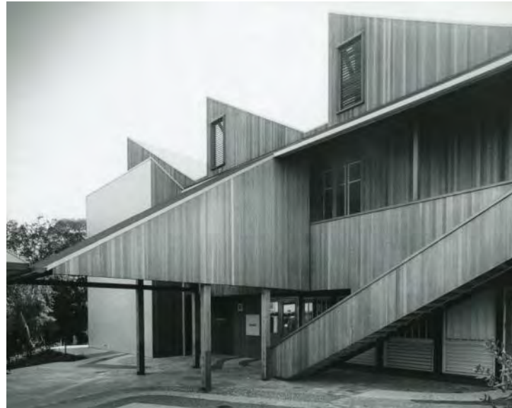
Figure 79. Martinez Hall completed, 1968, blank mural wall visible at left. Source: CCA Libraries Special Collections.
