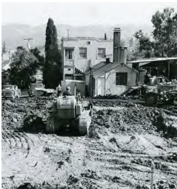
Figure 48. South façade of B Building during site clearing and construction of the Noni Eccles Treadwell Ceramic Arts Center, 1973. Source: CCA Libraries Special Collections.
