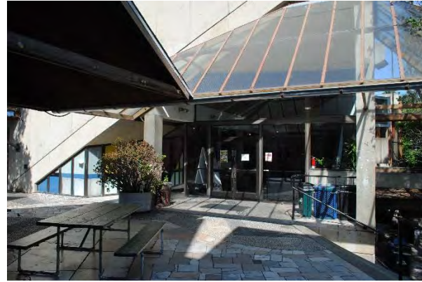
Figure 81. Recessed entry of Founders Hall, covered by a projecting glass canopy which meets the wood canopy of Martinez Hall, looking west.
