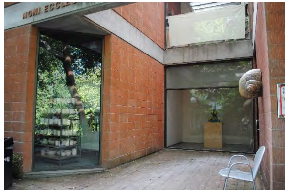
Figure 102. Chamfered corner of the first story of the north volume of the Ceramic Arts Center, featuring a fully glazed window wall with views to the kiln area, looking northeast.
