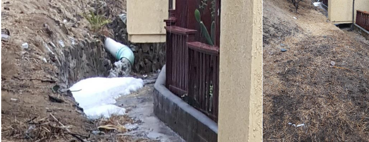
Photo Figure 9: Characteristic conditions of stormwater inputs to the channel system, north of the proposed project area, taken during a rain event.
