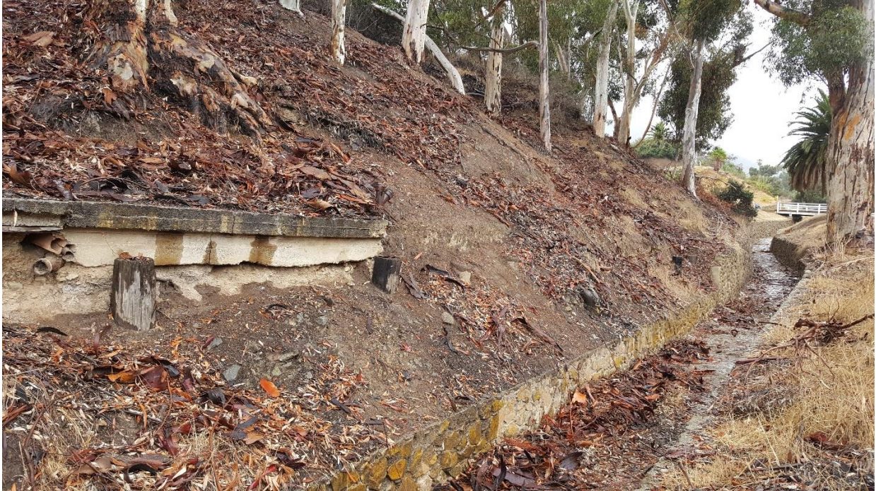
Photo Figure 7: Characteristic conditions of Avalon Creek, facing upstream towards golf course.
