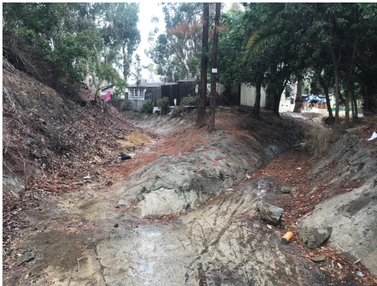
Photo Figure 14: Characteristic conditions at the confluence of Avalon Creek and the stormwater channel that is parallel to Fremont Street. Both features have constructed bottoms.
