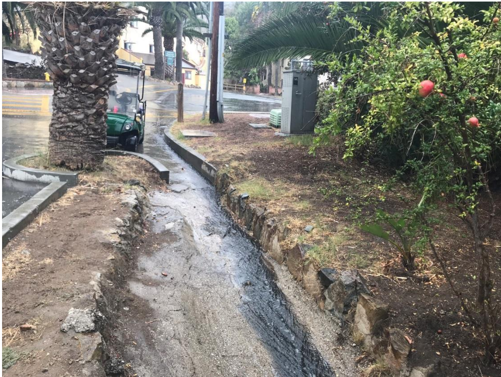
Photo Figure 10: Characteristic conditions of stormwater inputs to the channel system, in the proposed project area, taken during a rain event.
