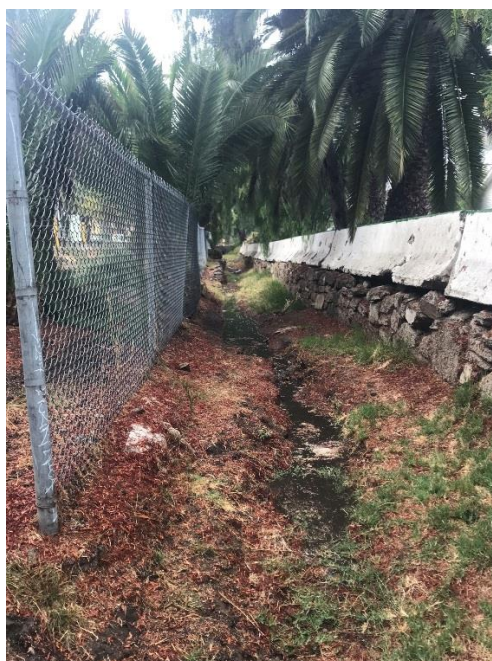
Photo Figure 12: Characteristic conditions of stormwater channel system, in the proposed project area, taken during a rain event below the confluence of the inputs from areas shown in Photo Figures 11, 10, and 9.
